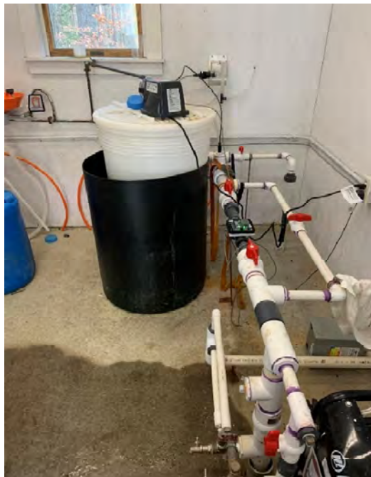
Figure 2-8 Thetford Co-Op Chlorination Assembly
