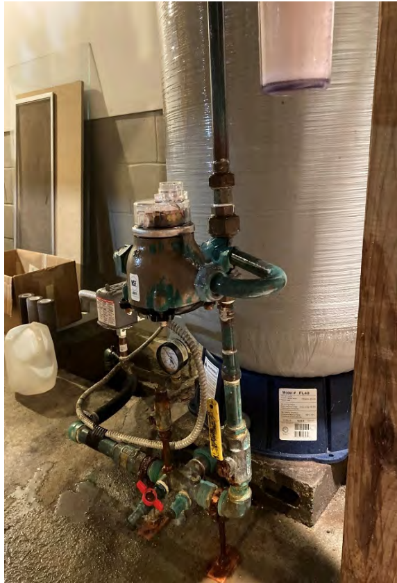
Figure 2-3 North Village Water Company Hydro-pneumatic Tank and Meter
