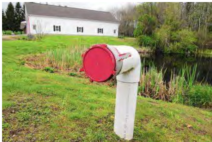
Figure 2-13 Dry Hydrant and Fire Pond
