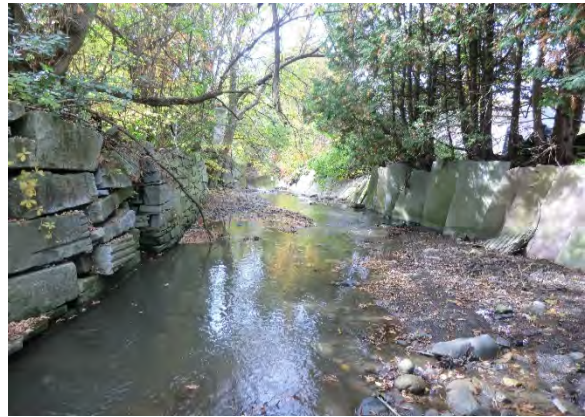
Figure 13: Failing walls typical in Barre City
