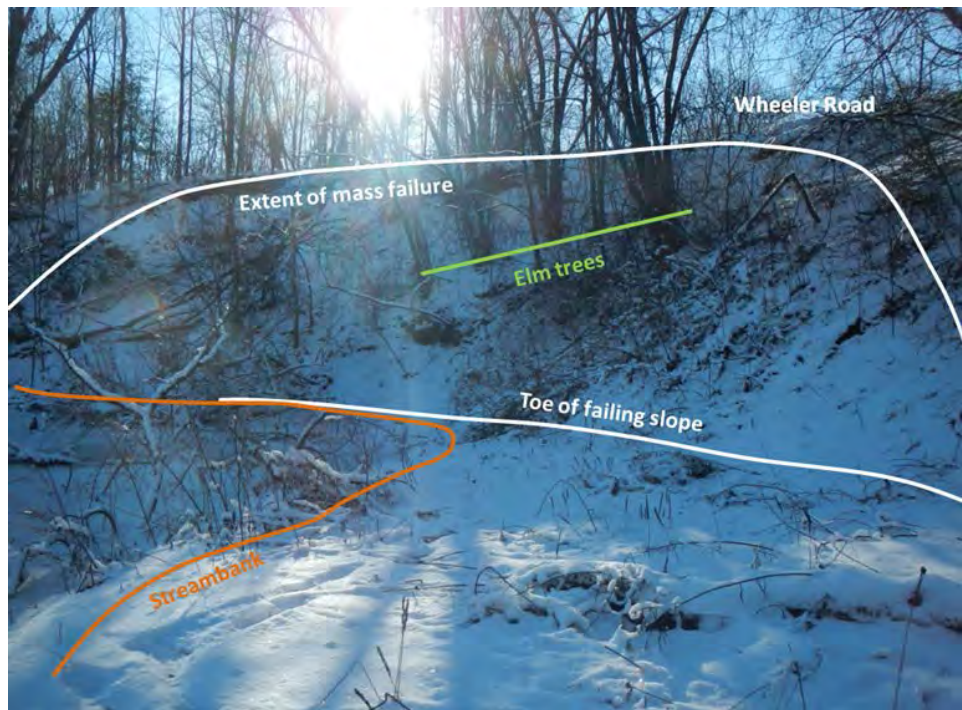
Figure 10: Bank failure site from the upstream right bank floodplain
