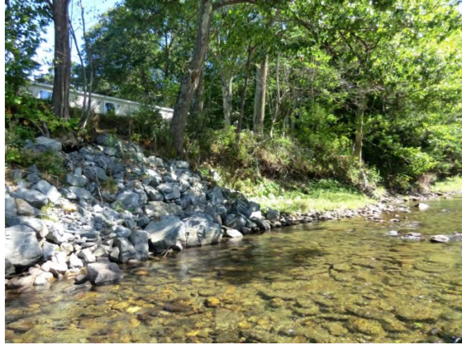
Figure 4: Rock riprap placed at the Riverside Mobile Home Park following Tropical Storm Irene to reinforce the bank
