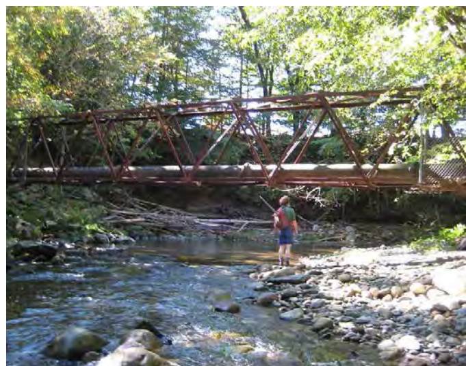
Figure 11: Sewer line crossing Whetstone Brook, 2008 before it washed out in Tropical Storm Irene.
