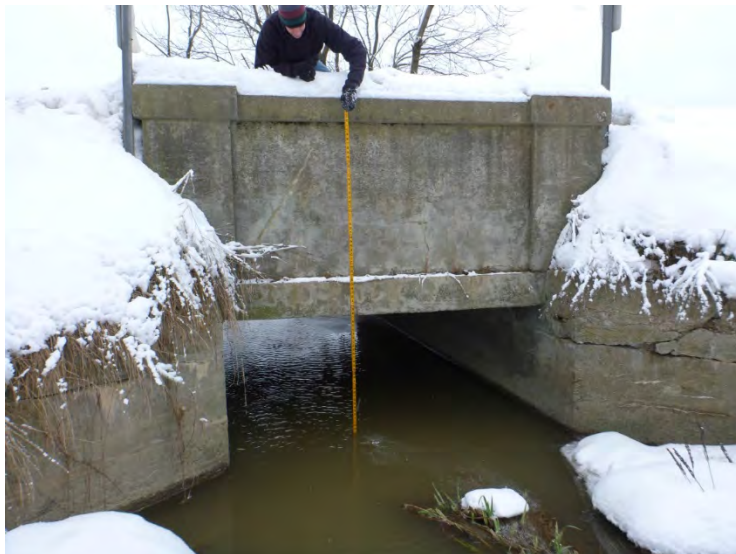
Figure 4.3: Fieldwork Makes the Difference – Measuring Undersized Culvert
