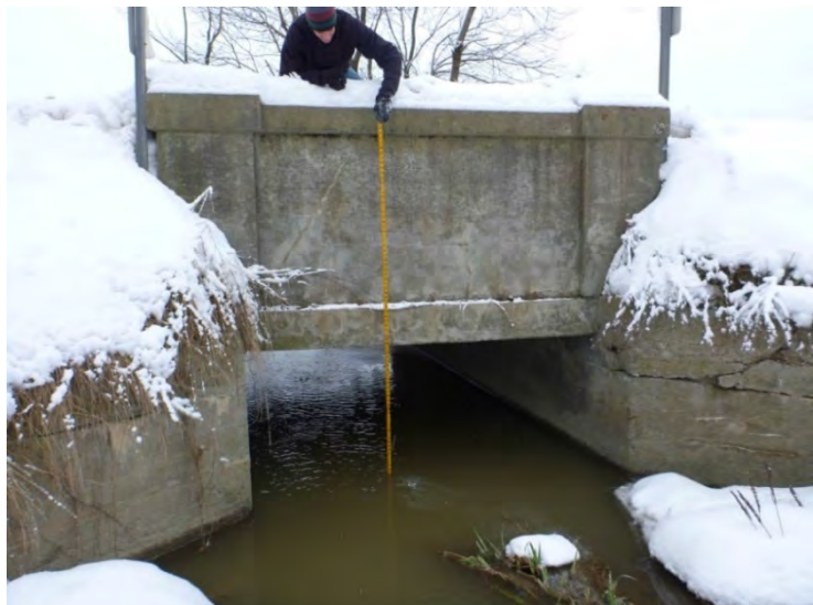
Figure 10: Undersized culvert on a tributary of the Missisquoi River at Hayes Farm Road (Source: FEA, 2014)
