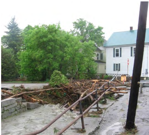
Figure 12: Debris at bridges compounded the May 2011 Flood
