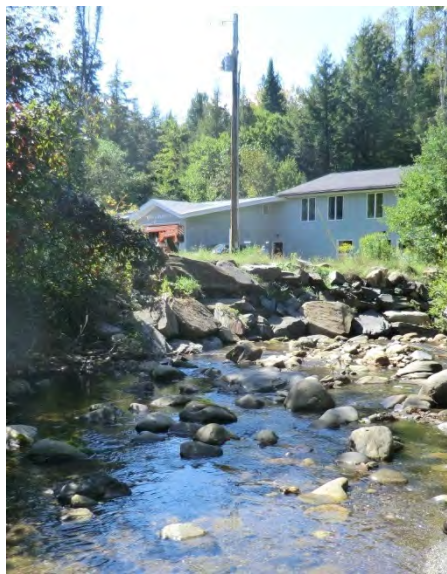
Figure 10: The Bates and Murray building in Barre Town was flooded in May 2011
