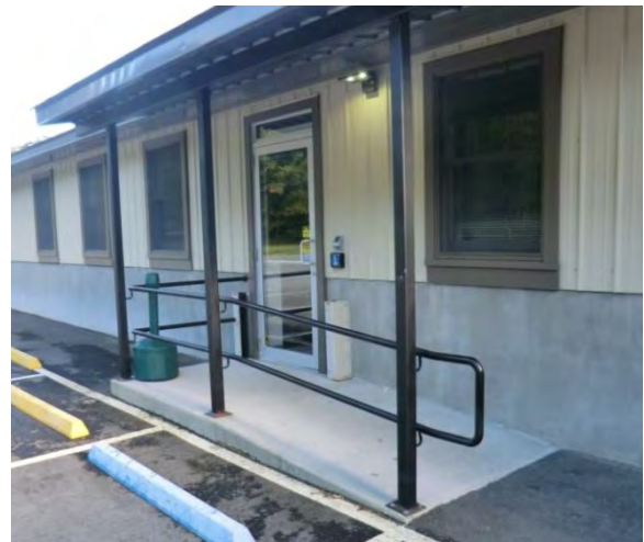
Figure 10: Dead River Propane offices have sealed walls and door dams to keep floodwaters out
