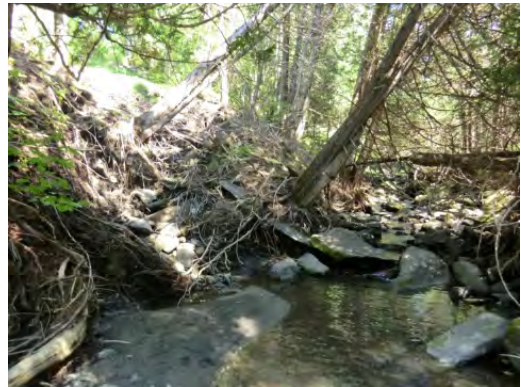
Figure 3: Slope failures are common on upper Gunners Brook in Barre Town
