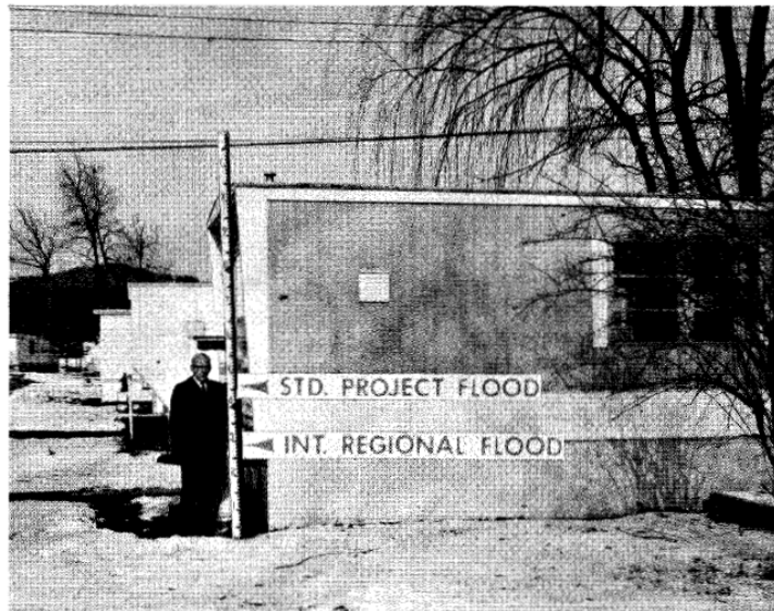
Flood Heights, mobile home in Glen Trailer Park, across Whetstone Brook from photograph above.
