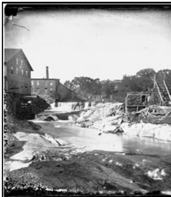
Figure 5: Damage to downtown, 1869 Freshet (Brattleboro Historical Society)
