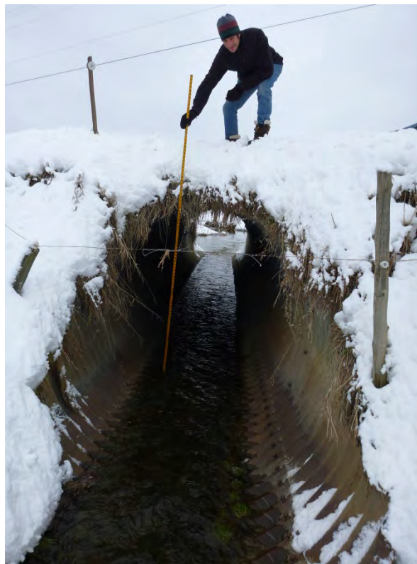
Figure 15: Undersized culvert on a tributary of the Missisquoi River at Davis Road (Source: FEA, 2014)
