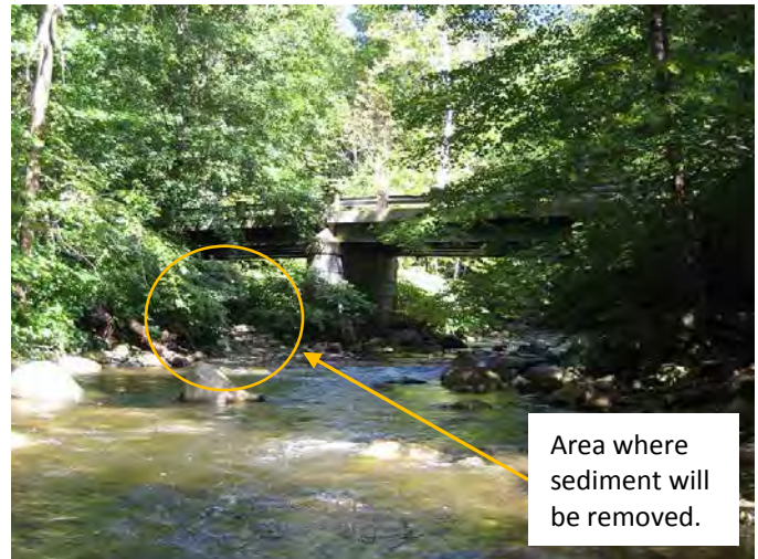
Figure 10: Easterly Williams Street Bridge 2008
