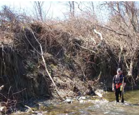
Mass failure before restoration
