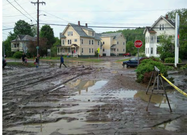
Figure 11: Road damage and sediment deposits following the May 2011 Flood
