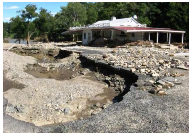
Destroyed White Cottage Snack Bar building
