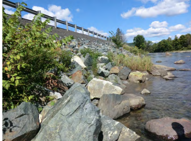
Figure 12: Poor rock riprap placement that needs to be reinforced to improve the stability of US Route 4
