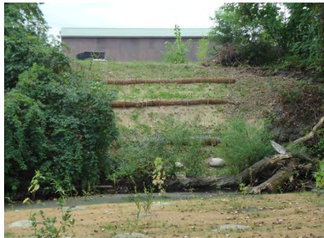
Mass failure after restoration
