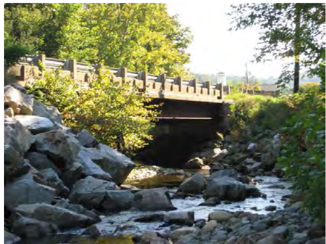
Figure 9: Misaligned VT Route 9 Bridge (2008) before Tropical Storm Irene
