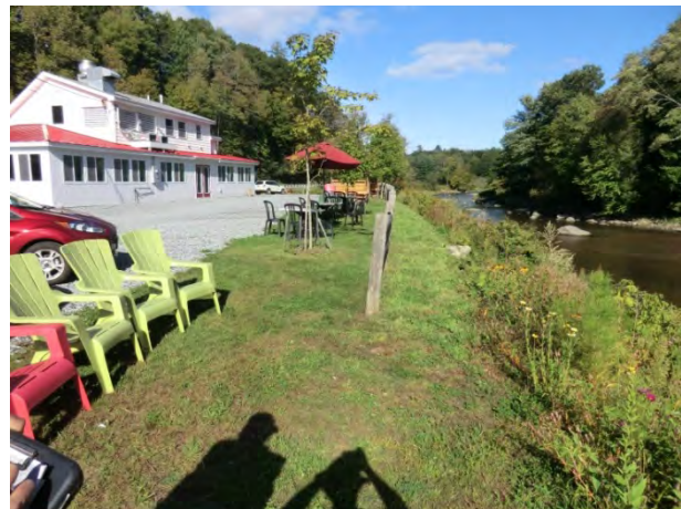
Figure 11: The White Cottage Snack Bar was rebuilt farther away from the river
