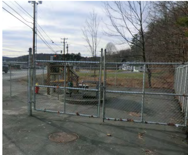
Figure 13: Municipal sewer pump station in West Woodstock needs to be retrofitted to prevent inundation by floodwaters
