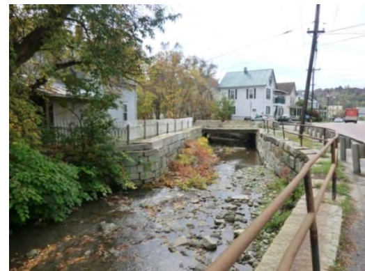
Figure 7: Retaining walls and typical small bridge opening in the downstream portion of Barre City
