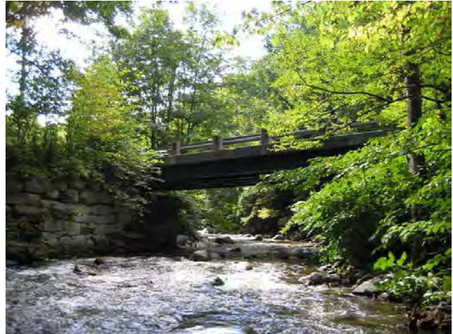
Figure 8: View of Eastern Williams Street Bridge from upstream. Left abutment eroded during Irene, sediment buildup shown right.
