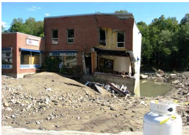
Destroyed Dead River Propane Office building
