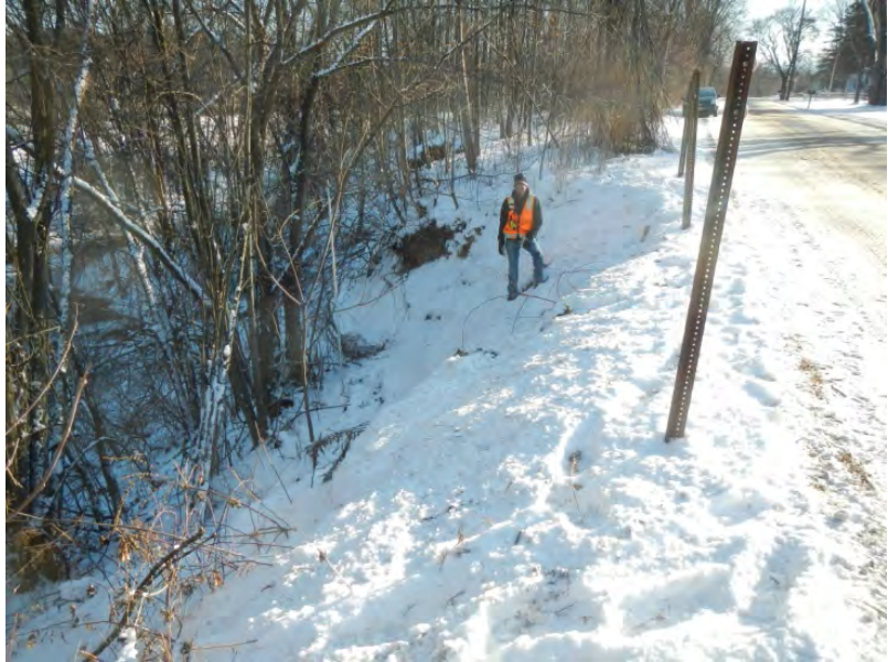
Figure 9: Top of bank failure along Wheeler Road
