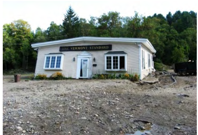
Destroyed Vermont Standard building
