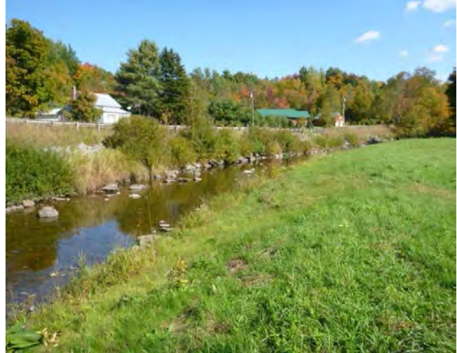
Figure 7: Tyler branch Road is threatened by erosion from the river and rock armoring is common along the embankment. (Source: FEA, 2014)
