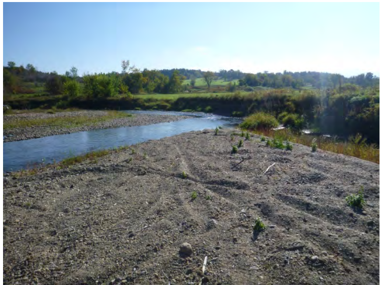
Figure 6: Deposited sediment and eroding banks upstream of Tyler Branch Road Bridge (Source: FEA, 2014)
