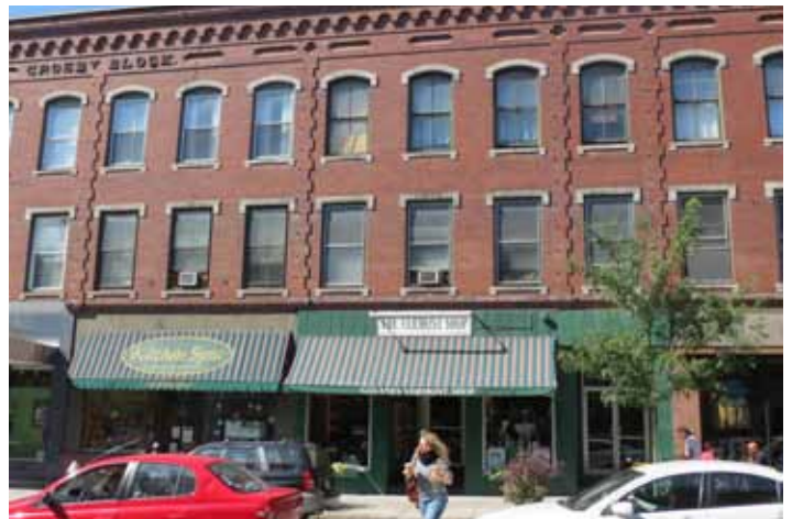
Stone Heads and Sills, Detailed Brick Cornices
