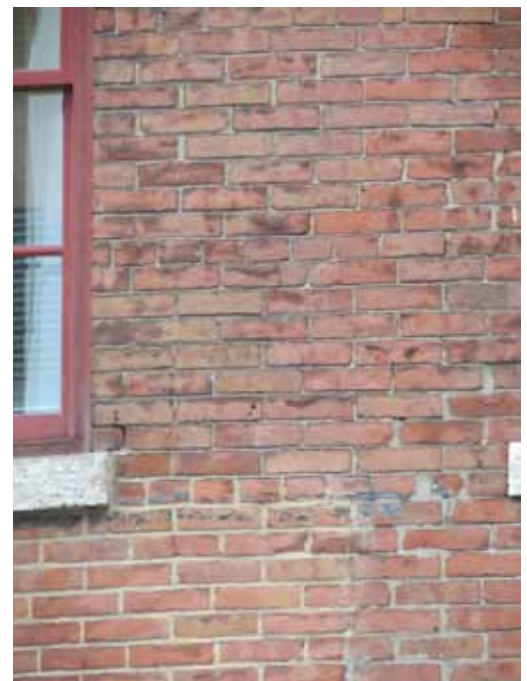
Examples of New Brick and Mortar Joints That Do Not Match Existing
