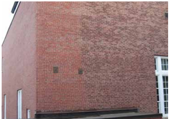
Brick that has Been Cleaned and Brick That Has Not
