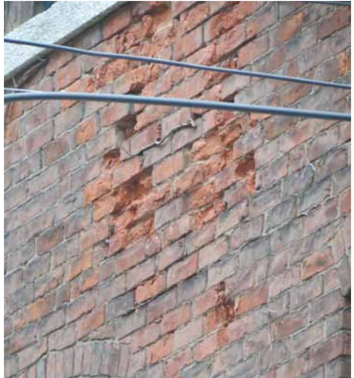
Examples of Spalled Brick
