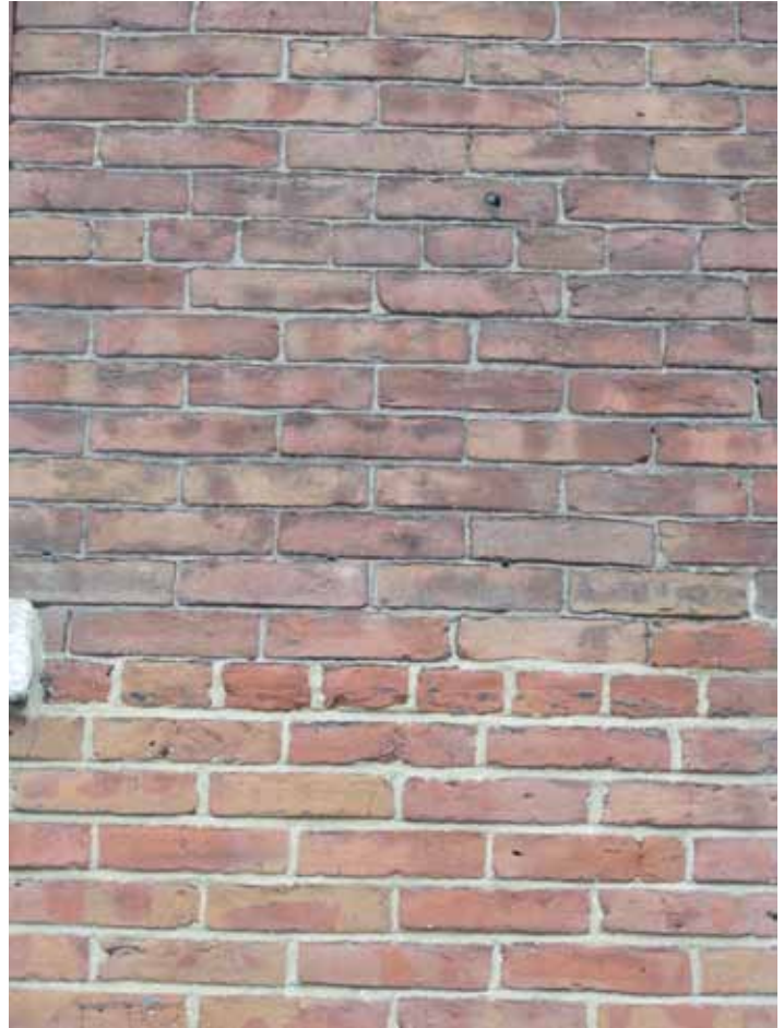
Examples of Poor Repointing Matching existing
