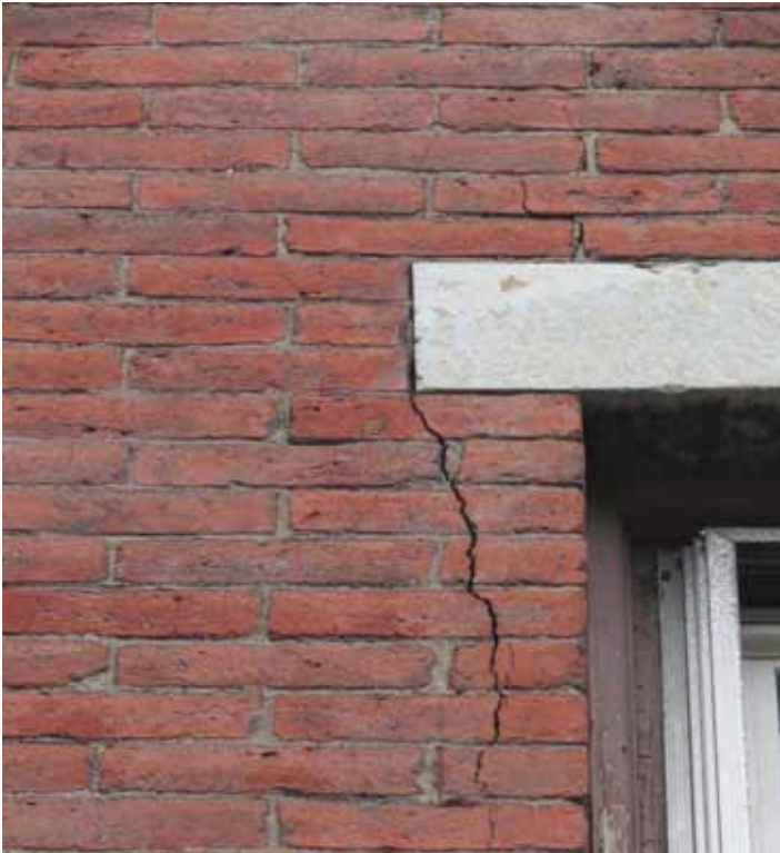
Examples of Split Brick Below Stone Header
