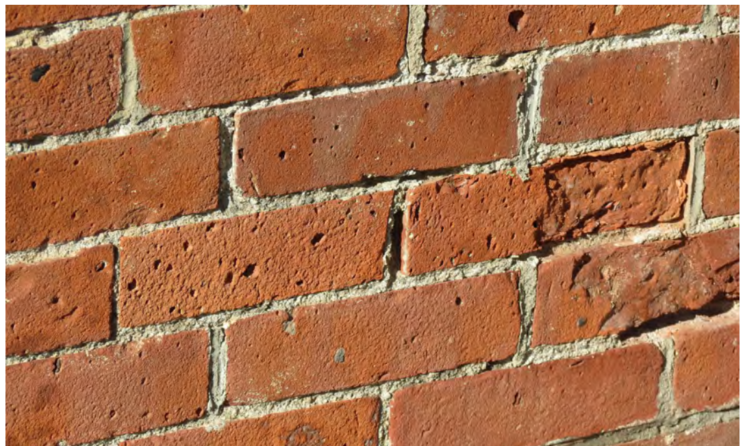
View of existing brick that has been be improperly repointed
