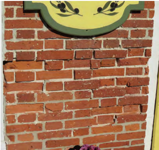
View of sandblasted brick that has spalled
