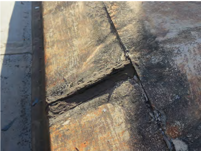
Close Up View of Failed Panel Joints
