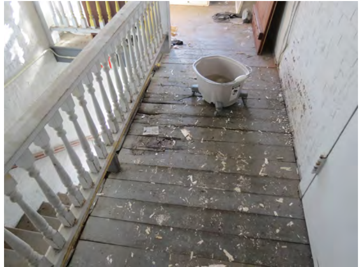
View of water damaged wood flooring
