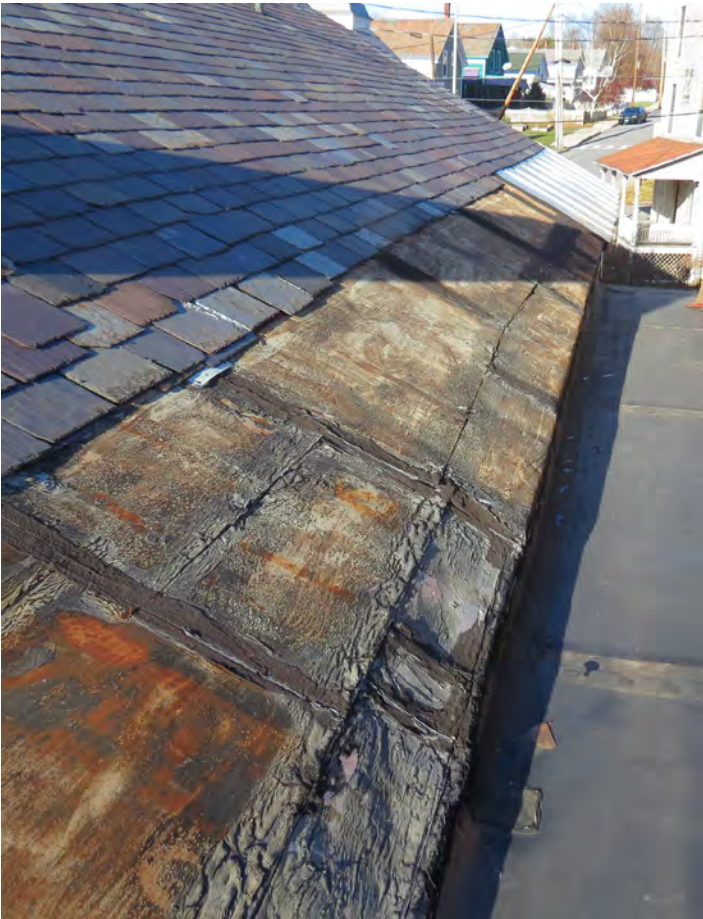
View of Adjacent Owner's Roof with Failed Panel Joints
