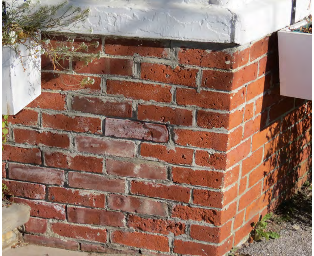
View of existing brick that has been be improperly repointed
