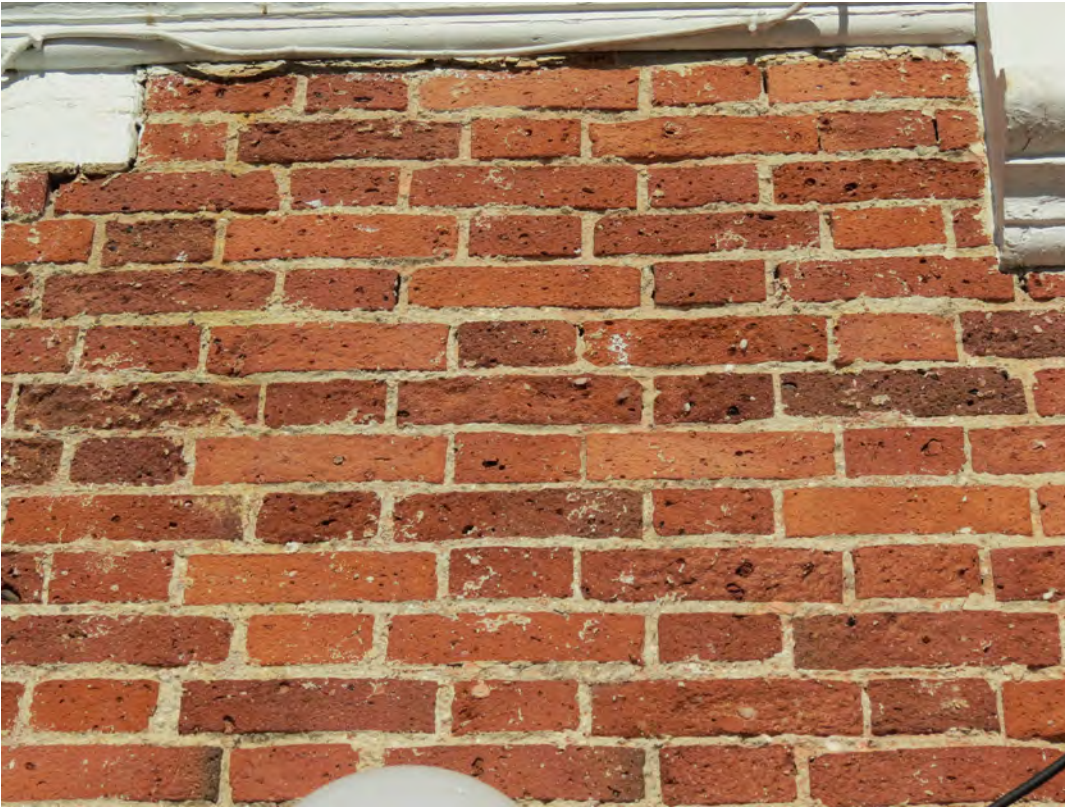
View of existing brick that has been sandblasted
