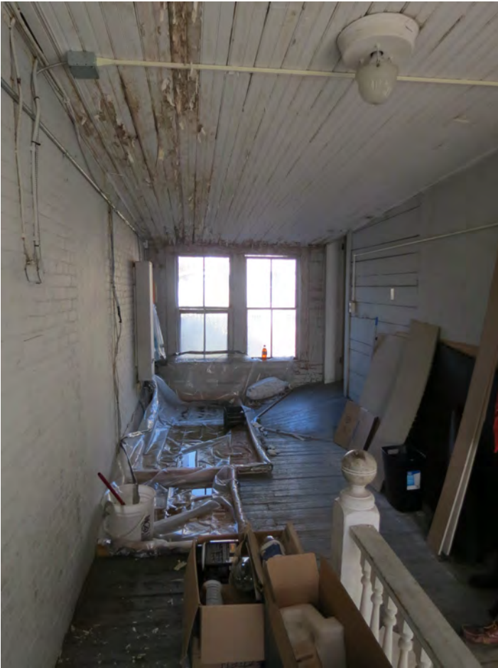
View of shared stairway with leak at ceiling
