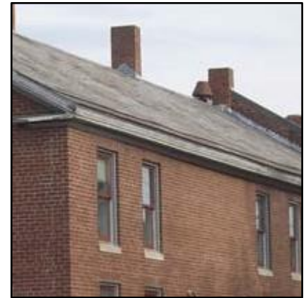
Pitched roof with enclosed eaves
