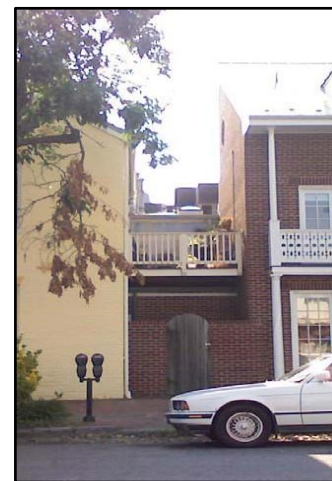
Brick STREET WALL between Townhouses
