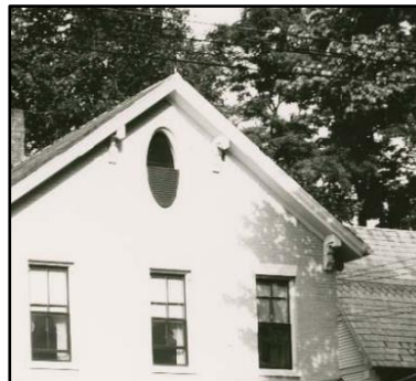
Pitched roof gable end with brackets
