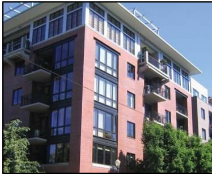
Parapet wall with projecting cornice
