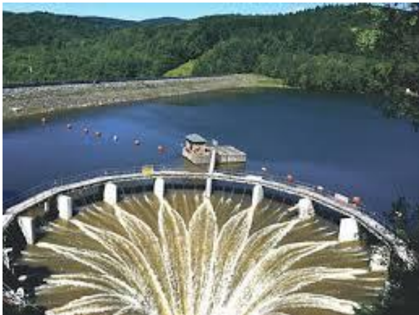
Harriman Power Generation Dam Glory Hole Photo: DVNews.com
