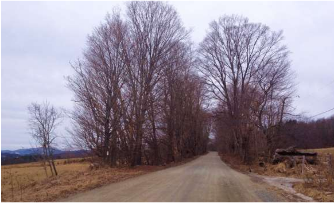
View southwest along Hale Road between Sutor Rd and Valley View
