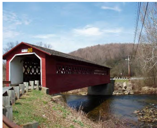
The Walloomsac River at the Henry Covered Bridge.
