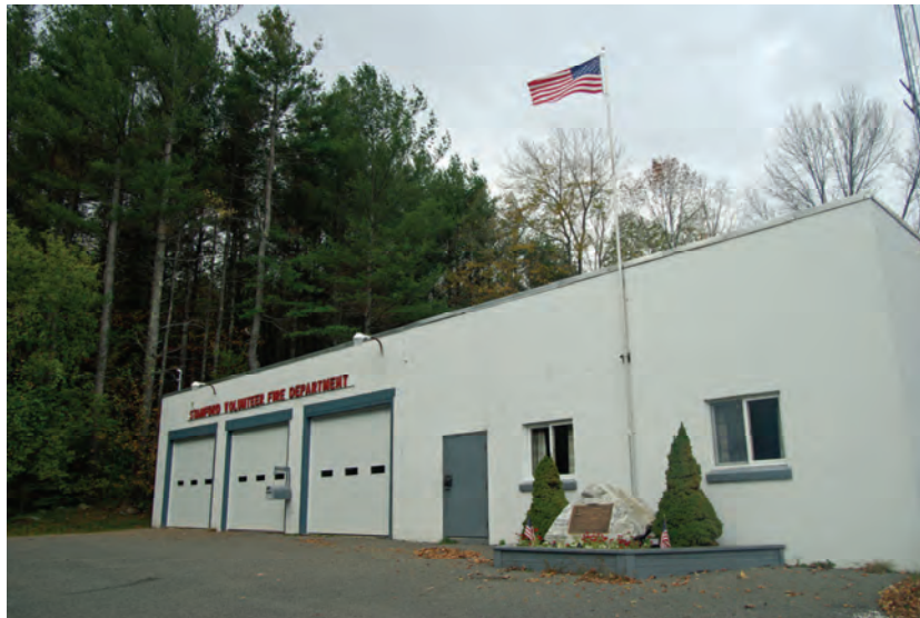
The Stamford Volunteer Fire Department provides a full range of emergency fire, medical, and natural disaster services to the community, operating out of this centrally located facility on Mountain View Lane.
