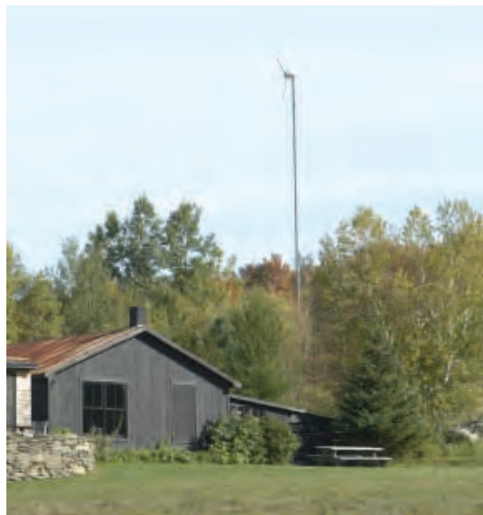
Residential-scale turbines can provide electricity for homes located on windy sites.
