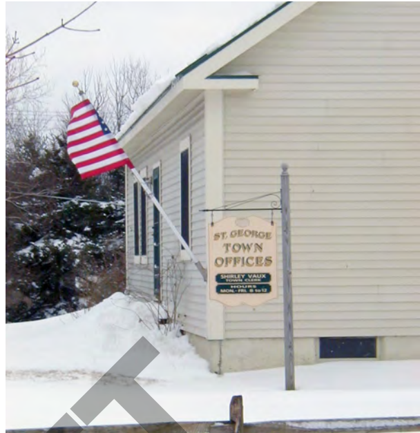
FIGURE 2. ST. GEORGE TOWN OFFICE
