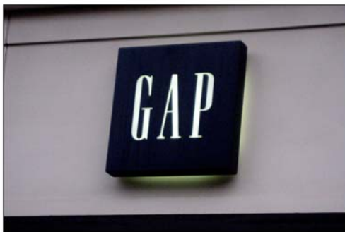
Internal illumination w/ opaque background
