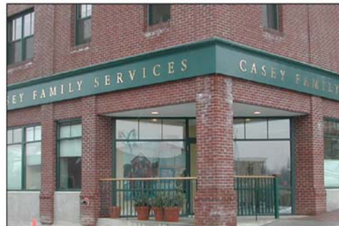
Cut-out lettering and sign band
