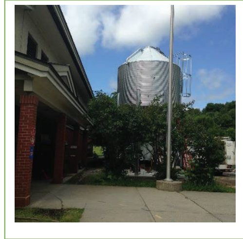
Figure 3: Sharon Elementary School wood pellet hopper (photo credit Sharon Elementary)
