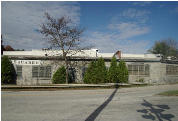
The former Eagle Square tool plant is now occupied by Bernstein Displays.
