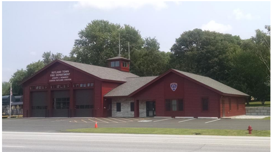
New Center Rutland Fire Station constructed in 2014
