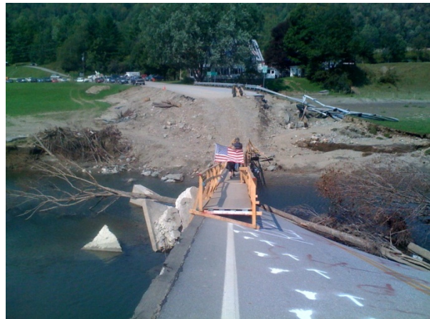
5 - Temporary footbridge over White River (Source: VTrans)
