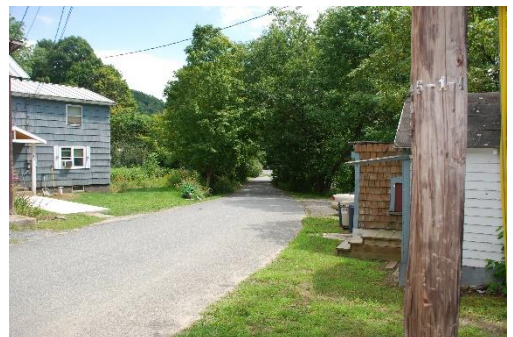
View looking south along Niagara Street before the impacts of Tropical Storm Irene. This section of road today does not connect to Route 106.
