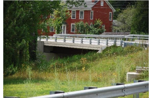
Route 44 near Route 106 and 1815 House at Mill Brook stream crossing.
