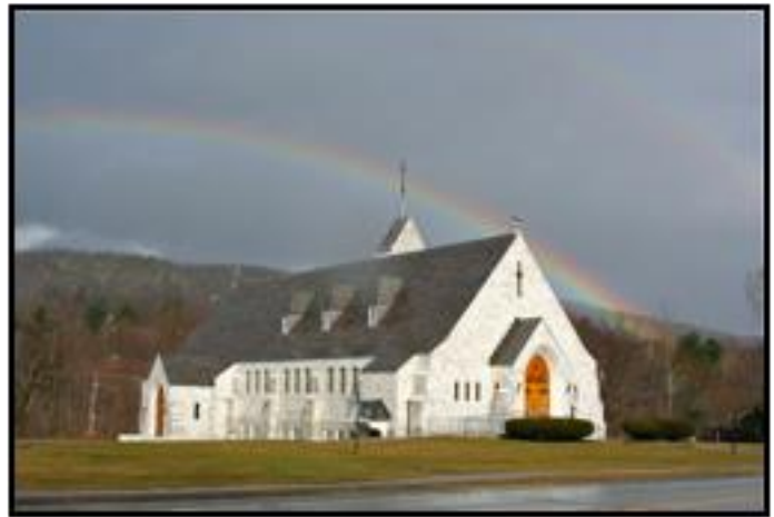
St Dominic's Roman Catholic Church, 1925, Neo-Gothic Revival. Built of local materials, the walls are faced with smooth blocks of marble and the roof is covered with many rows of longwearing slate.
