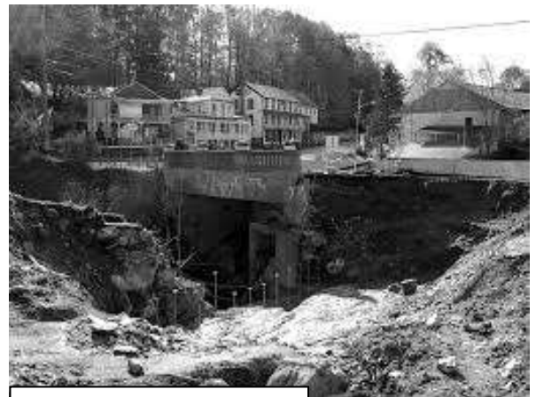
View of Route 30 Bridge from Cemetery Hill Road
