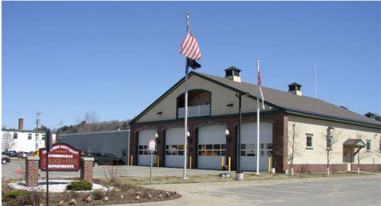
Lyndon Public Safety Facility, Lyndonville
