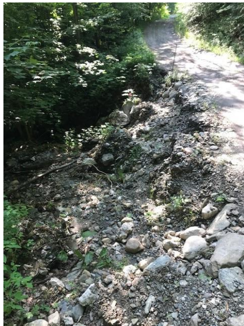
Flood damage to a road. Source: Bob Toppin.
