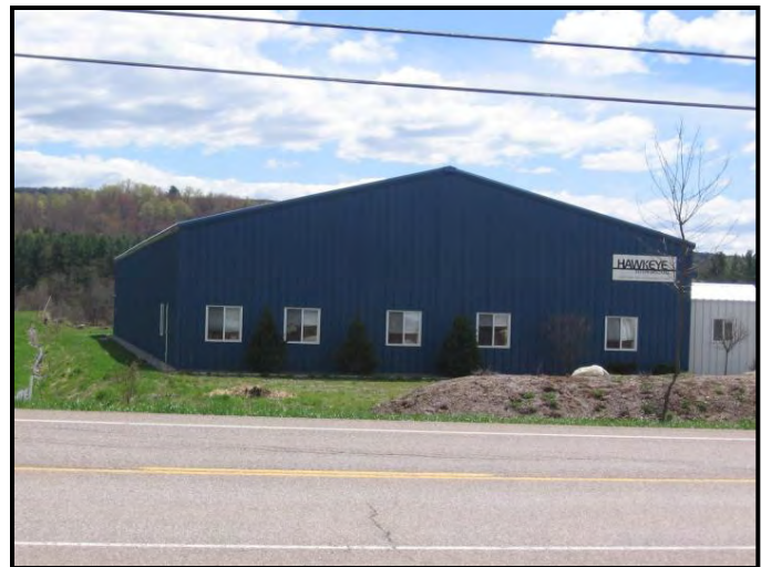
Photo: N. Hyde Park Industrial Park from Route 100
