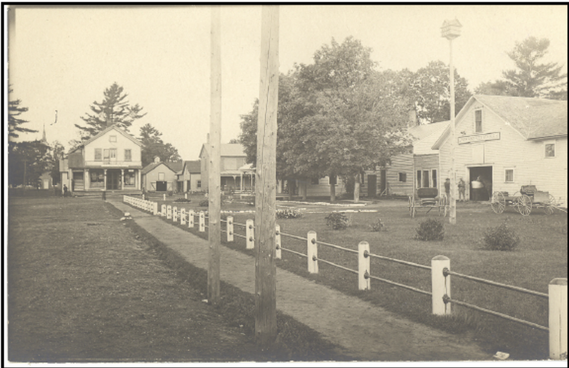
Highgate Center looking west at Desorcie's Store, circa 1900 Photo used with permission from the Highgate Historical Society
