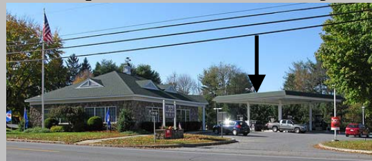
Pumps on side of building
