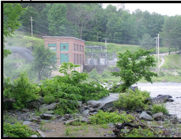
Photo 7 - Fairfax Falls Substation, by Skip Taylor
