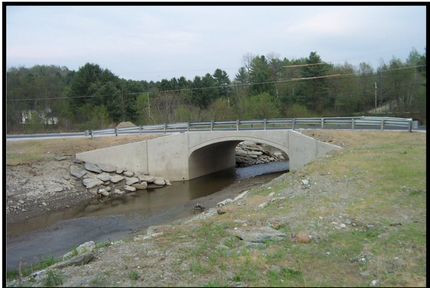
Photo 19 - Improved River Road Bridge, by Henry Raymond
