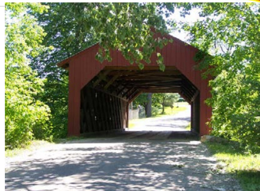
Photo 5 - Maple Street Covered Bridge, by Skip Taylor
