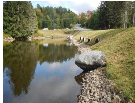
Snow Lake Dam at South Access Road (Credit: WRC)
