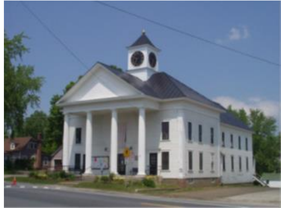
Danville Town Hall and Offices
