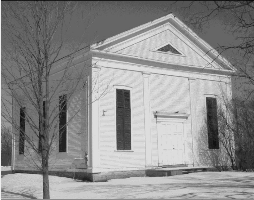
Figure 42: Former Baptist Church in West Cornwall
