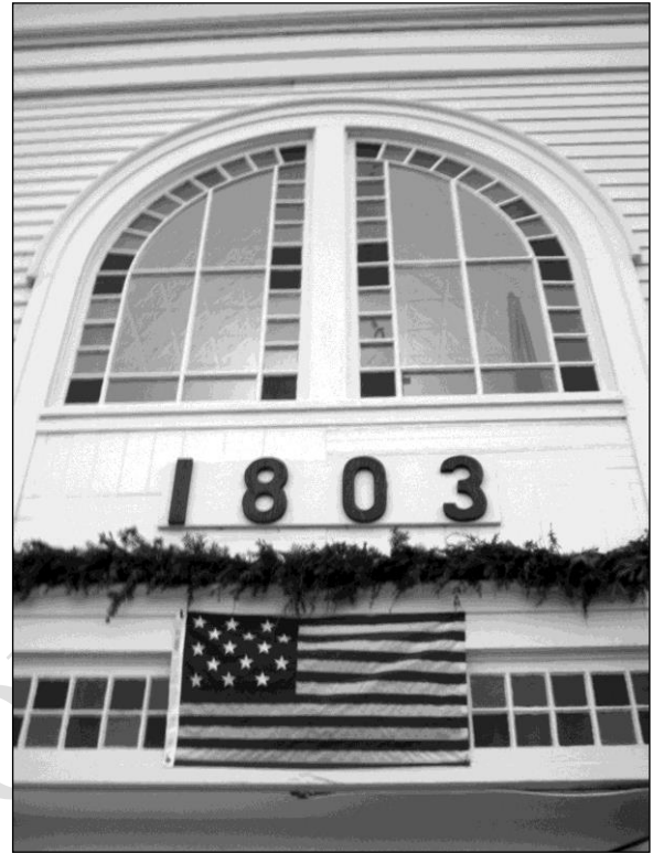
Figure 2: Facade of the Congregation Church
