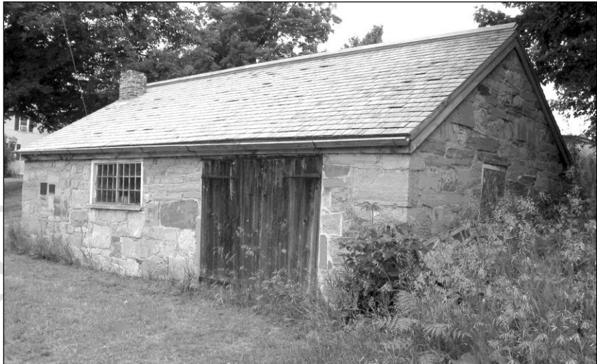
Figure 14: Blacksmith's Shop on Route 30, 1791
