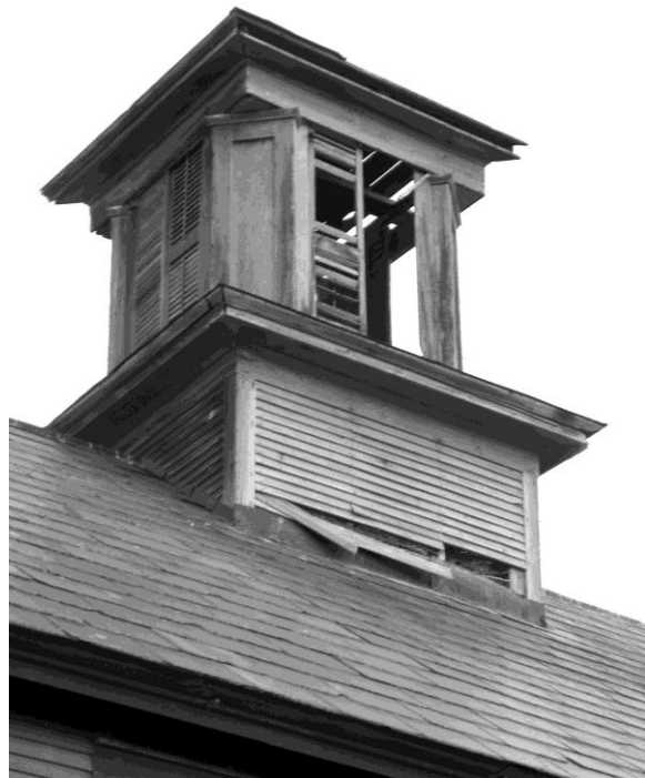
Figure 4: Cupola on a 19th Century Barn
