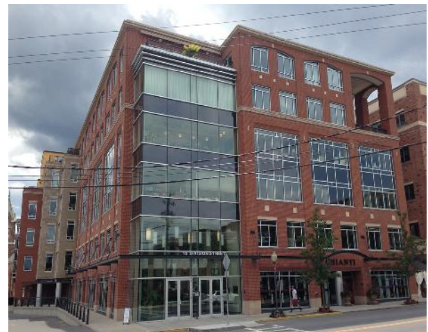
An example of an individual Mixed Use Building employing multiple Frontage Types.
