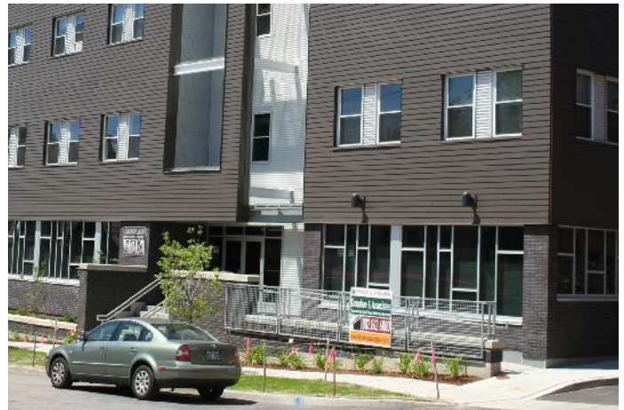
An example of a handicapped access ramp integrated into a Building Frontage.
