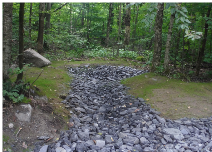
New Ditching on Notch Road (photo by: Bill Atwood)
