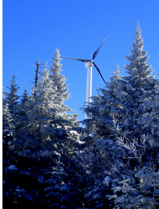
Bolton Valley Wind Turbine (photo by Lee Krohn)
