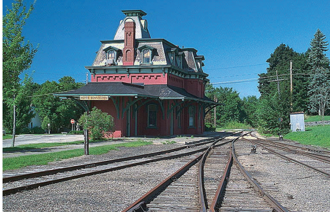
The historic railway station in North Bennington represents the past, as well as the future potential, of rail transportation in the region.
