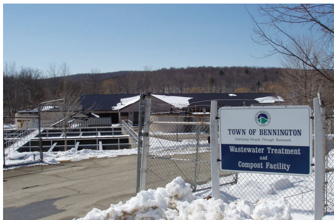
The municipal wastewater treatment plant includes an innovative sludge composting facility.
