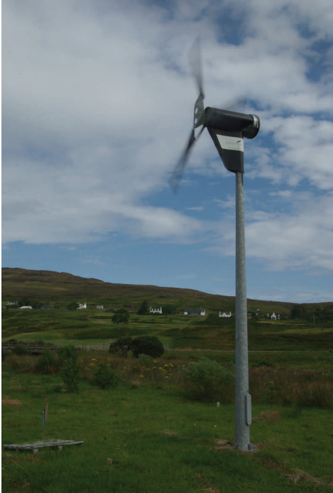
A 2.5 KW wind turbine like this one can supply most of the electricity demand for a typical home.
