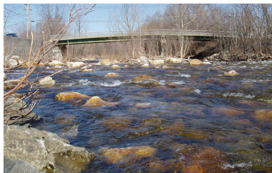
Restoration work along the Roaring Branch on the east side of town will improve water quality and floodplain management.
