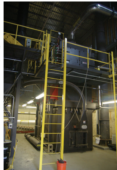
Biomass energy facility at Bennington College fueled by locally available wood chips.
