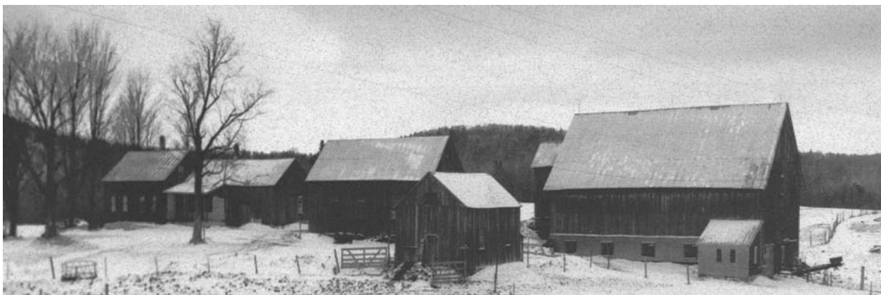
The Malone Farm in East Bakersfield includes an 1850 house on the left and a high bank dairy built in 1890 on the right. Horses pulled hay wagons piled high with loose hay up the ramp or wharf. Hay was packed into the sides of the loft and dropped down to the dairy cows in the ground floor stable below. Credit: Bakersfield Historical Society.
