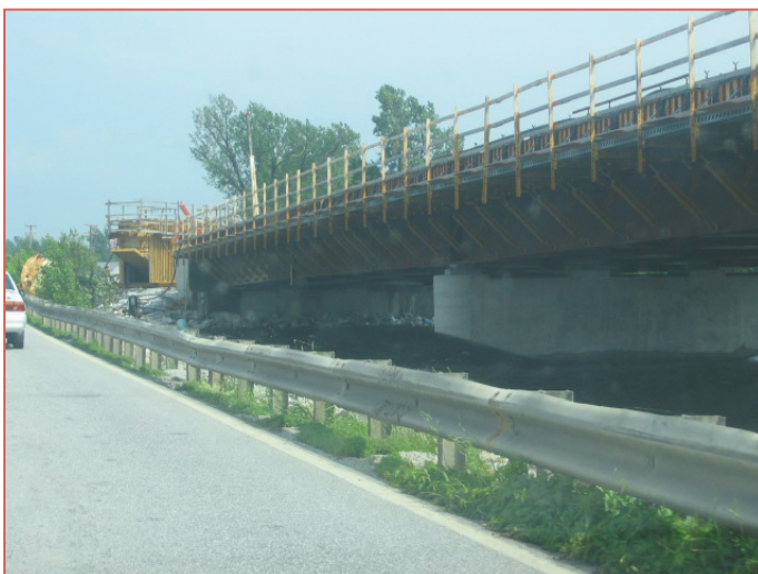
Missisquoi Bridge Under Construction
