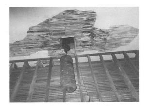
Attic conditions: I inspected all of the attic that I could safely access. The undersides of the roof sheathing boards were all dry and showed no signs of chronic leaking or decay except for minor decay and staining near the southwest chimney.
