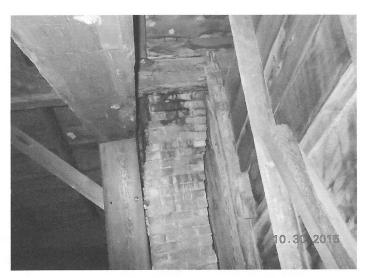
Lower level floor: The lower floor has settled more than two inches away from the wall baseboards in some areas on the east and west walls. There are two possible causes that come to mind. Either the framing has been exposed to a high moisture environment and is decaying or the support post system for the floor is settling in the soil beneath them. The initial cause is the most likely as any settlement should have ended decades ago.
