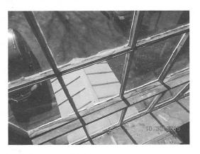
Roofing: There are quite a few missing, cracked or incomplete slates visible on the south exposure of the roof. There is a cluster of missing slate and therefore bare roof at the west rake edge of the roof. (I was unable to see the north side of the roof because of the slope of the ground to the north of the church.) There should be a regular inspection of the roof and contracted repair every two or three years or as needed.
