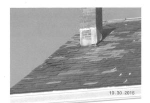
particularly for a building on the Historic Register. The slates are mismatched and what appears to be white caulk used on cracked slates. Replacement slates should be compatible with the originals and secured with slate hooks. Cracked slates can be reinforced by a piece of copper flashing inserted beneath them and extending to above the overlap of the upper slate. Caulk, roofing cement and the like should not be used as a part of the slate repair process.
