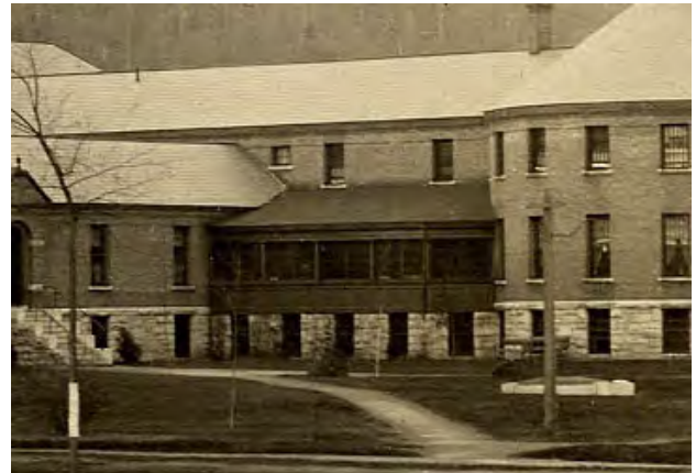
Figure 49. Historic- Porch # 1 (using North side porch to illustrate style/materials) Source: VSH Archives
