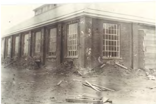
Figure 25. 1927 Flood damage at Laundry Source: VSH Archives
