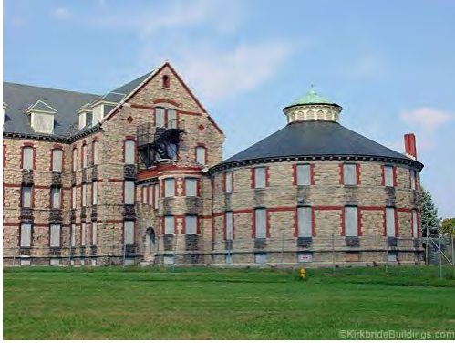
Figure 44. Hooper Hall, Worcester State Hospital
