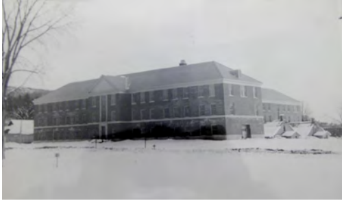
Figure 29. View of Public Safety Building Source: VSH Archives
