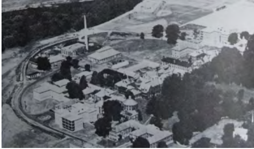
Figure 33. Aerial view showing earthen dike along the rear of buildings
