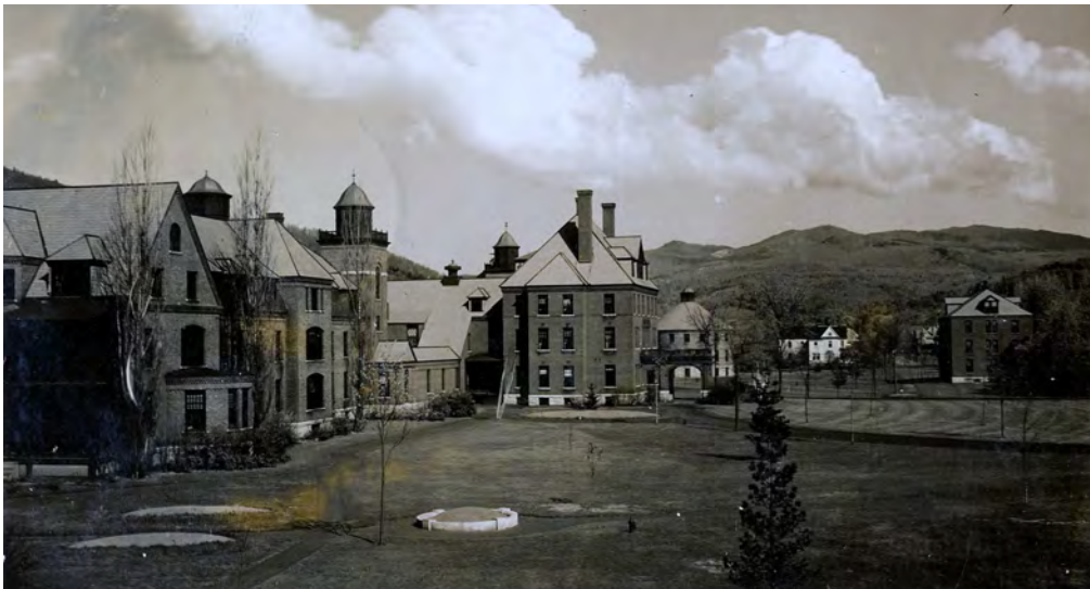
Figure 17. View of front lawn. Note fountain bed in the foreground
