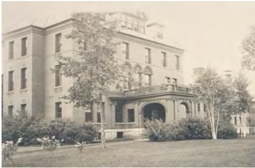
Figure 34. Front Porch on Center Building, c.1911
