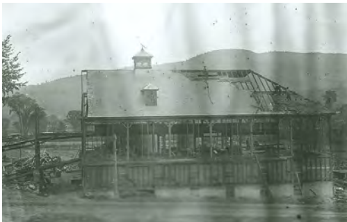
Figure 26. 1927 Flood damage at Asylum Barn Source: VSH Archives
