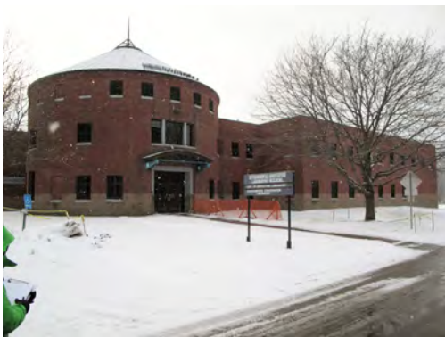
Figure 38. View of Agricultural & Environmental Resource Building
