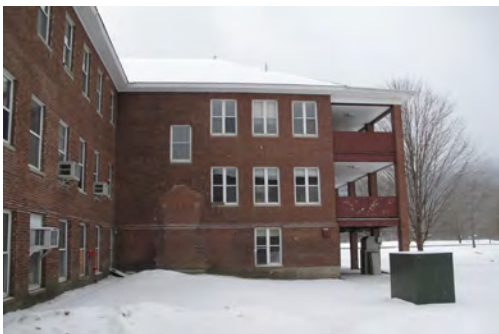
Figure 27. View of A Building Source: GCA
