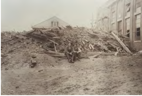
Figure 24. 1927 Flood damage behind Power House Source: VSH Archives
