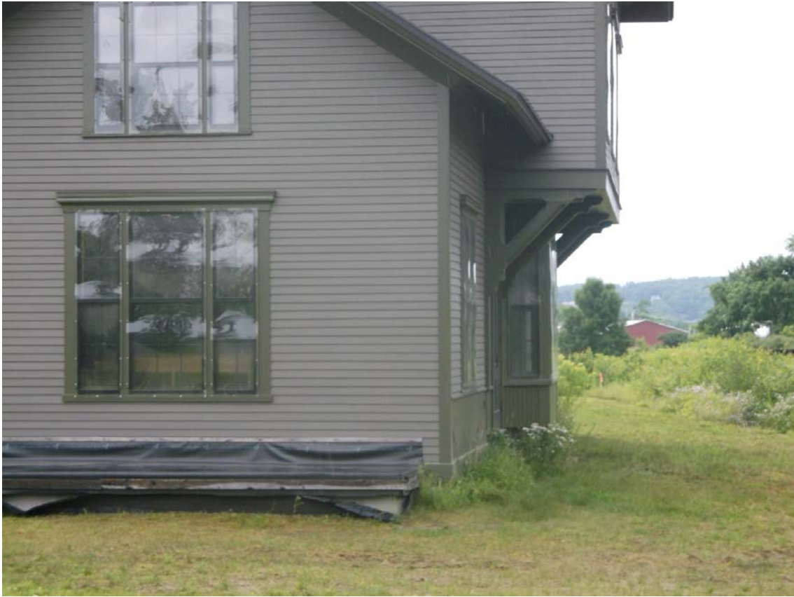
Photo 9. View S, showing the Vergennes Depot in its new location on the east side of the railroad tracks. The Operator's Bay on the rear (now west) elevation is not original to the first generation RR building but was added later in the 19th century. The bay was a typical feature on later Depots.
