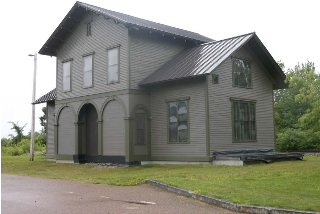
Photo 7. View SW, showing the east and north elevations of the relocated depot. The tracks are now on the west side of the building.
