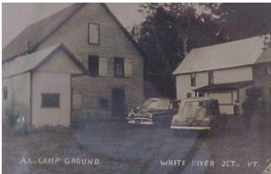
Figure 14. Dormitory, Kitchen and Bookstore
