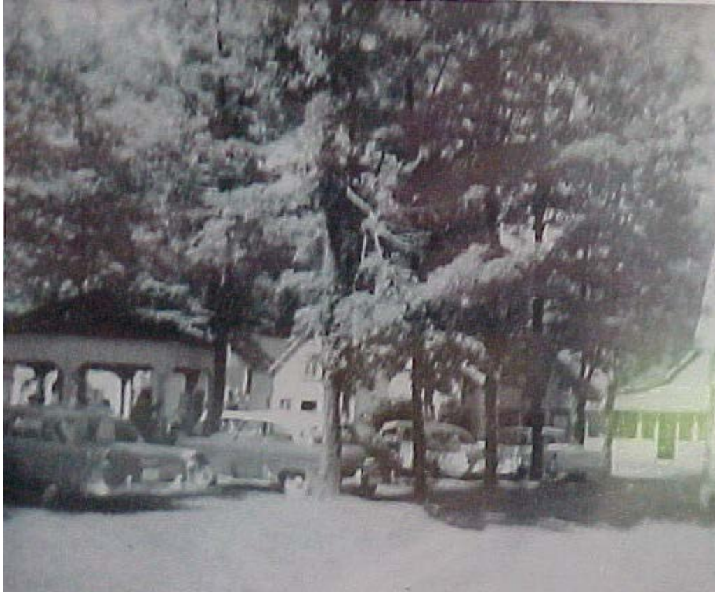
Figure 6 View of Baptistery from southwest
