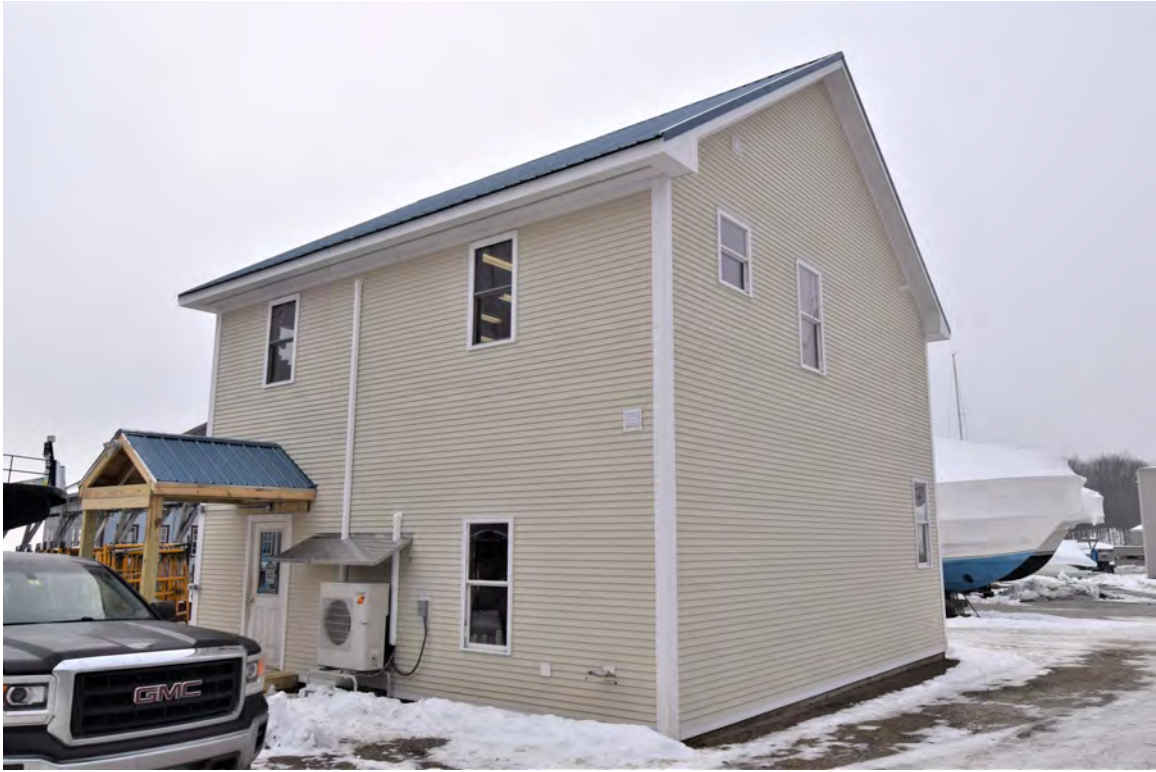
Photo 55: Building #5, view looking west
