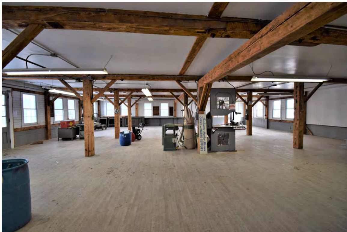
Photo 40: Building #4, view looking southwest in main block second floor
