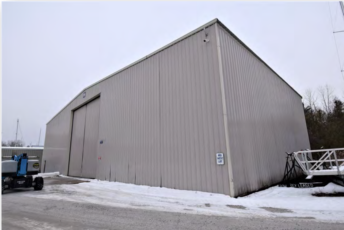
Photo 60: Building #9, view looking west
