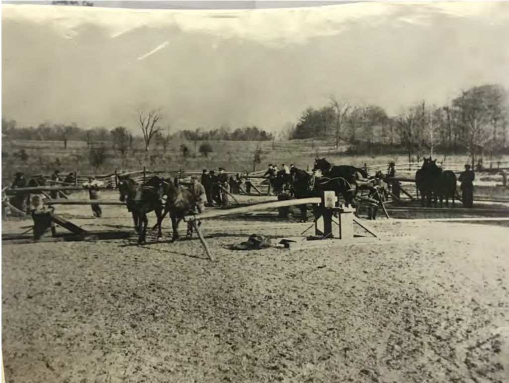
Photo 103: View shows teams of horses, each hitched to a windlass that wound ropes connected in the gear house to the southeast, shown below. Photo before 1929
