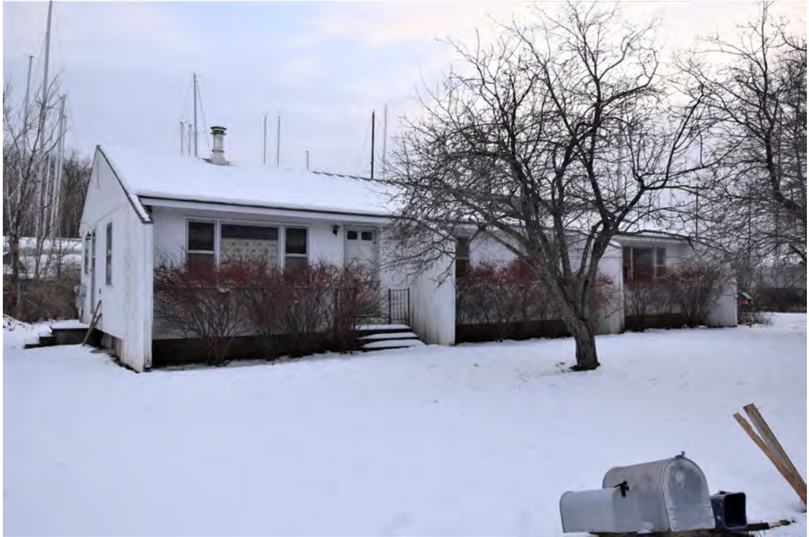
Photo 75: Building #13, view looking southwest
