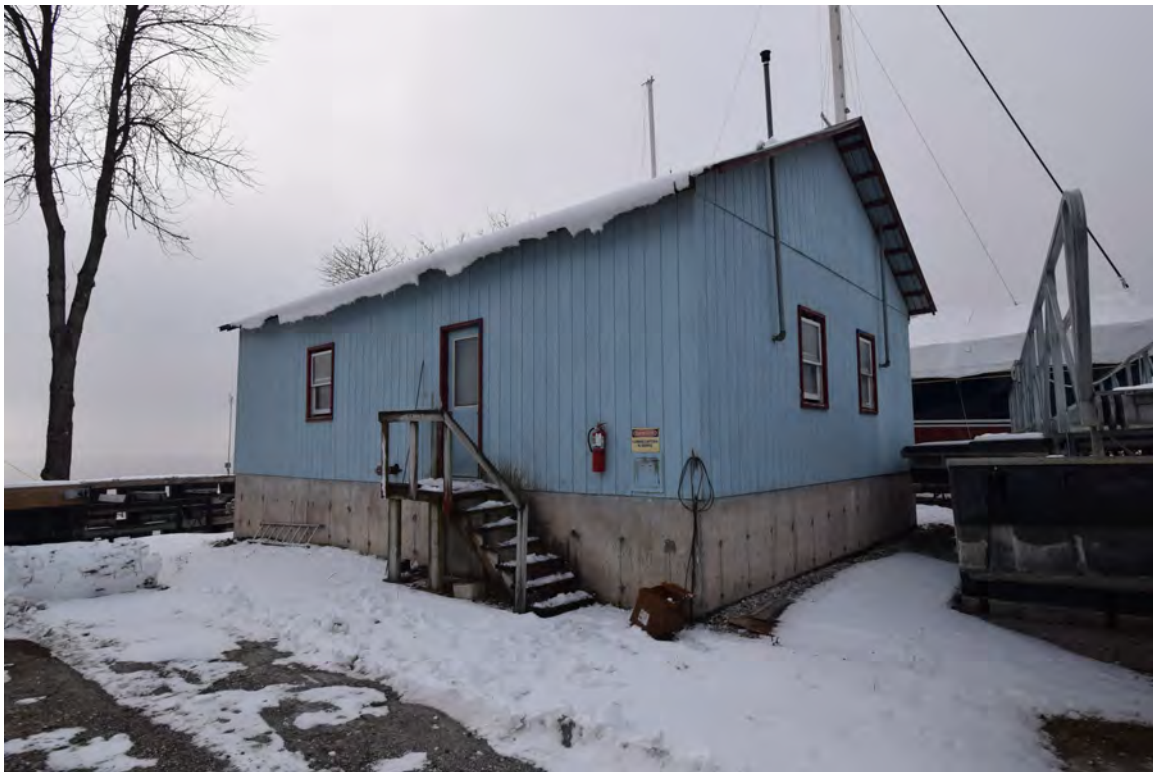
Photo 10: Building #3, view looking south
