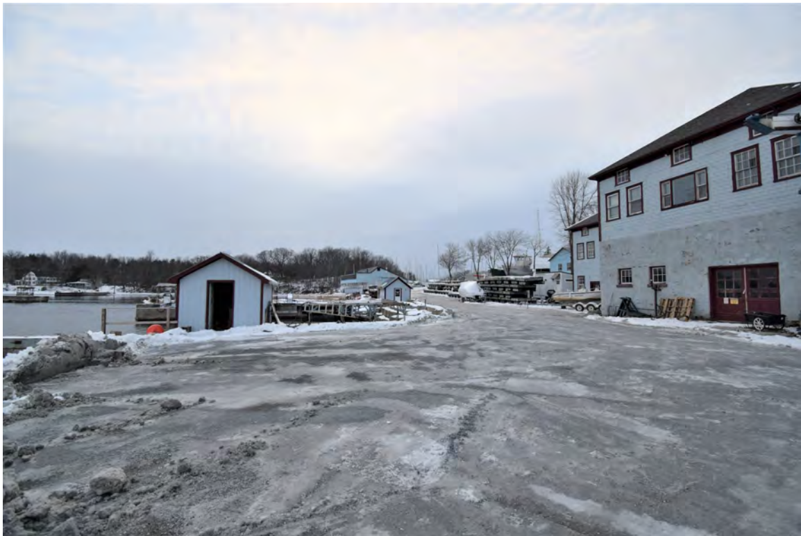
Photo 88: General View: looking southwest, view shows unnumbered utility shed at left, building #4 at right
