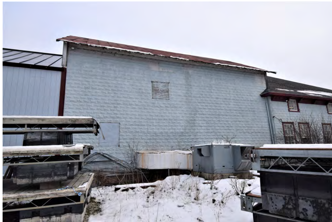
Photo 18: Building #4, view looking northeast
