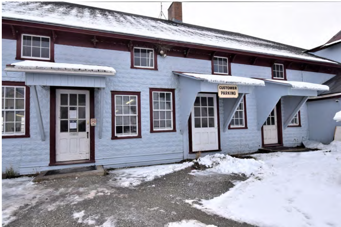
Photo 20: Building #4, view looking south
