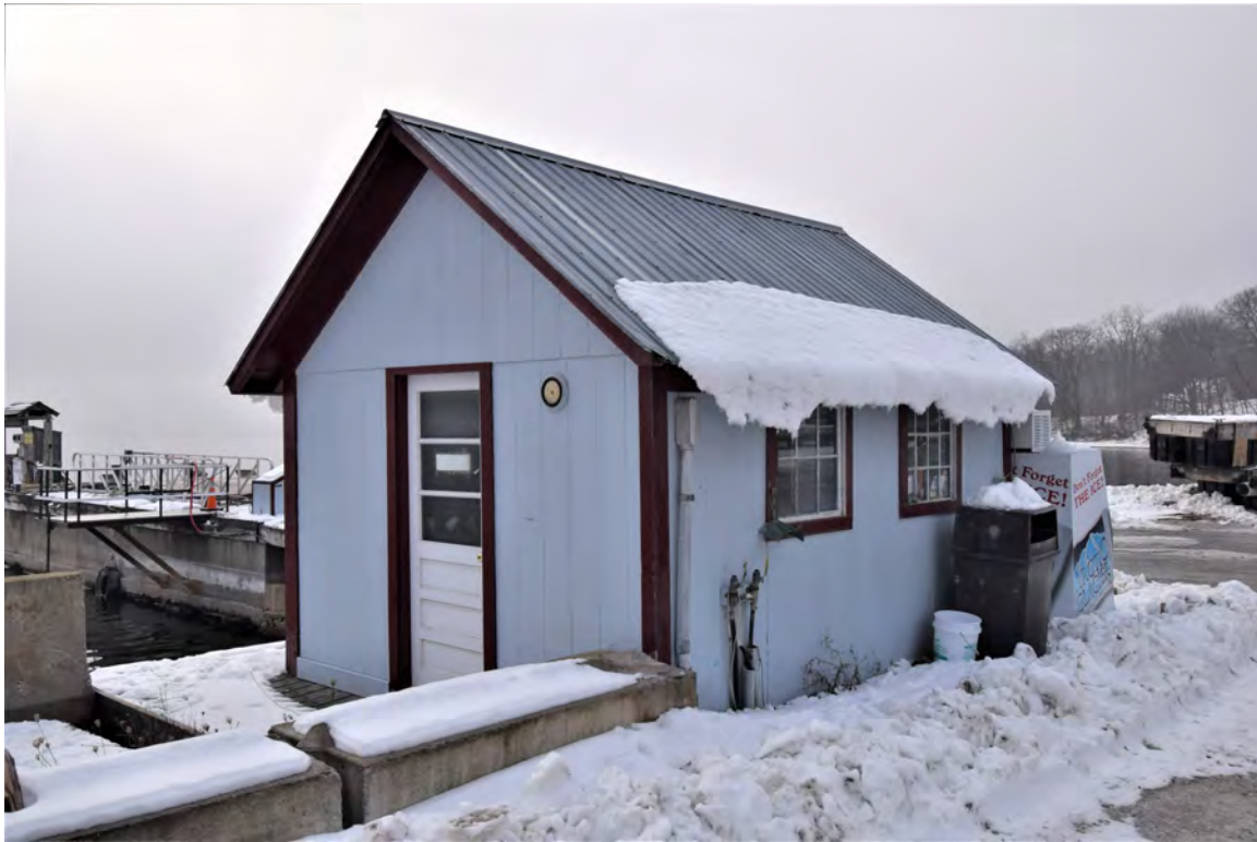
Photo 79: Building #15, view looking south
