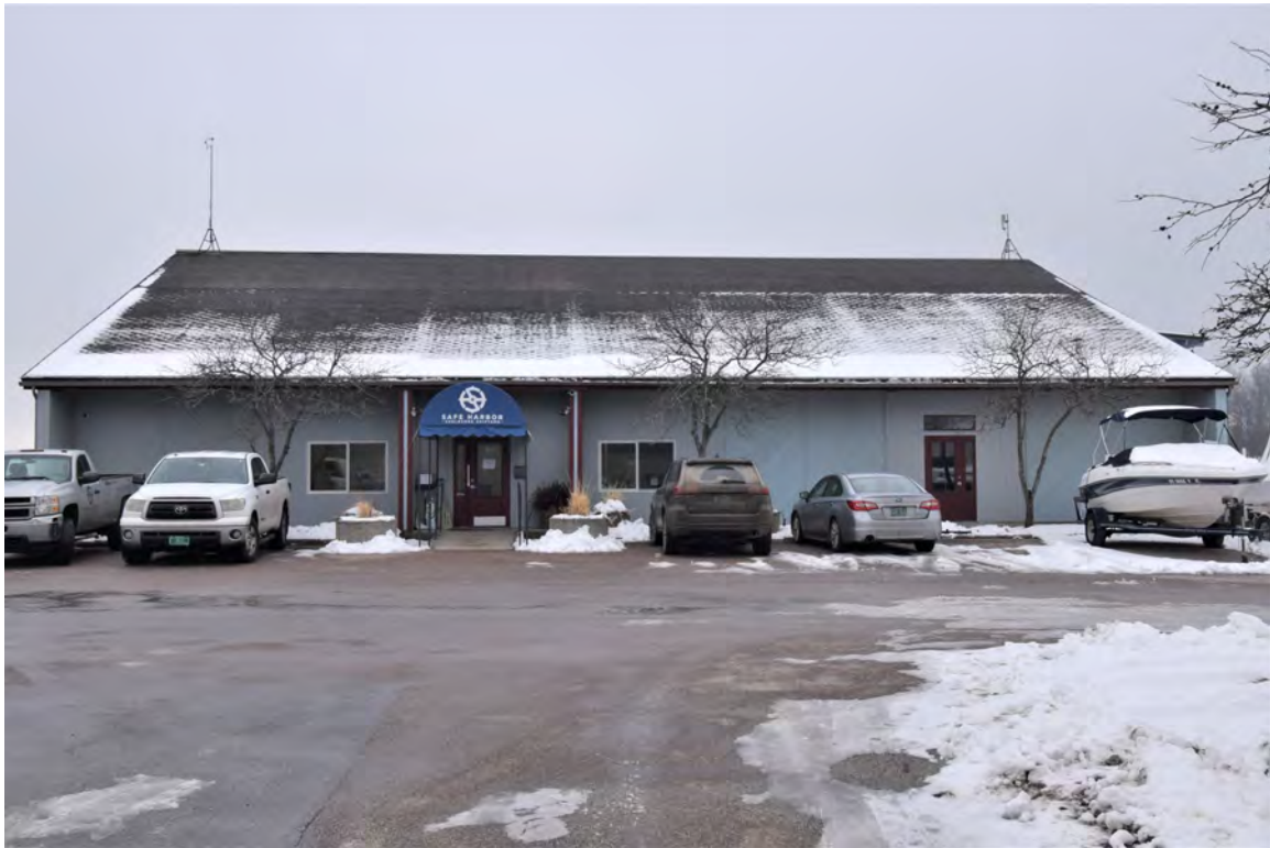
Photo 1: Building #1, view looking northwest
