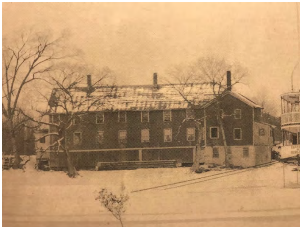
Photo 97: view shows closeup of boarding house (building #1) from photo 95
