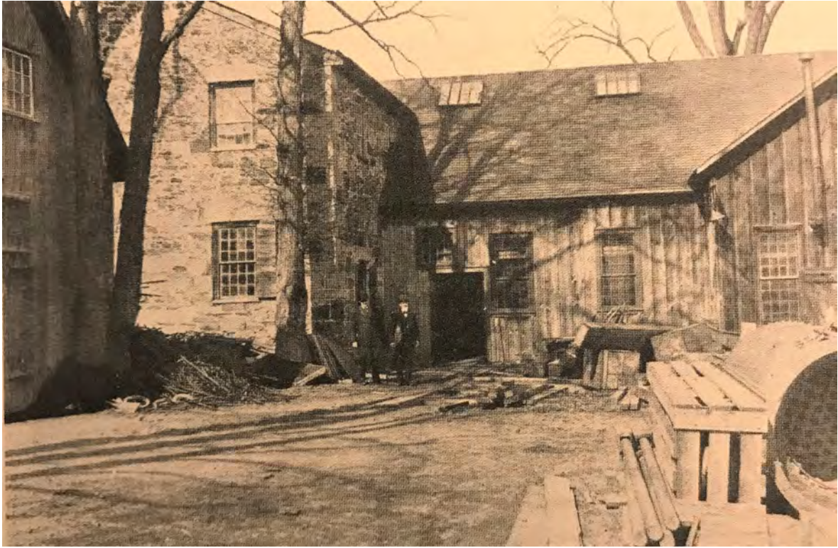
Photo 91: View shows Old Stone Shop, built 1827, burned 1910 with several other manufacturing buildings
