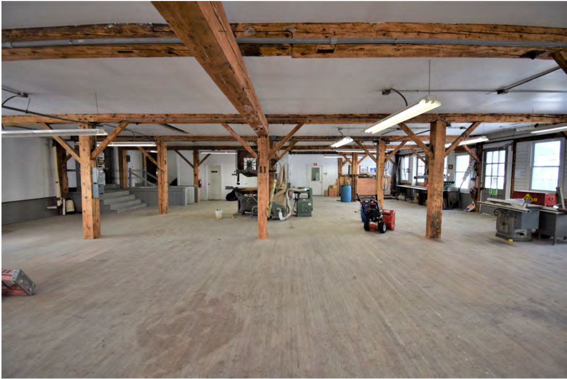
Photo 39: Building #4, view looking northeast in main block second floor
