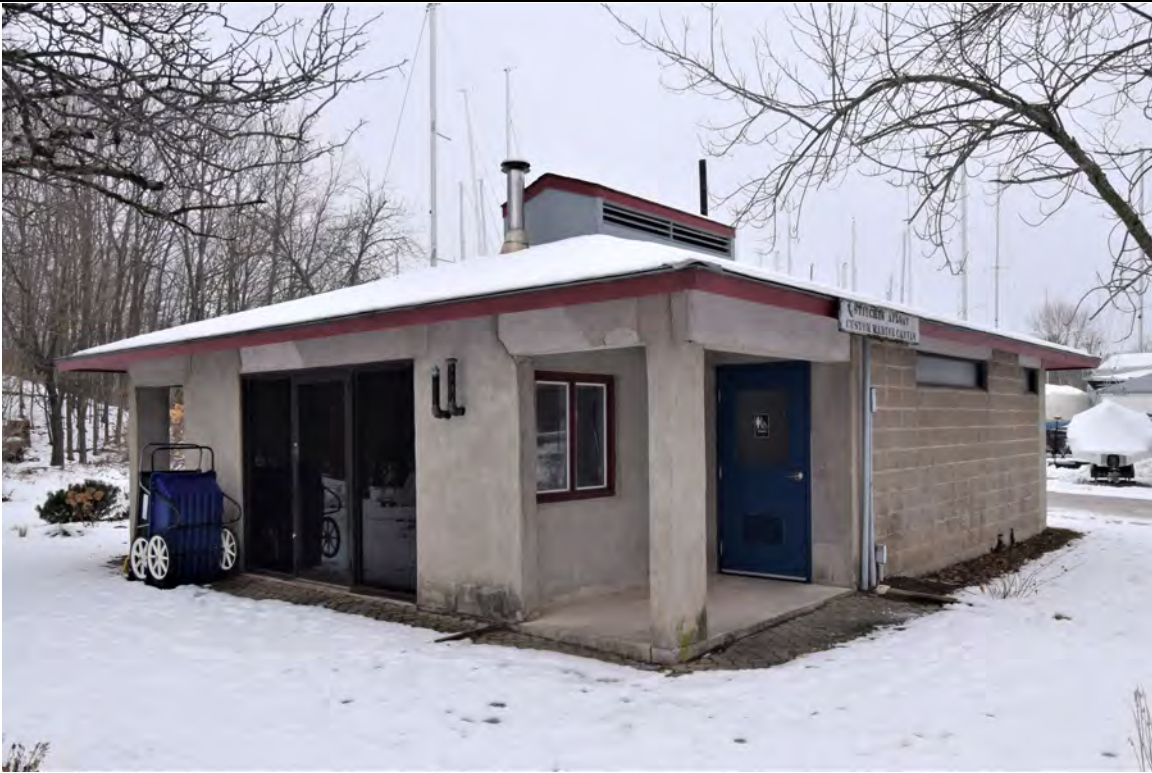
Photo 57: Building #8, view looking west
