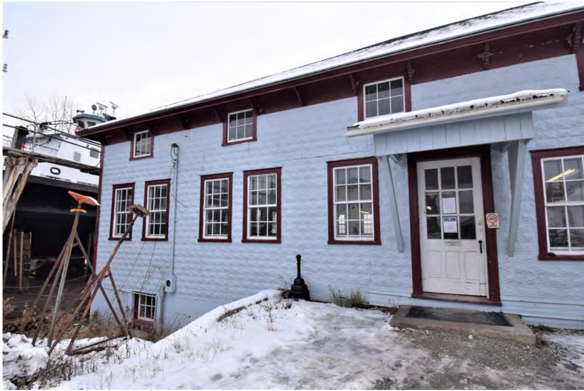
Photo 21: Building #4, view looking east
