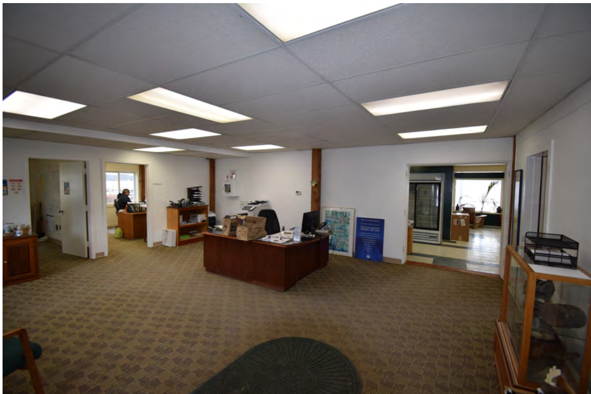
Photo 6: Building #1: view shows first floor general conditions
