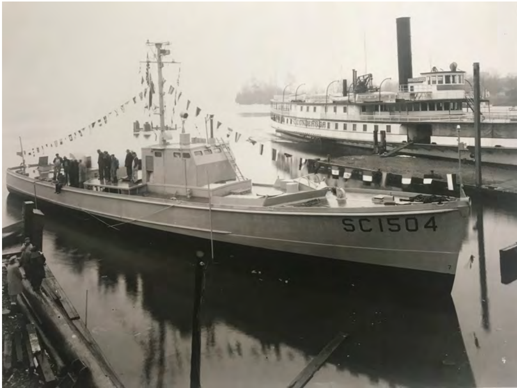
Photo 109: Looking southwest, view shows one of several 110' "sub-chasers" commissioned by the US Navy during WWII and built by Donovan Construction Co. at Shelburne Shipyard
