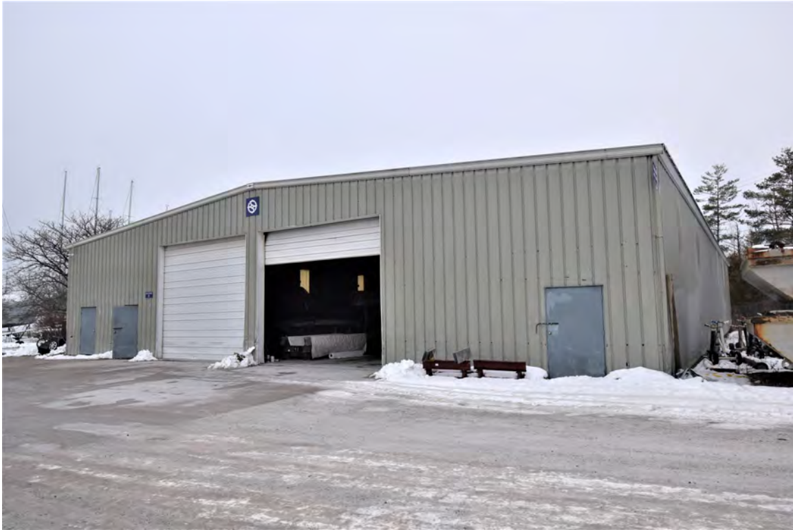
Photo 9: Building #2, view looking northwest
