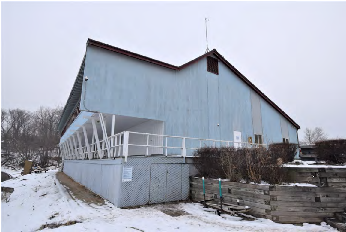
Photo 5: Building #1, view looking southwest
