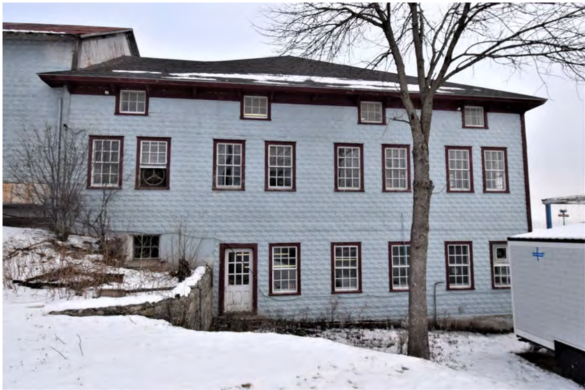
Photo 16: Building #4, view looking northeast
