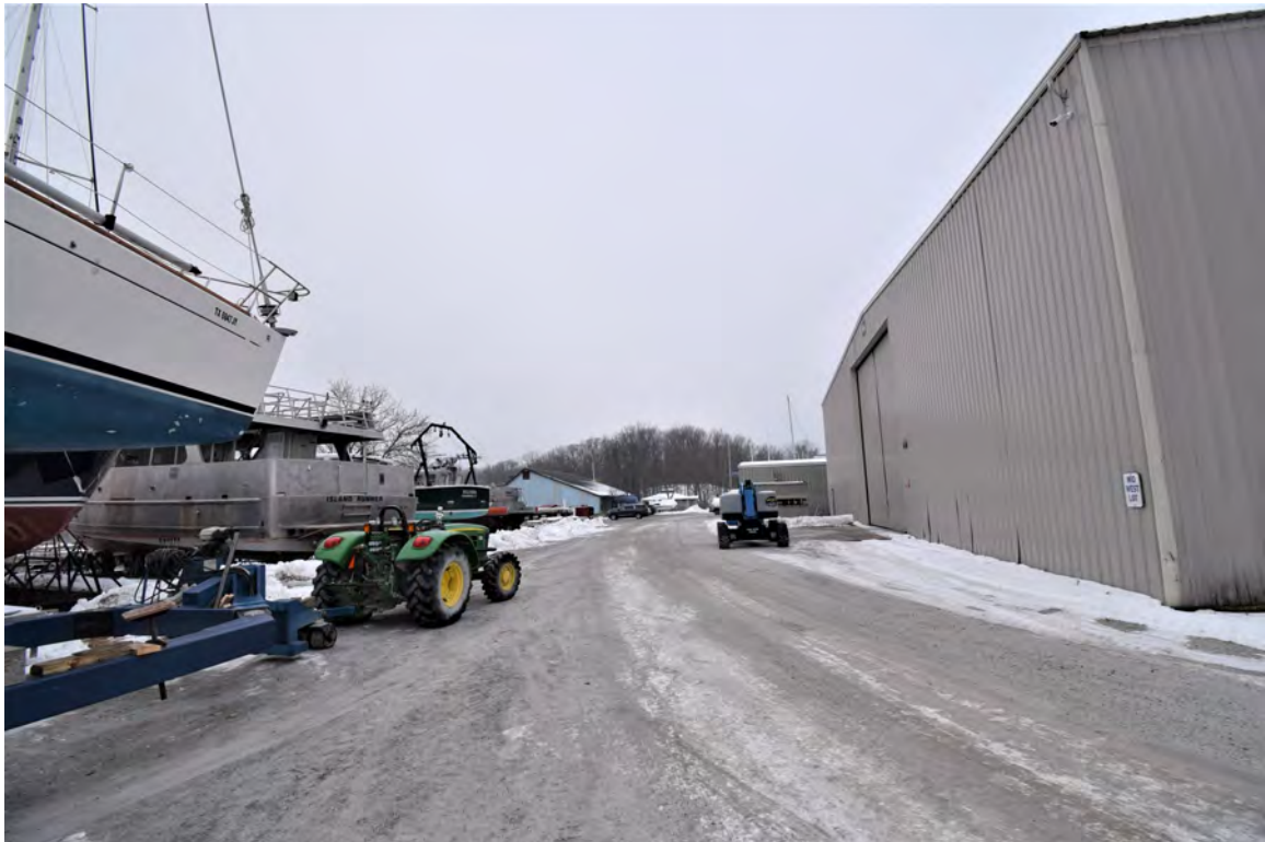
Photo 84: General View: looking southwest, building # 9 in right foreground
