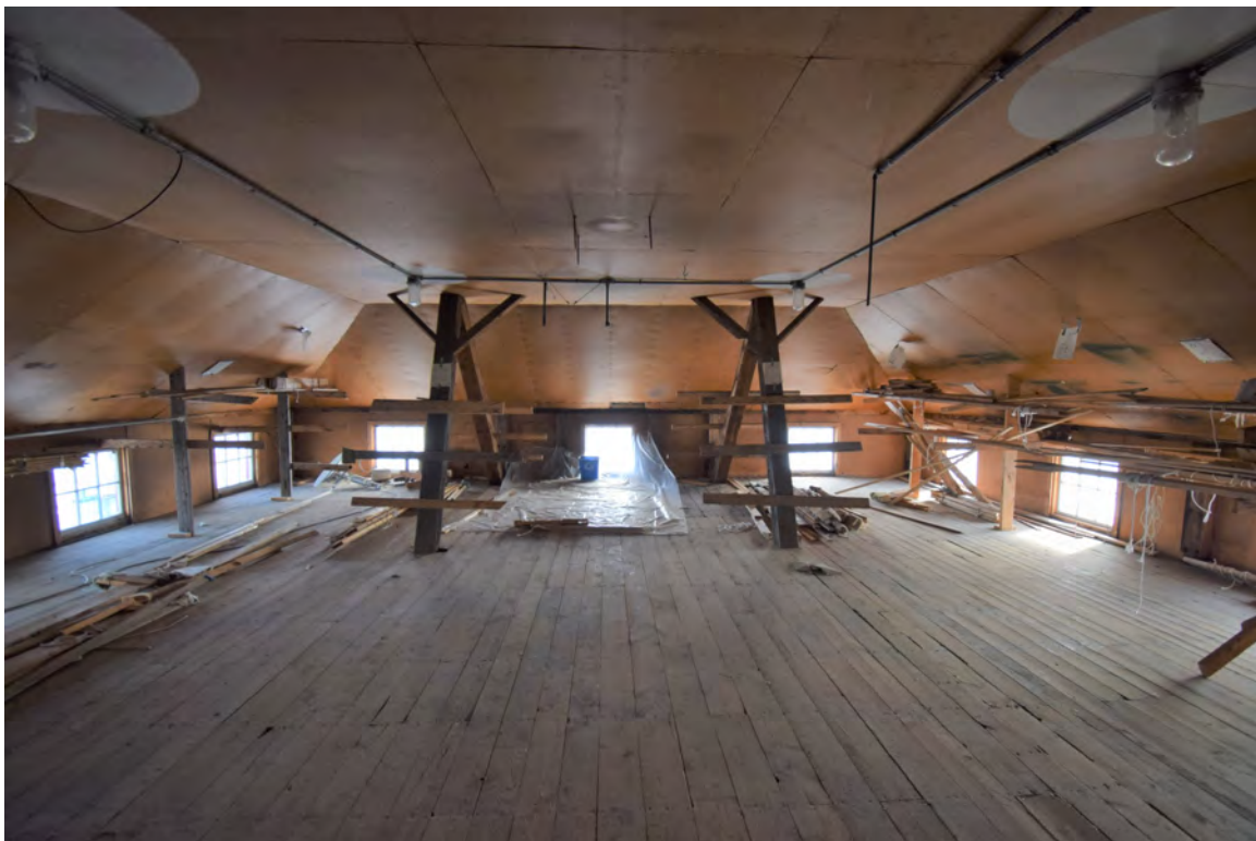
Photo 50: Building #4, view looking southeast in lakeside pavilion third floor; note kneewall windows and timber diagonals supporting gable/hip roof connection
