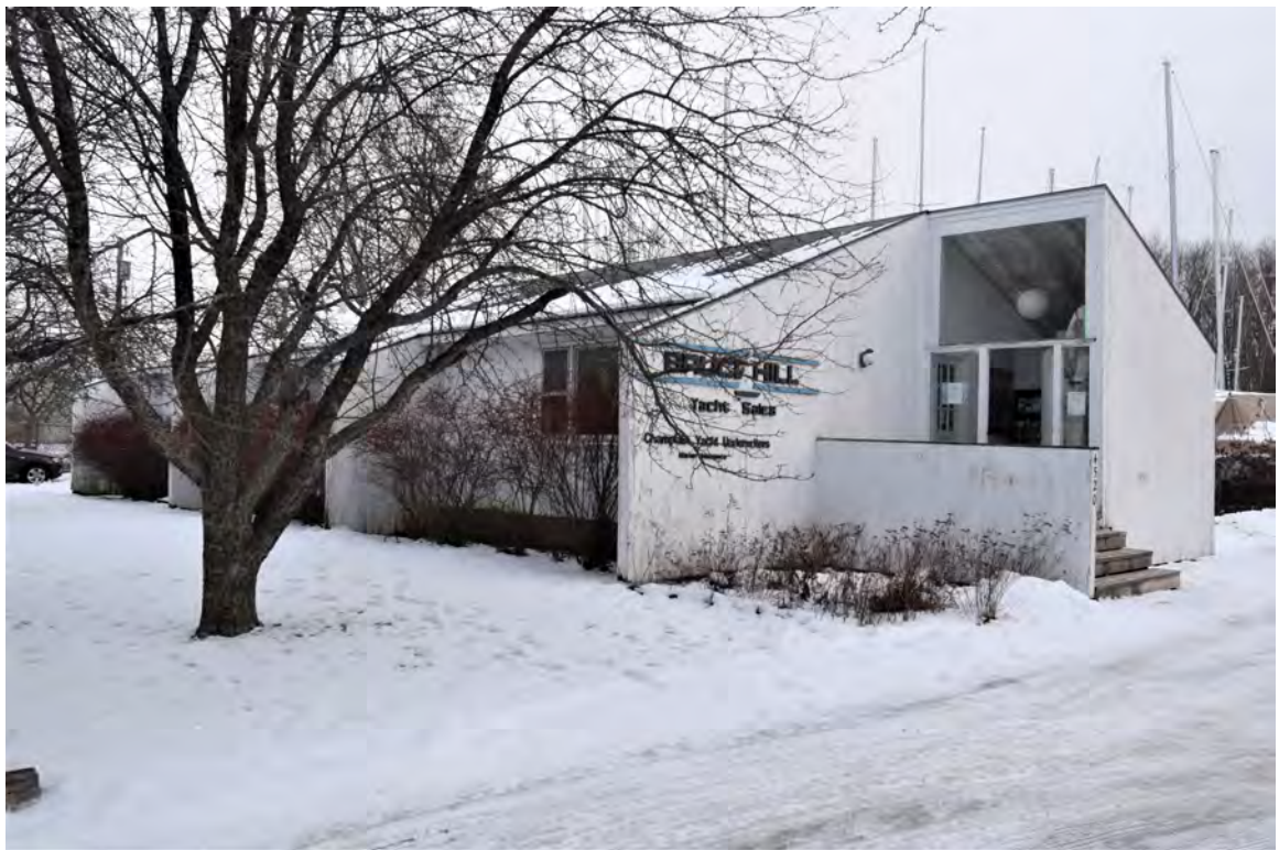
Photo 76: Building #13, view looking southeast
