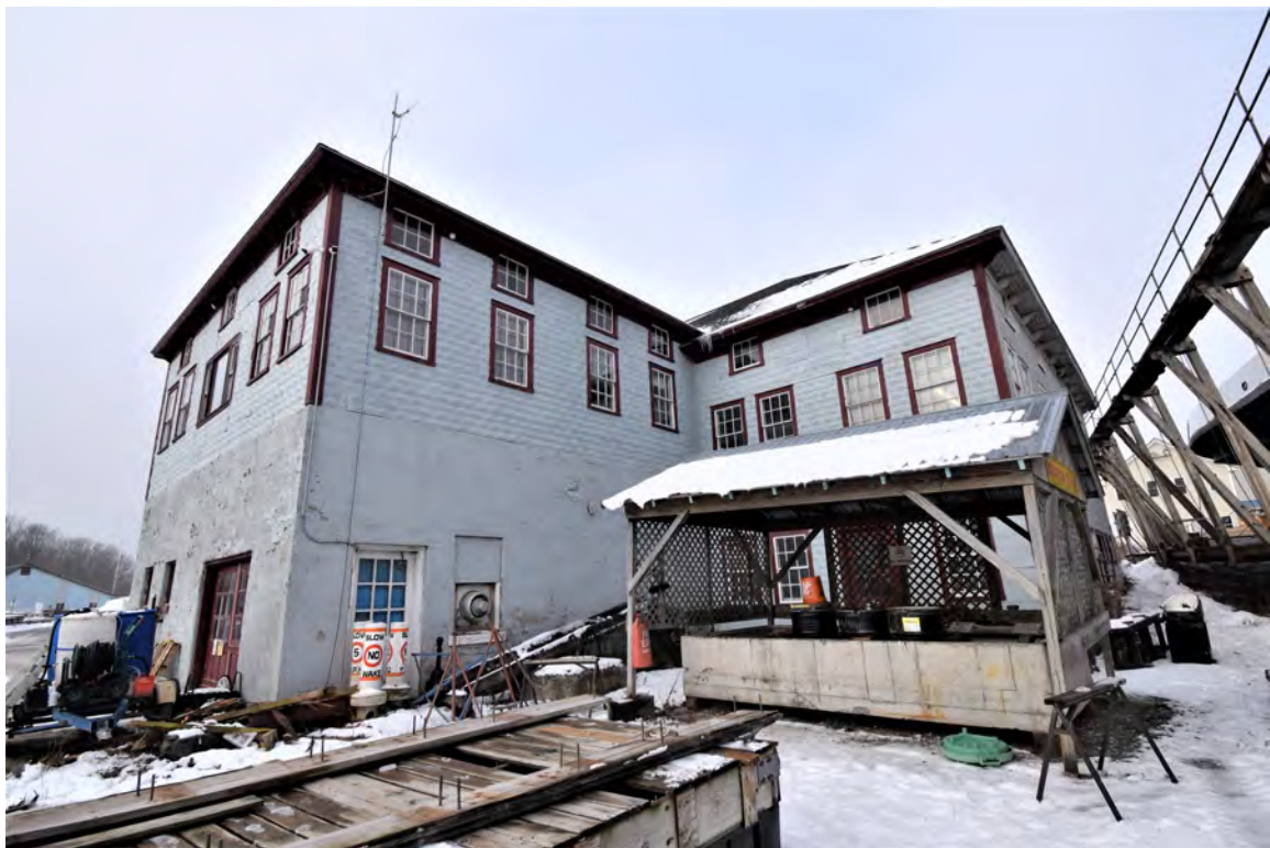
Photo 14: Building #4, view looking northwest
