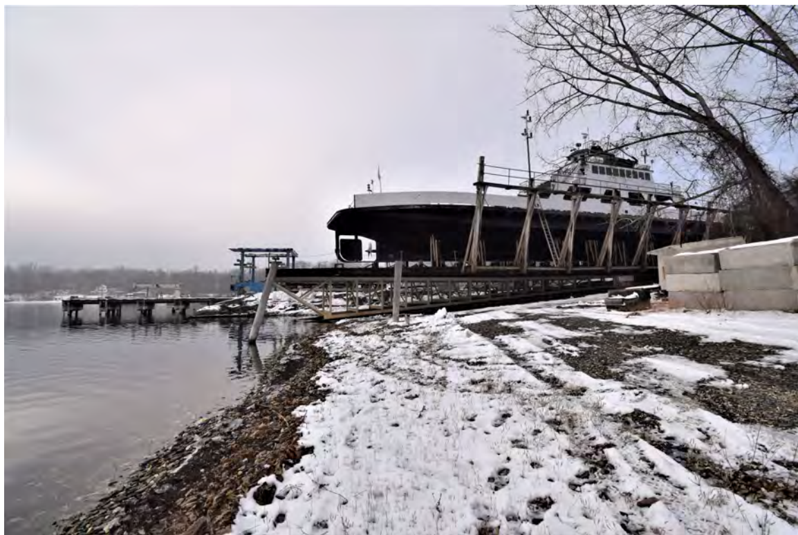
Photo 68: Structure #12, view looking southwest
