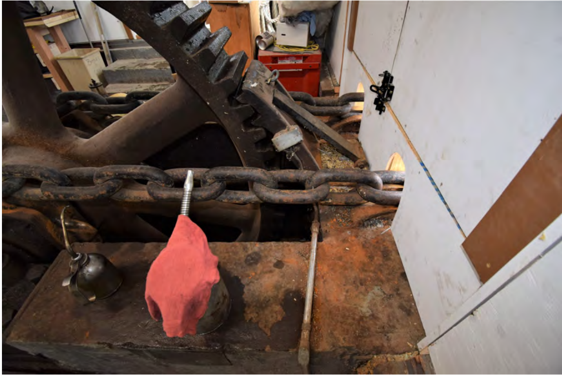
Photo 73: Structure #12, view looking northeast
