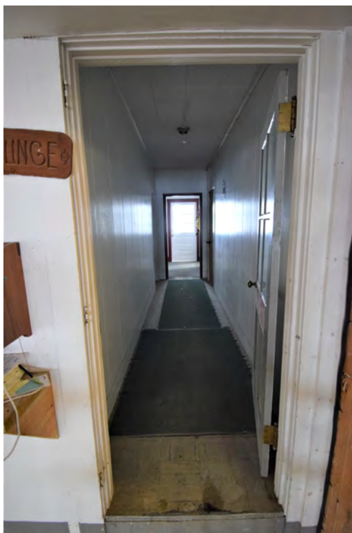
Photo 42: Building #4, view looking southeast from main block second into lakeside pavilion
