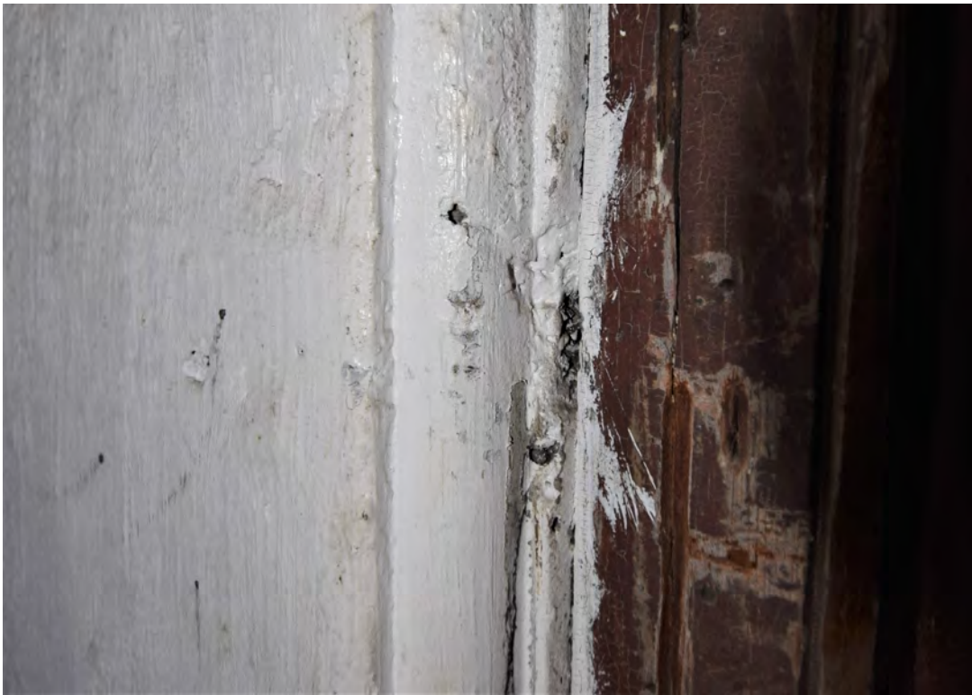
Photo 38: Building #4, view shows concrete detailing at door frames in lakeside pavilion first floor
