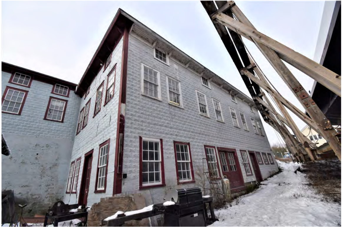
Photo 13: Building #4, view looking northwest
