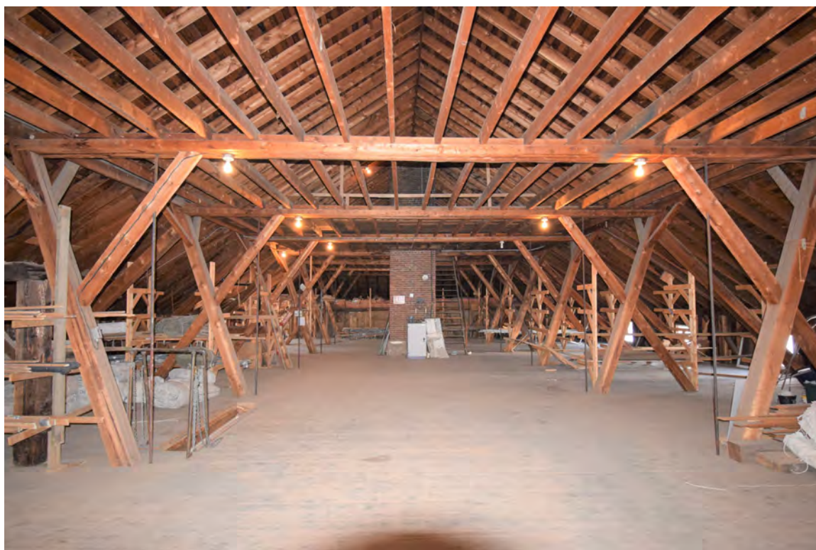
Photo 46: Building #4, view looking southwest in main block third floor
