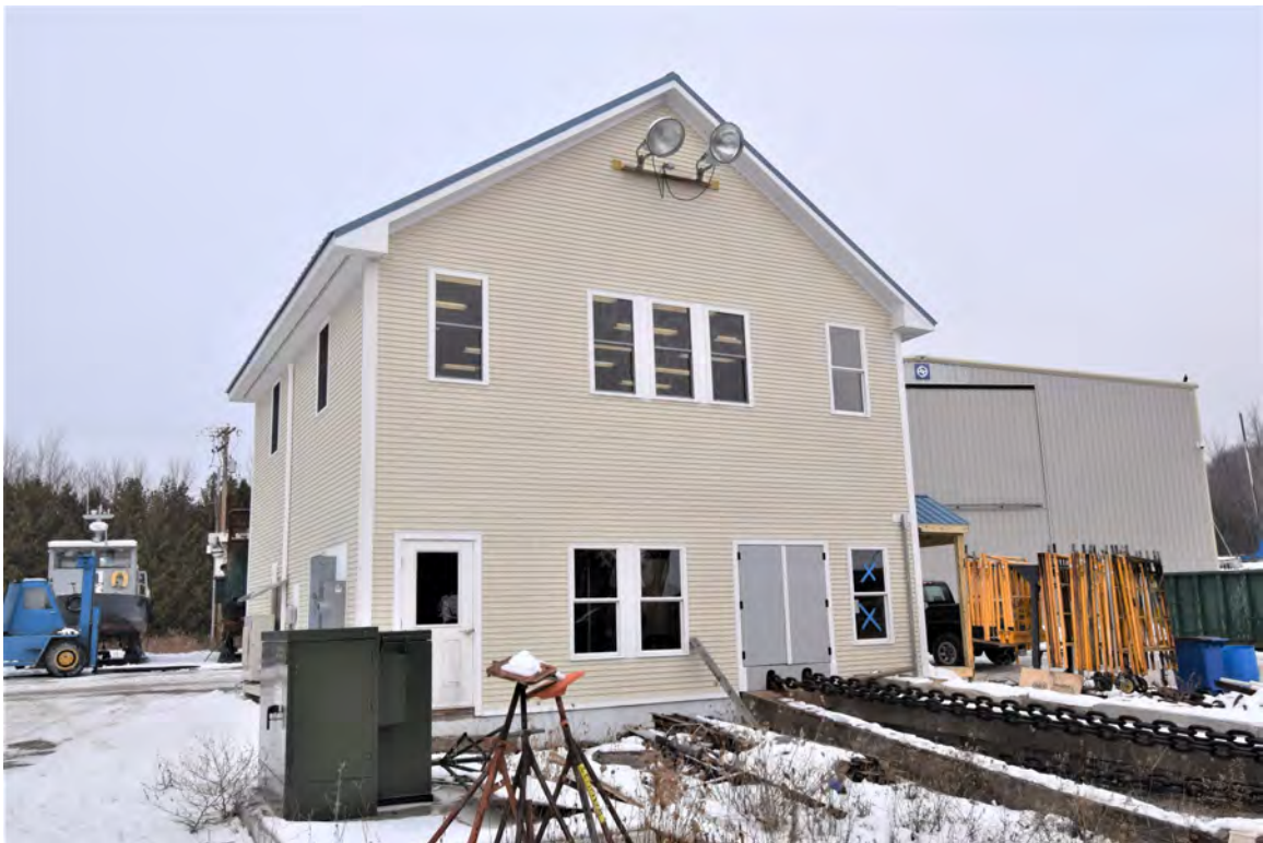
Photo 56: Building #5, view looking northwest
