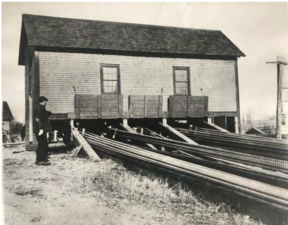
Map 104: Looking northwest, view shows gear house where block and tackle rendered enough mechanical advantage through dozens of hemp ropes to haul steamers from the water on greased skids.
