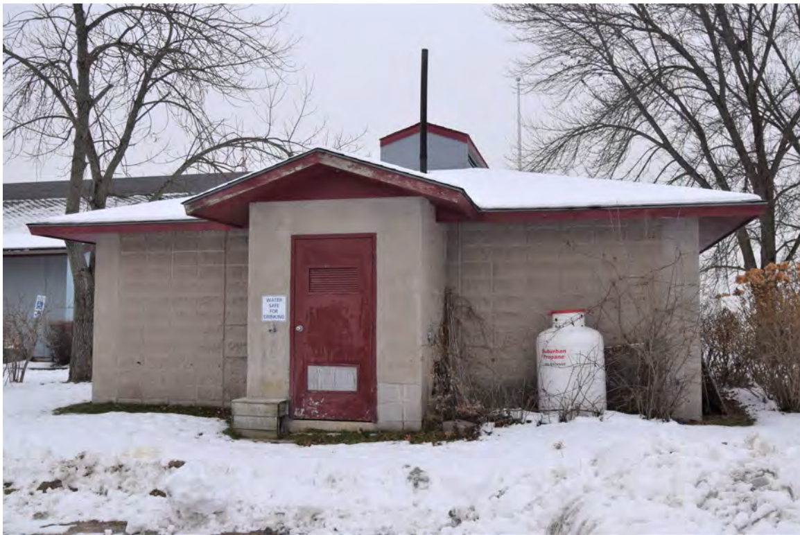
Photo 58: Building #8, view looking southeast
