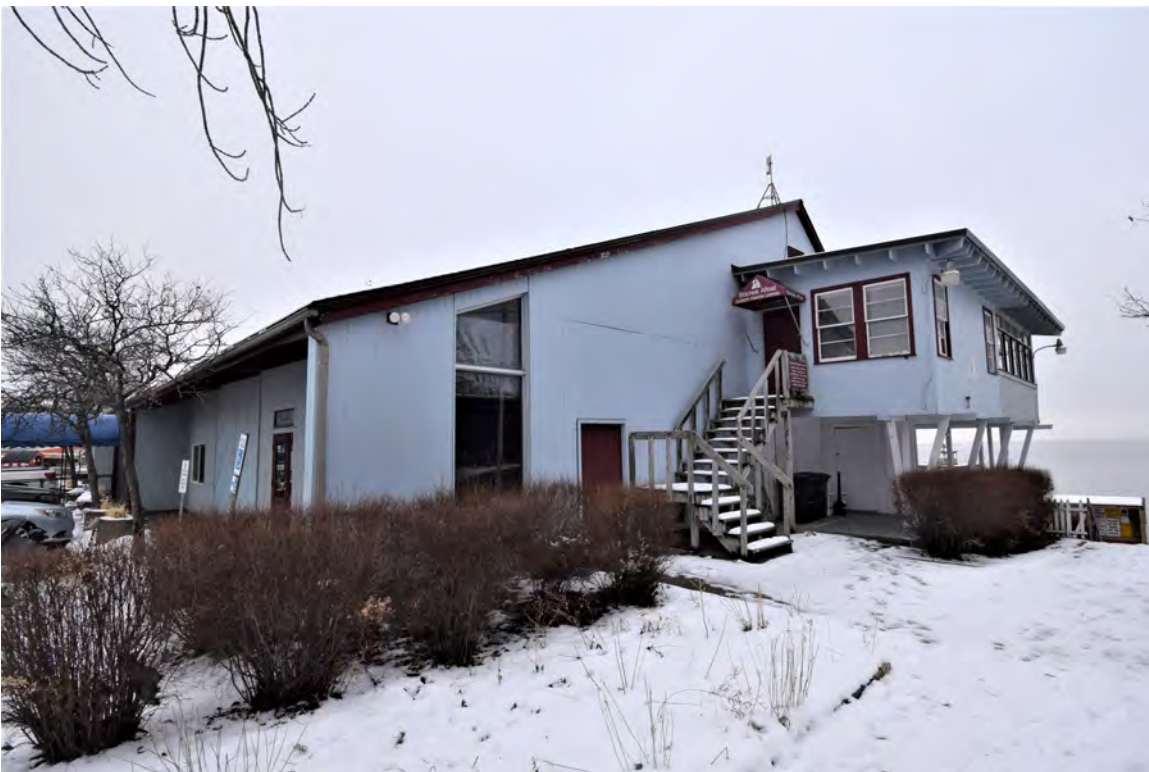
Photo 2: Building #1, view looking east
