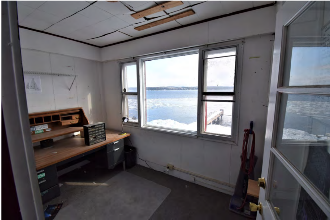
Photo 43: Building #4, view shows on of three second floor offices in the lakeside pavilion
