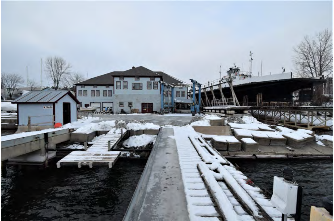
Photo 89: General View: looking northwest, view from “drop well” shows building #4 in center background, boat launch #12 at right
