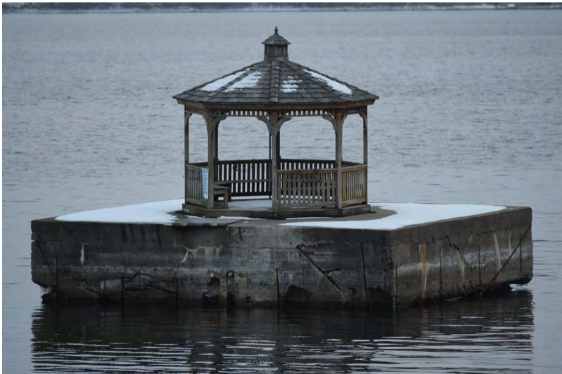
Photo 78: Structure #14, view looking southeast
