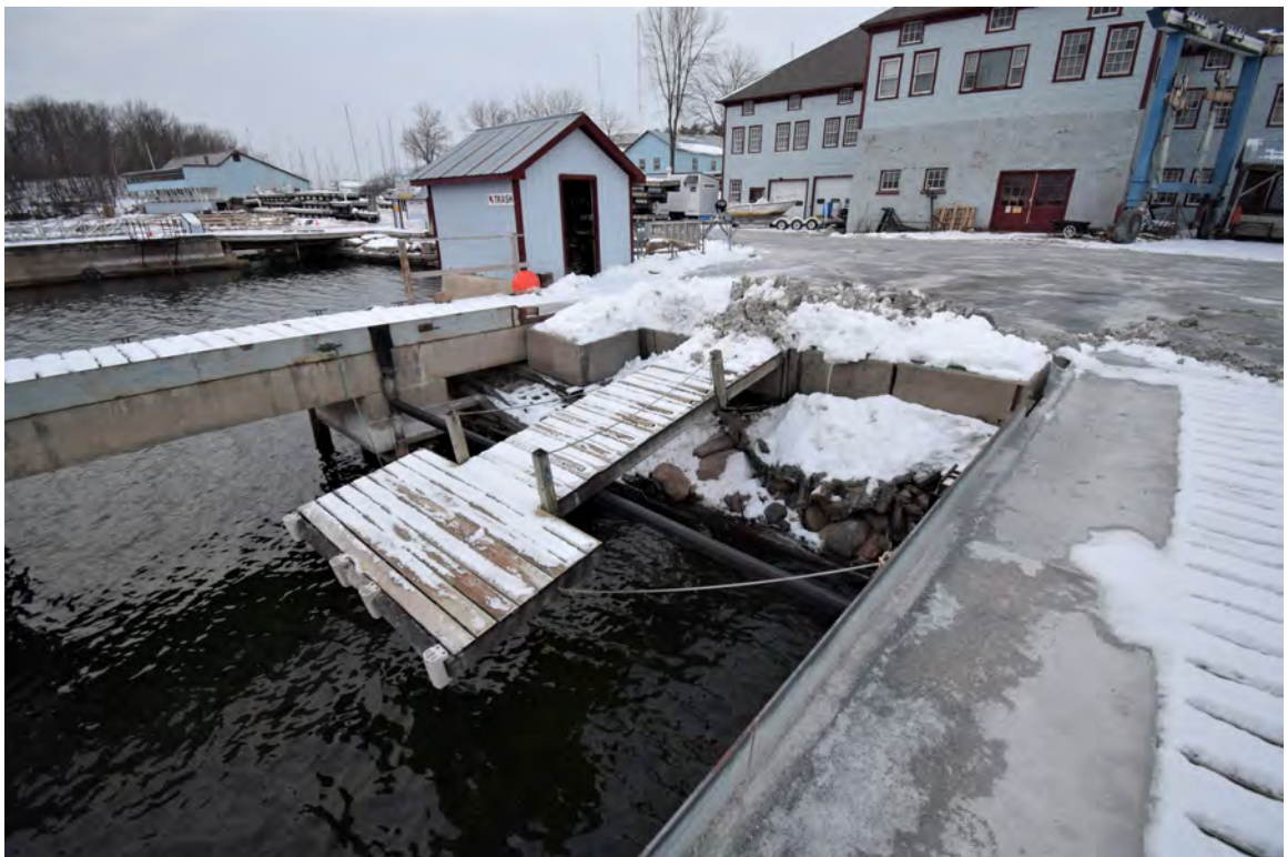
Photo 90: General View: looking west, view shows building #4 at right, and building #1 in left background
