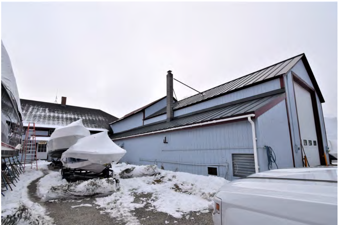
Photo 12: Building #4, view looking south
