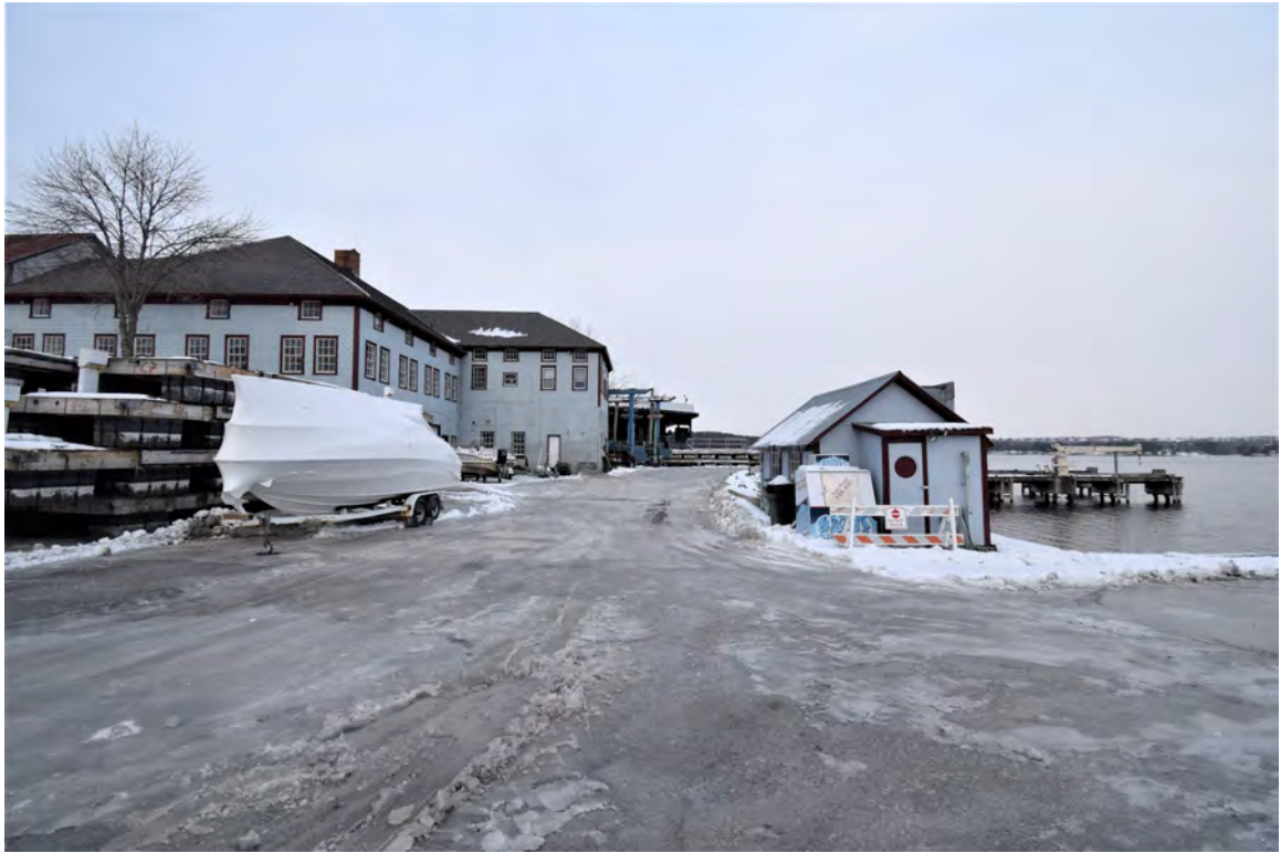
Photo 87: General View: looking northwest, building #4 at left, building #15 at right
