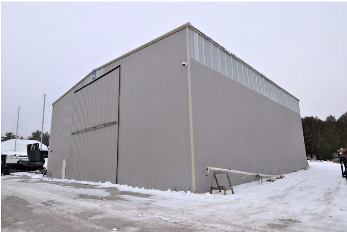
Photo 66: Building 11, view looking west
