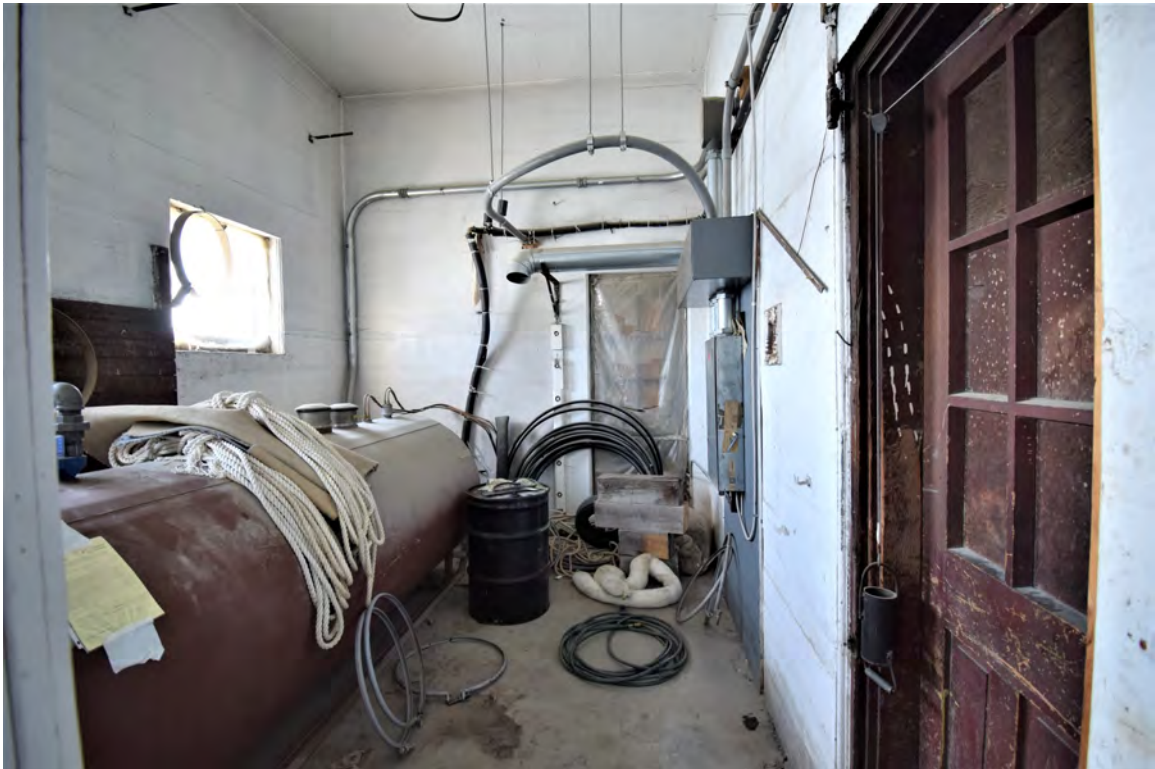
Photo 36: Building #4, view shows room 2 of 3 in the lakeside pavilion first floor
