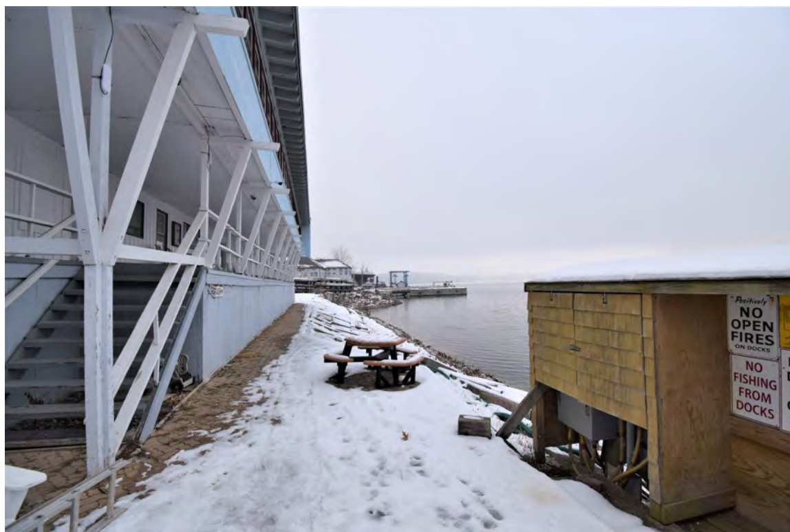
Photo 4: Building #1, view looking northeast
