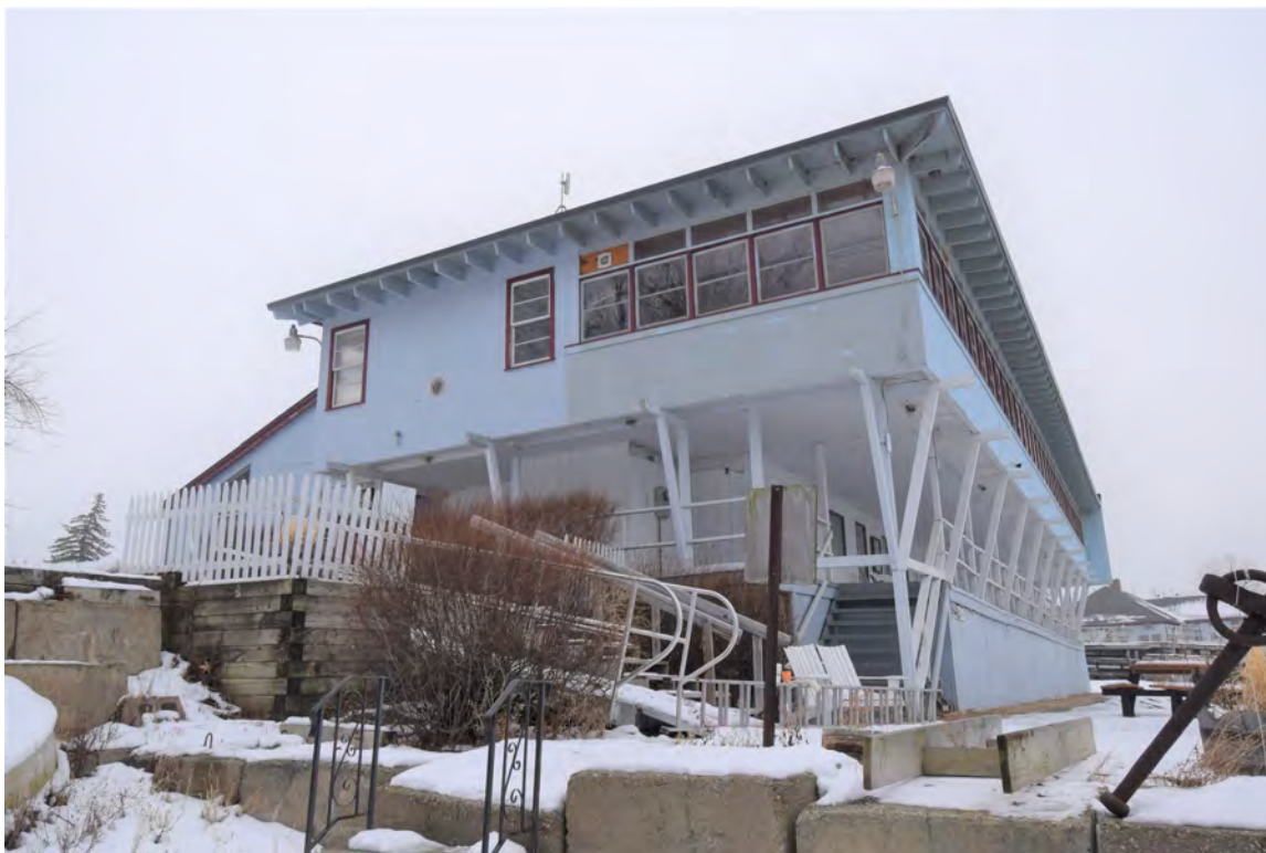
Photo 3: Building #1, view looking northeast
