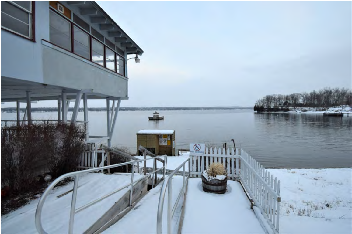
Photo 77: Structure #14, view looking southeast with resource in center background
