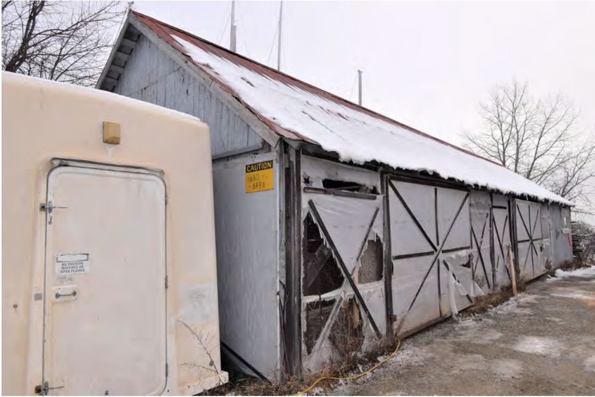
Photo 61: Building #10, view looking east
