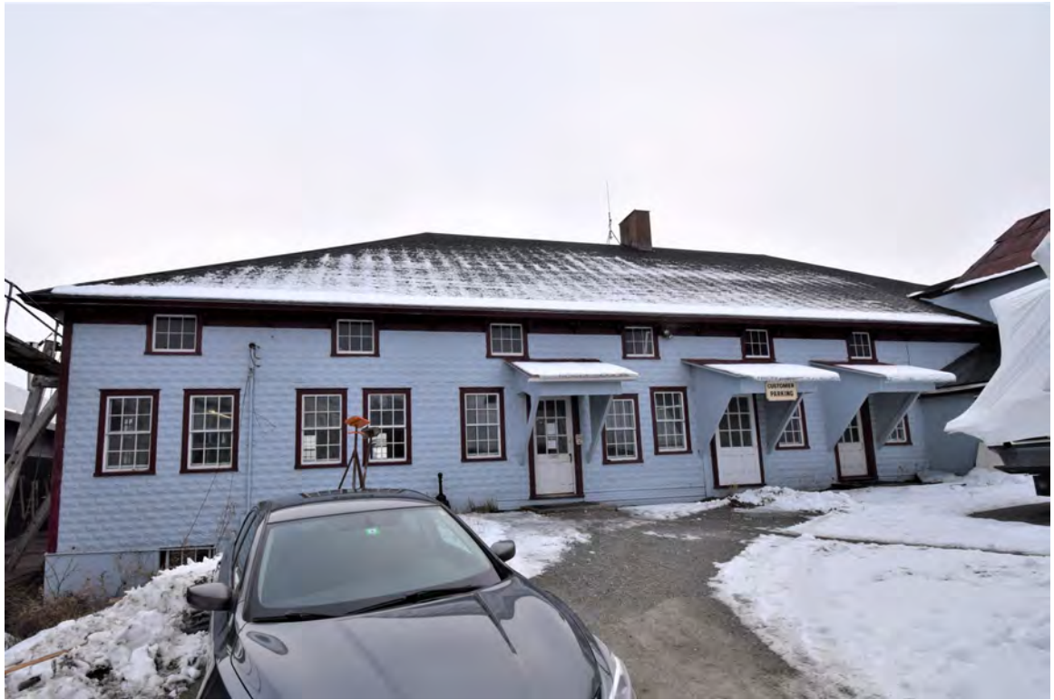
Photo 11: Building #4, view looking southeast
