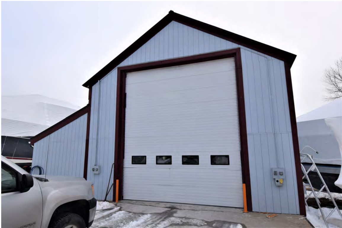
Photo 19: Building #4, view looking southeast, shows entrance to fiberglass shop
