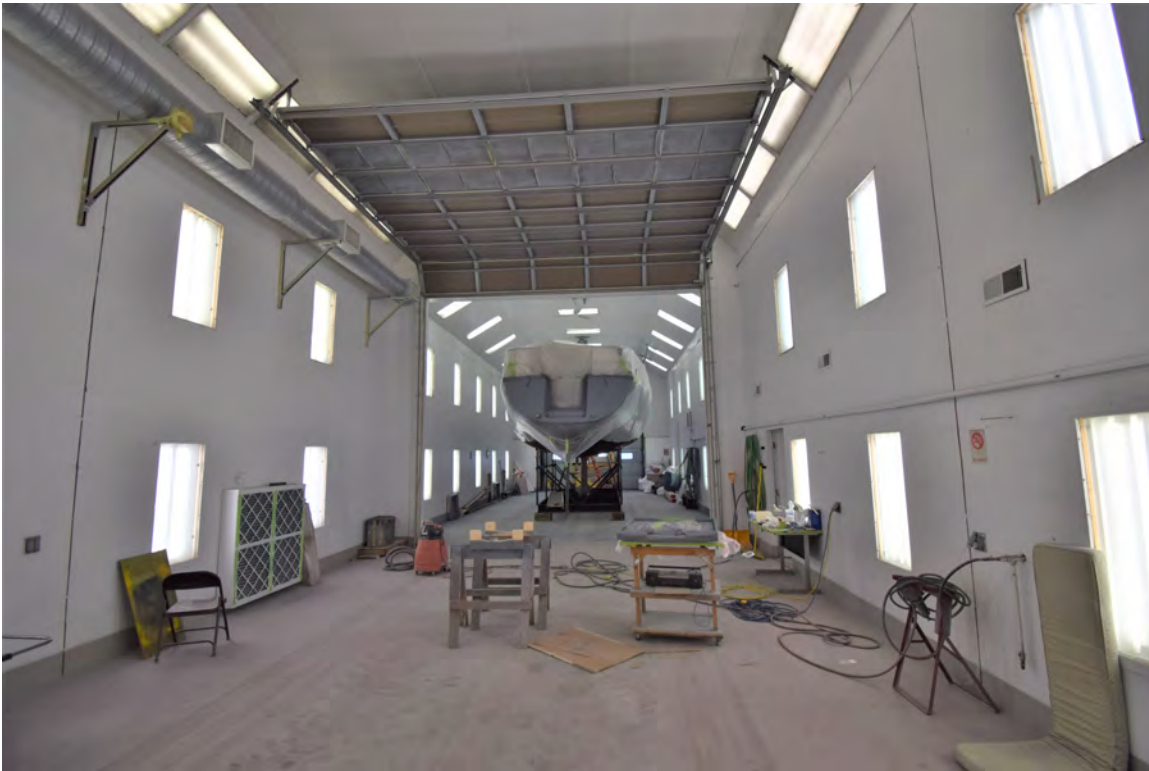
Photo 54: Building #4, view looking northwest in fiberglass shop
