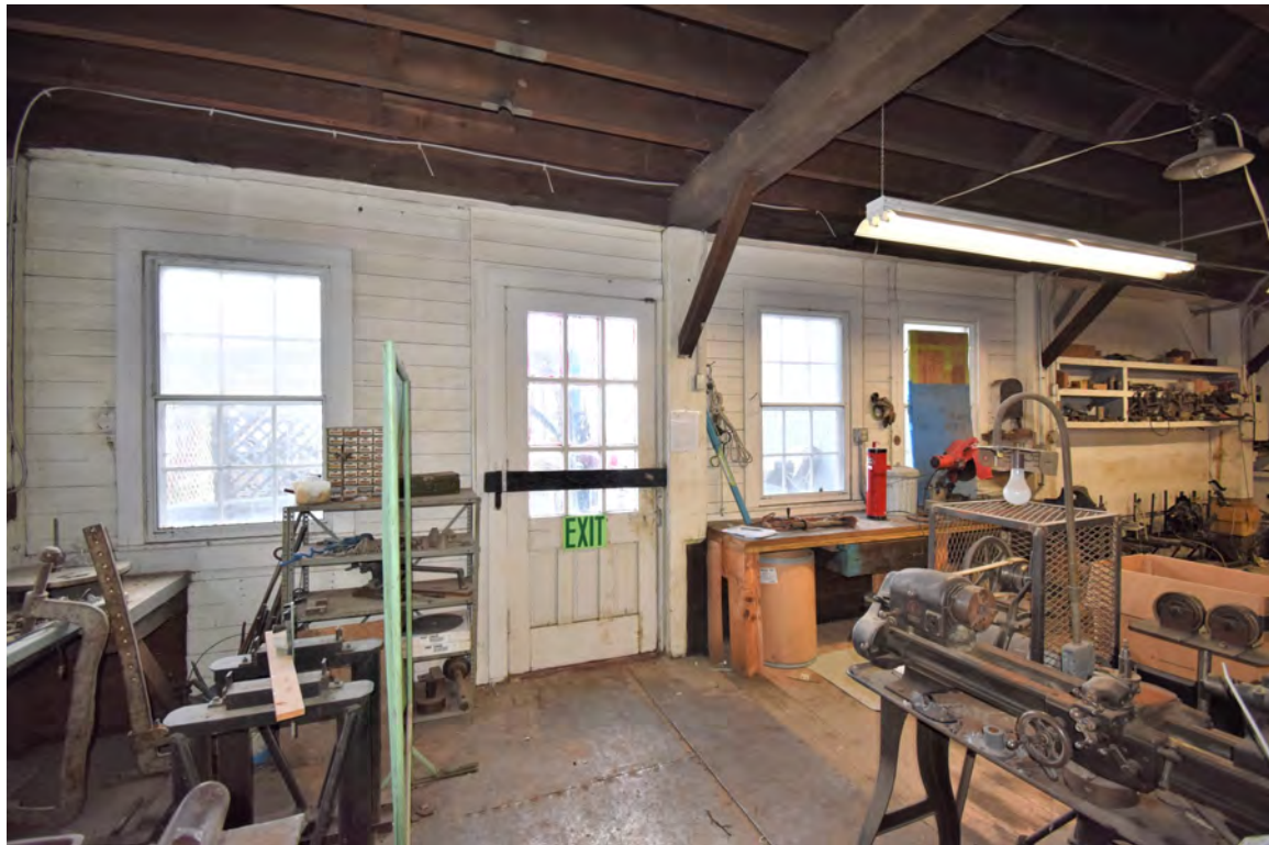
Photo 26: Building #4: view looking south in ground floor, machine shop side. Note original door, and windows with interior storm units.
