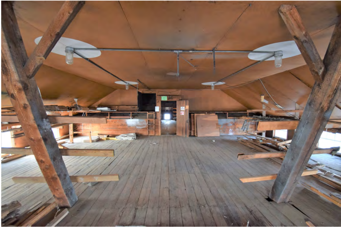
Photo 51: Building #4, view looking northwest in lakeside pavilion 3rd floor
