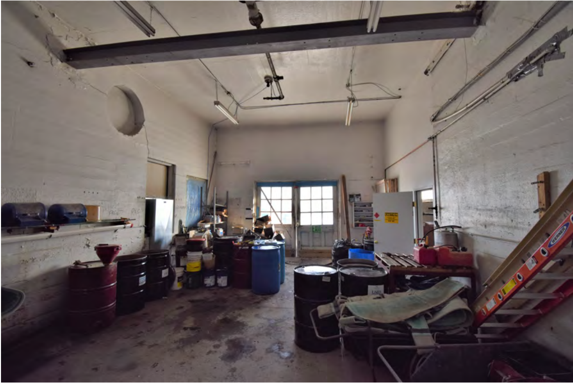
Photo 37: Building #4, view looking southeast in lakeside pavilion room 3 of 3. Note concrete floor, wall and ceiling fireproofing.
