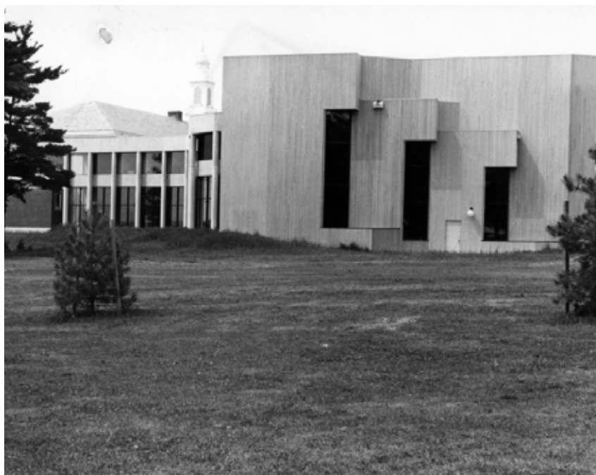
Figure 16: 1975 photograph of the Music Building addition to Southwick Hall (#8). UVM Landscape Change Program file #10382_000.
