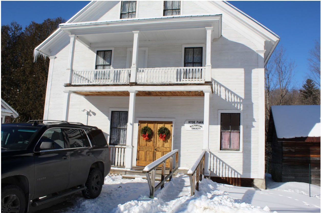
Vermont_LamoilleCounty_GihonValleyGrangeHall_0002: Exterior, detail view of the porch and façade. Camera facing northwest.
