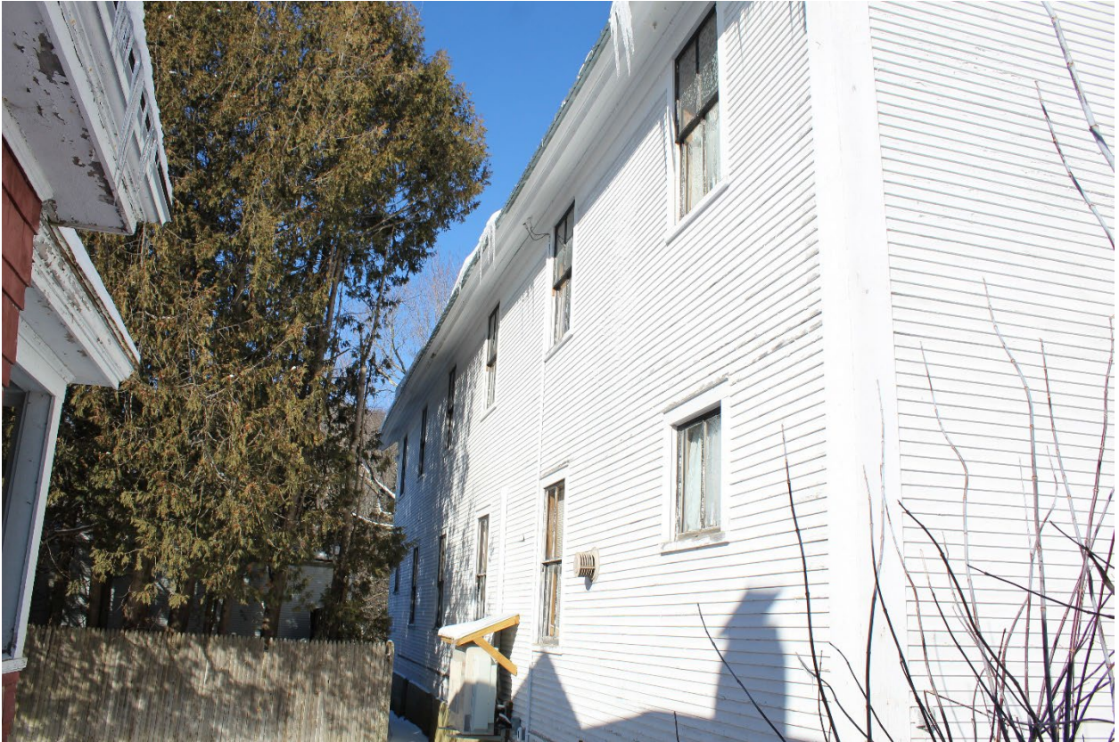
Vermont_LamoilleCounty_GihonValleyGrangeHall_0003: Exterior, southern elevation. Camera facing northwest.
