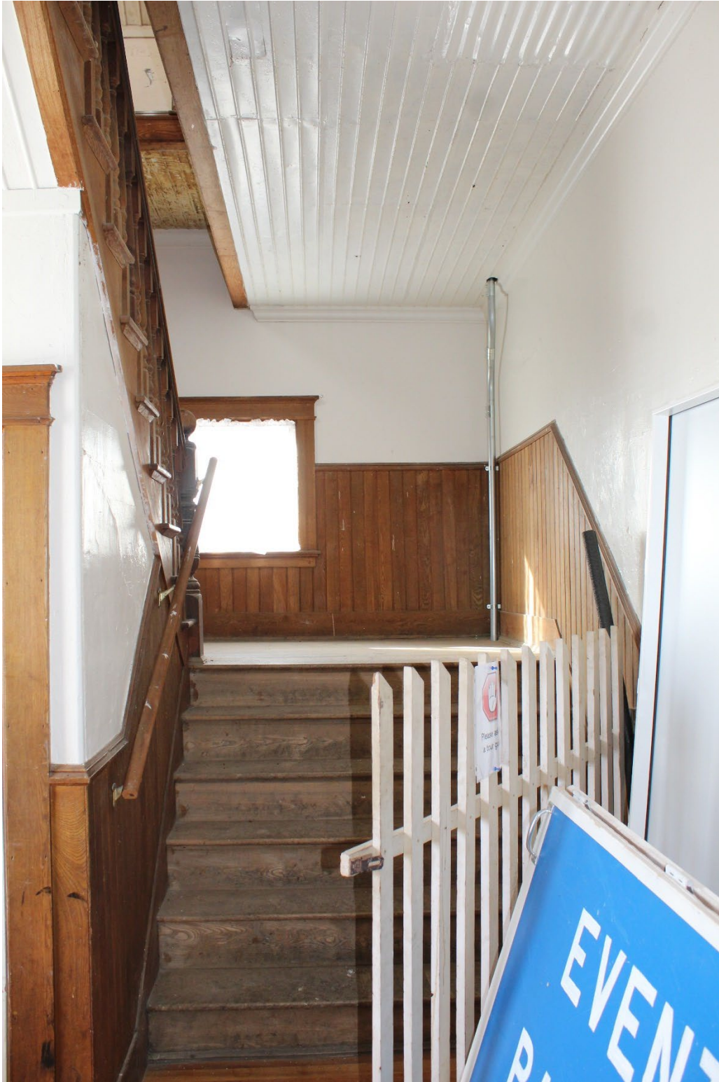
Vermont_LamoilleCounty_GihonValleyGrangeHall_0007: Interior, first floor vestibule showing staircase to the second floor. Camera facing southwest.
