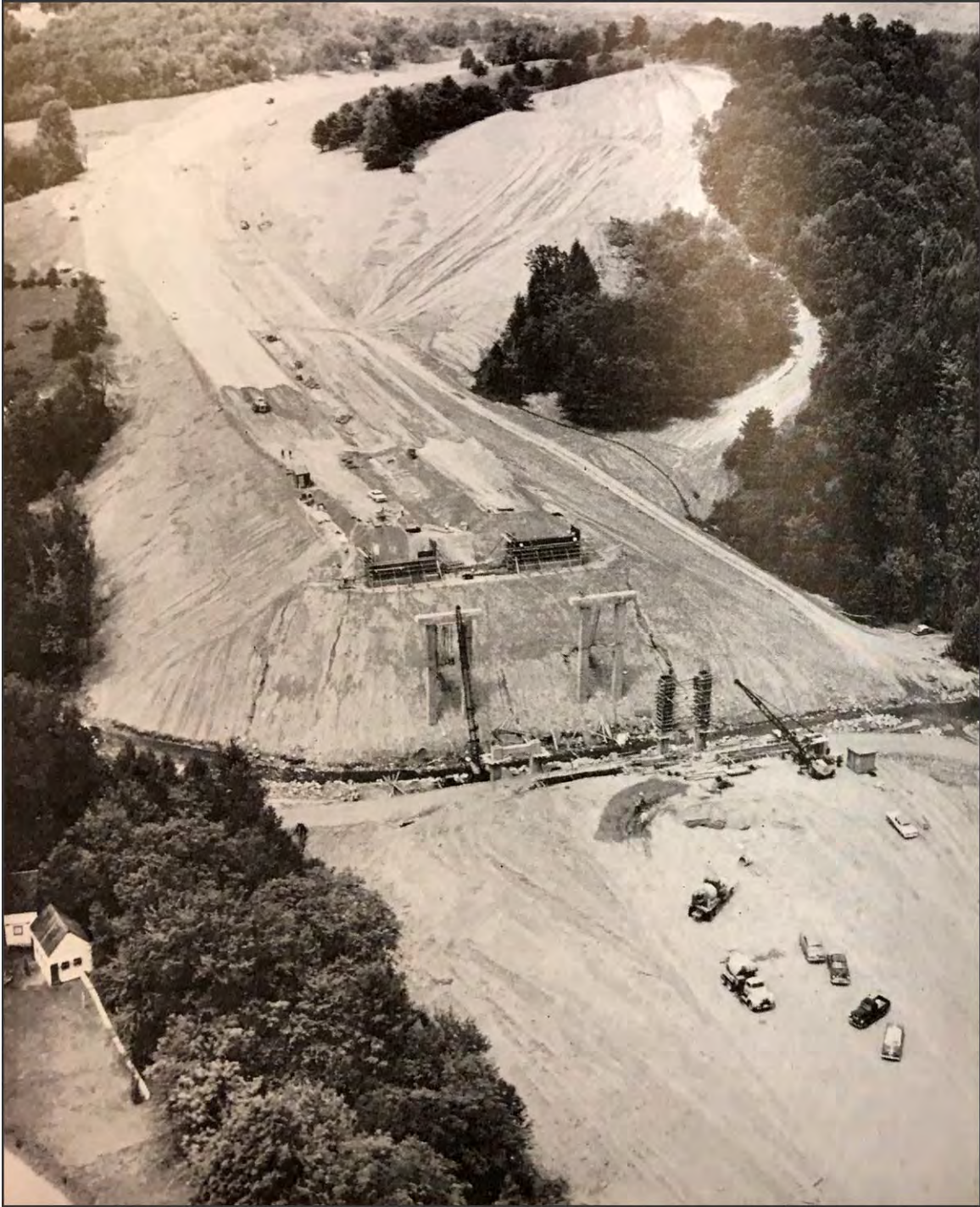
FIGURE 8: Construction of Twin Bridges over Broad Brook on the Brattleboro Bypass (Vermont State Highway Board 1956-1958)
