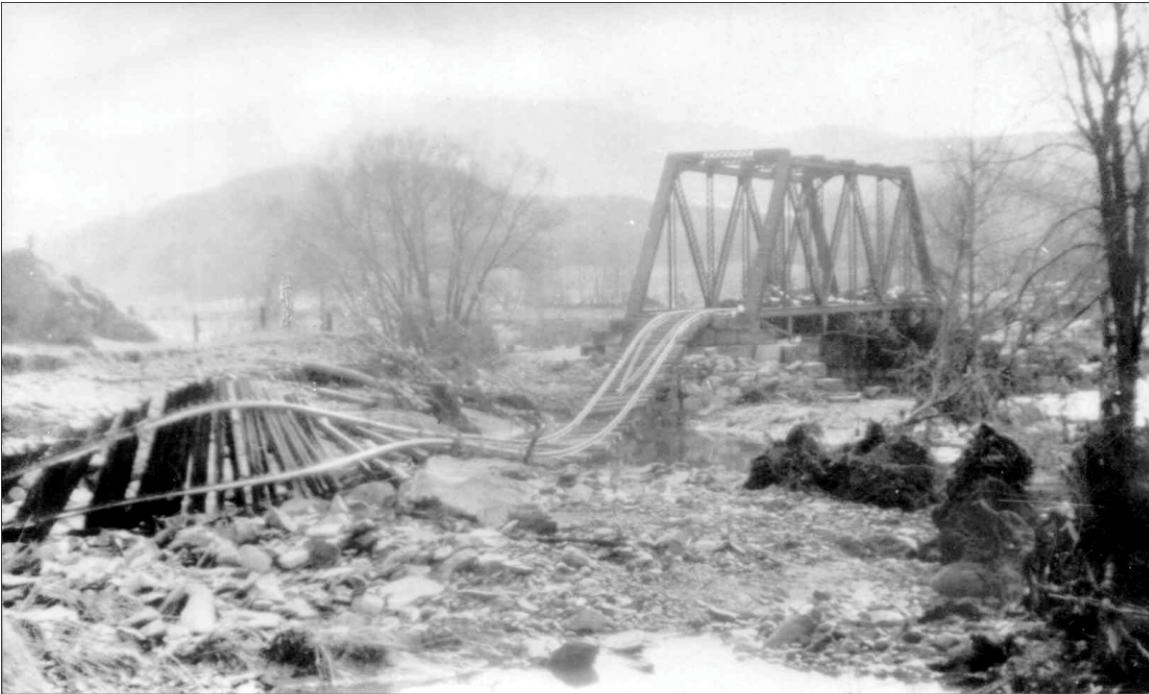
FIGURE 20: Damage to Railroad After Flood of 1927 (Landscape Change Program 2011i)
