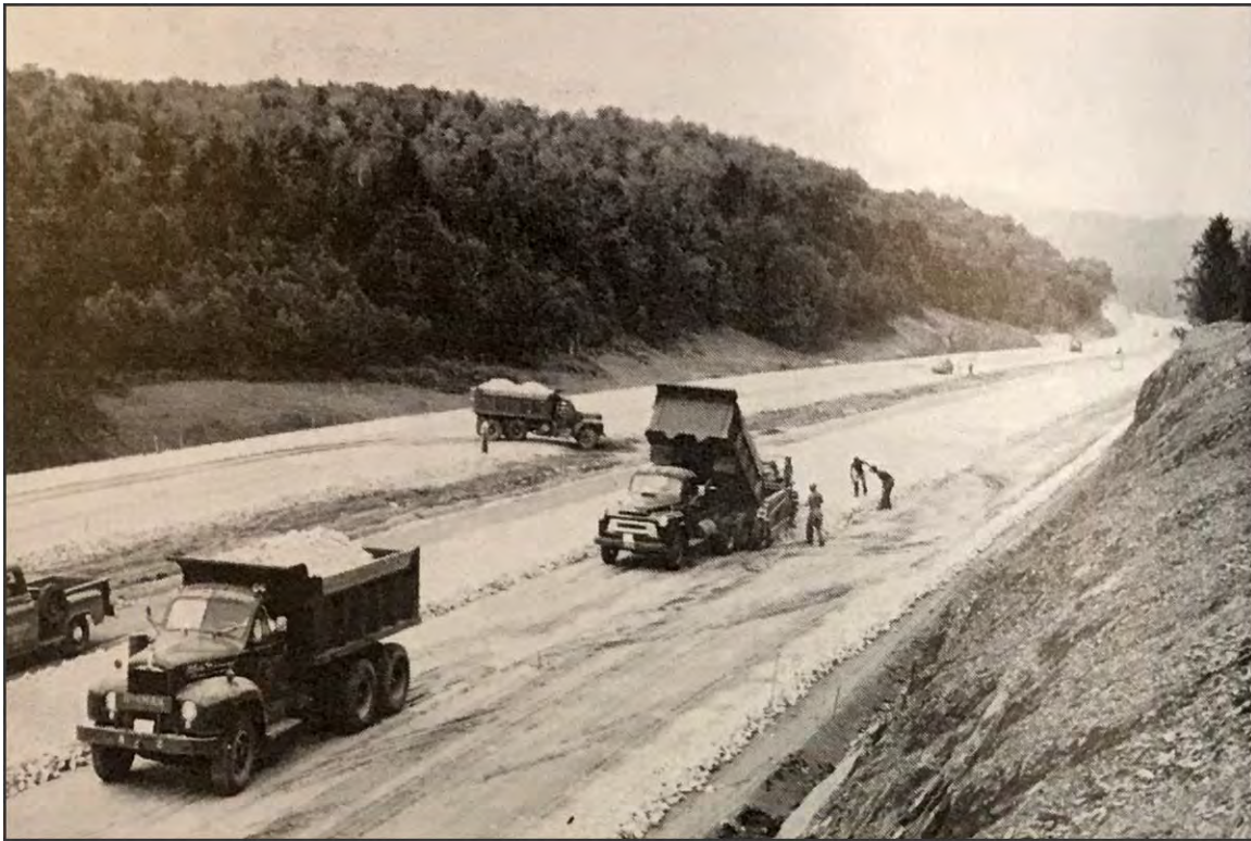
FIGURE 12: Constructing the Base on Vermont's First Interstate Highway Link (Vermont State Highway Board 1956-1958)
