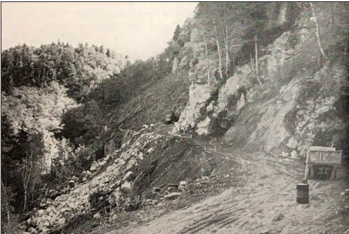
FIGURE 10: Excavation for McCullough Turnpike Connector, 1956 (Vermont State Highway Board 1954-1956)
