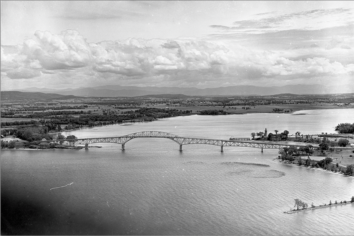
FIGURE 4: Aerial View of Champlain Bridge, 1938 (Landscape Change Program 2011a)
