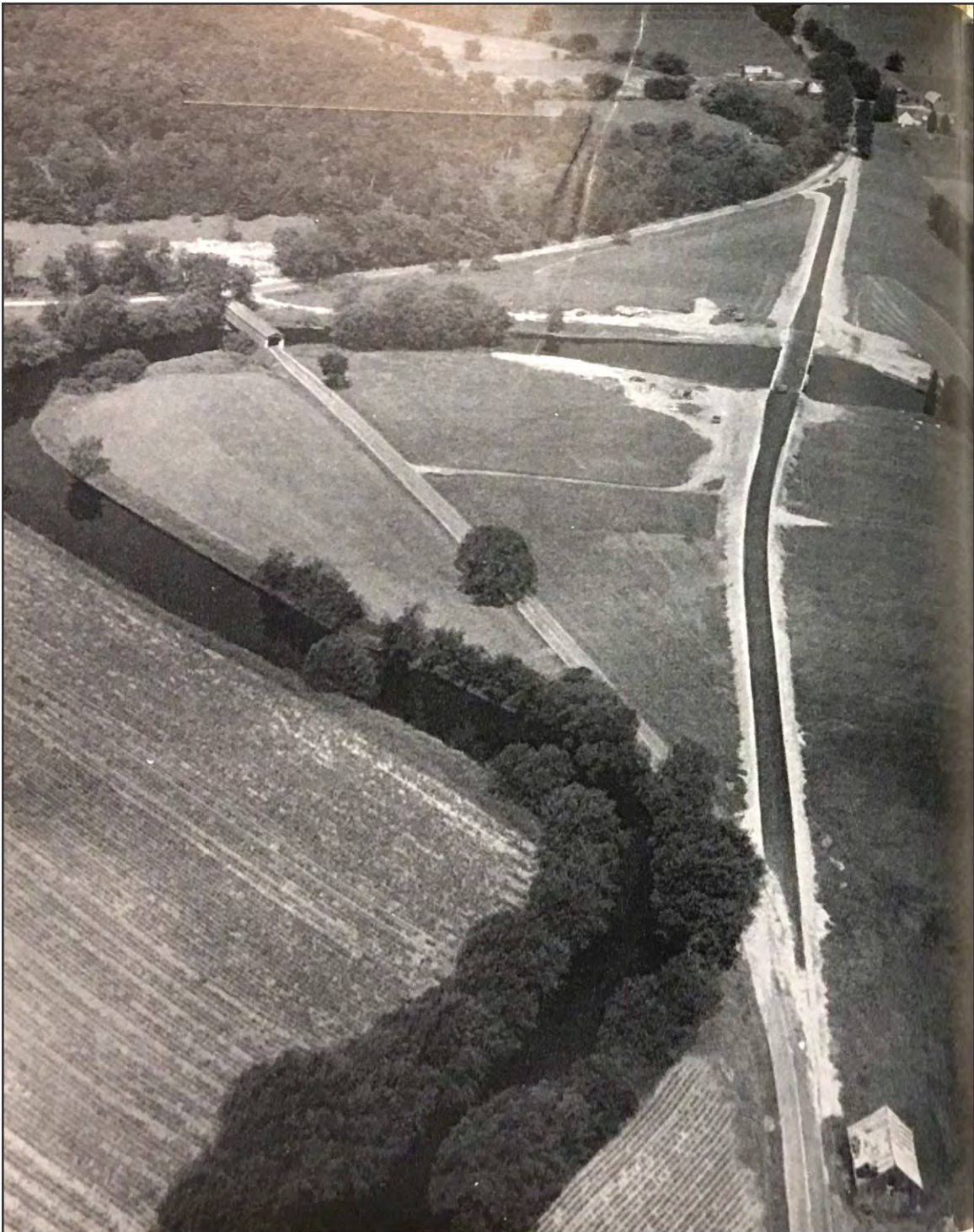
FIGURE 2: New Road Alignment Bypassing the Miller Bridge in Sudbury (Vermont State Highway Board 1950-1952)
