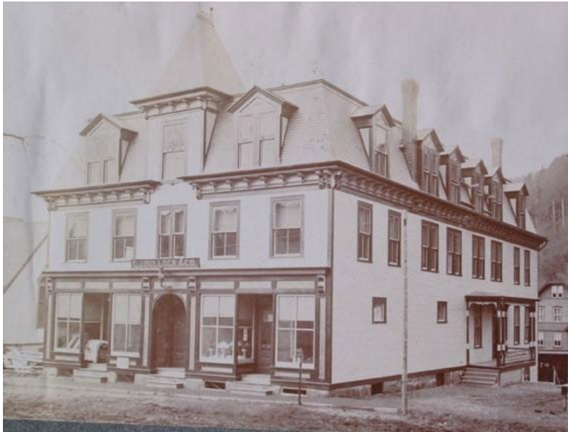
Figure 1: Photograph of the E. J. Bullock Block Circa 1895 showing the building soon after its construction and at a point when the E. J. Bullock & Co. Store occupied the building's first floor. 46
