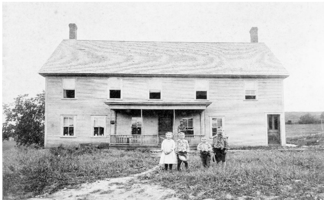
Figure 5 Parsonage (HD #46) (Calais Historic Preservation Commission)
