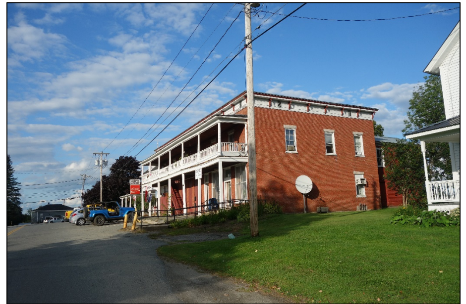
Figure 19: Ray's Market, Post Office, and Apartments Overhead (#34 on map)
