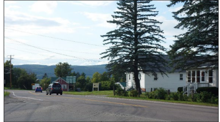
Figure 2: Looking west on Route 58. Masonic Temple (#8 on map) and excavation business (#6 on map) are on right.
