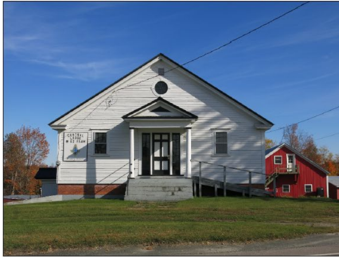
Figure 11: Masonic Temple (#8 on map) Excavation business (#6) in back
