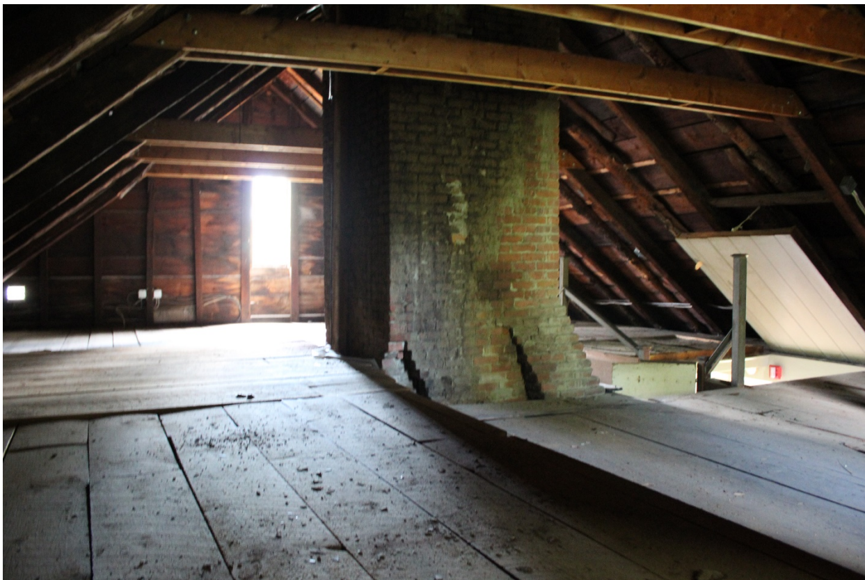
Photo 15: Vermont_Windham_GovernorHuntHouse_0015: Attic level showing massive chimney stack and roof framing in the unfinished space. Camera facing south.
