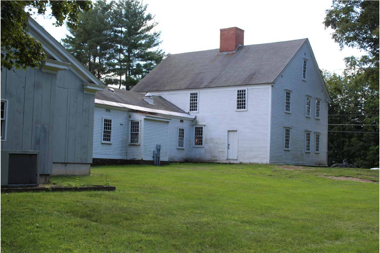
Photo 5: Vermont_Windham_GovernorHuntHouse_0005: Rear and northern elevation of the 1779 building as well as the rear additions. Camera facing southwest.
