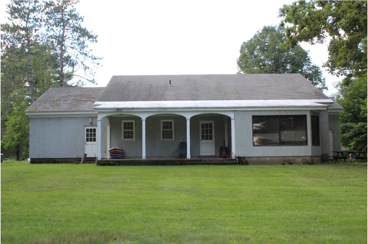
Photo 4: Vermont_Windham_GovernorHuntHouse_0004: Rear of the Vermont Yankee addition. Camera facing west.
