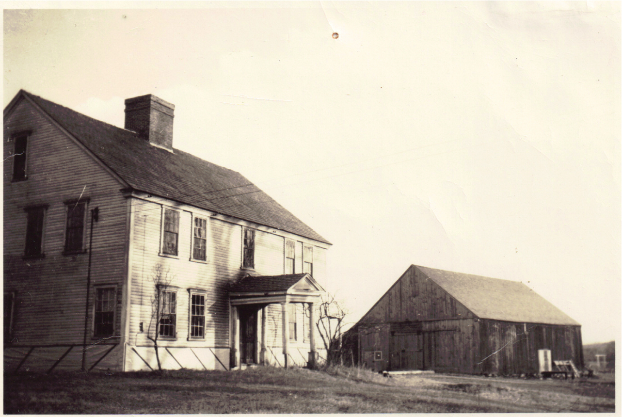
Figure 4: Photo from 1947 showing the Governor Hunt House prior to Florence Louchheim Stol's purchase of the property. Note the presence of 6/6 windows, and a large projecting portico believed to be non-original. Nearby barns have all been subsequently demolished. 43
