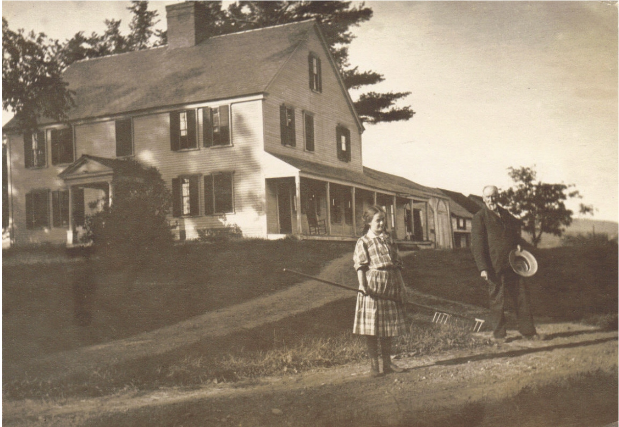
Figure 3: Photo from c. 1905 showing the Governor Hunt House. A full width porch occupies the southern elevation while there are multiple additions telescoping off the main house's rear elevation. 42
