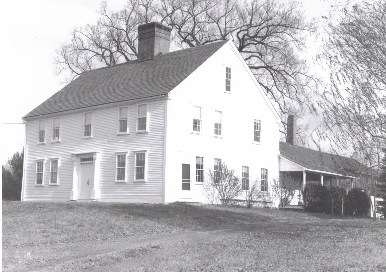
Figure 5: Photo from 1967 just prior to the Governor Hunt House's purchase by Vermont Yankee. The photo shows the entry installed by Florence Louchheim Stol with square pilasters, a secondary entry on the southern elevation, and a side porch/addition off the rear elevation. 44
