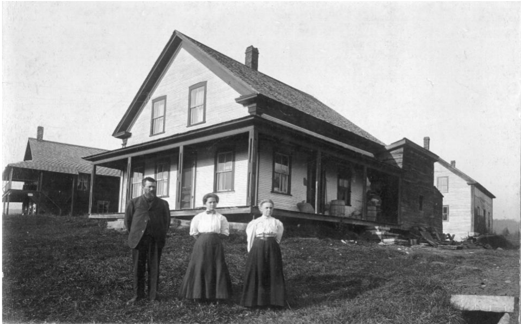
Figure 6 Dailey House (HD #10), c. 1908 (Calais Historic Preservation Commission). Note the former Dailey store to the left and the building that replaced it, to the right.
