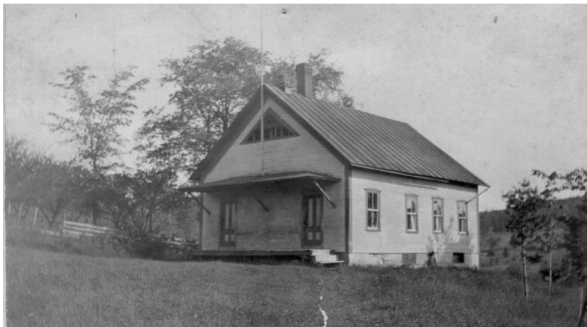
Figure 3 Schoolhouse (Calais Historic Preservation Commission)
