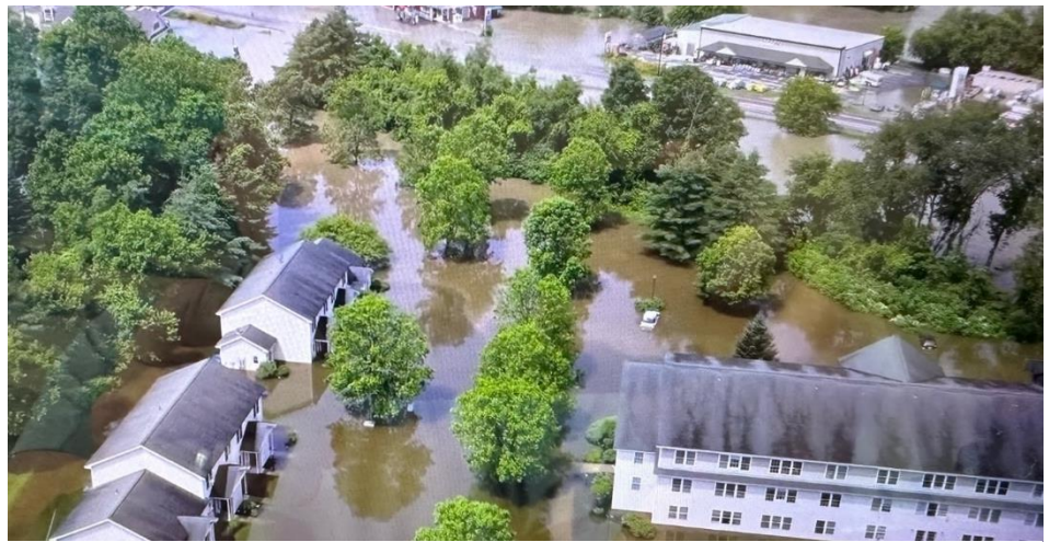
Mann’s Meadow apartments in Jeffersonville after July 2023 flooding.
