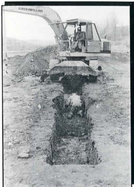
Backhoe digging trench through cellar.
