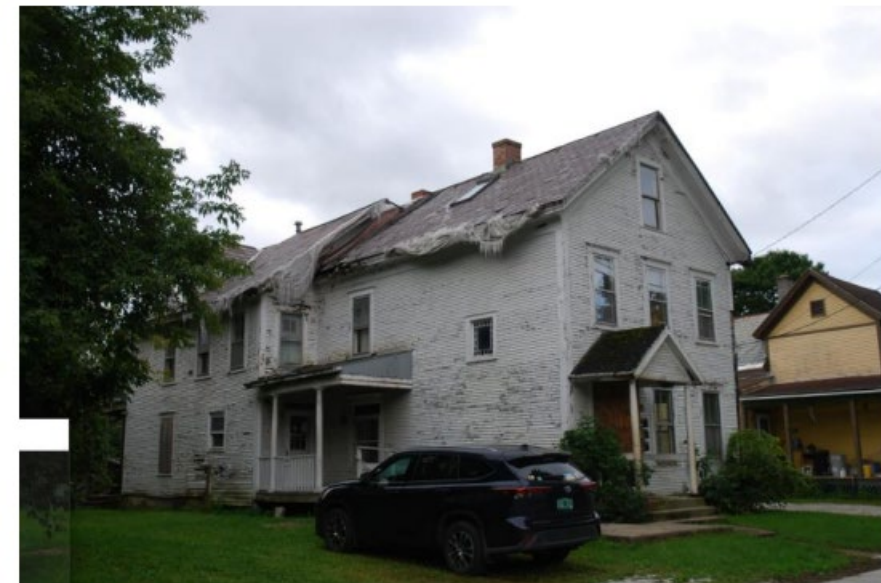
Figure 1 View looking Southwest
