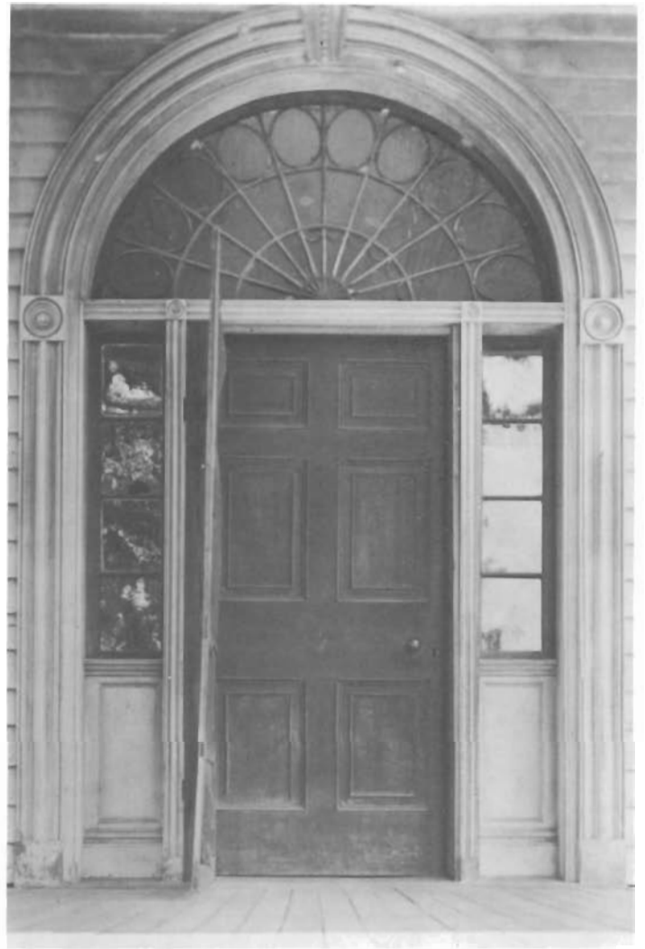
Boykin Hall, Georgia (early 19th century). In addition to providing illumination, the fanlight and side lights are incorporated into an architectural feature that is designed to draw attention to the doorway. Some side lights can be opened for ventilation.
