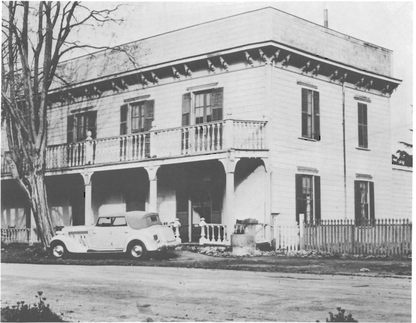
Zanetta House, California (1815). The whitewashed walls reflect the strong California sun. Shutters with movable louvers control the amount of sun passing through the windows. Another feature not readily apparent is that the walls are adobe under the wood sheathing. Adobe has characteristics similar to masonry, thus helping to moderate interior air temperatures.
