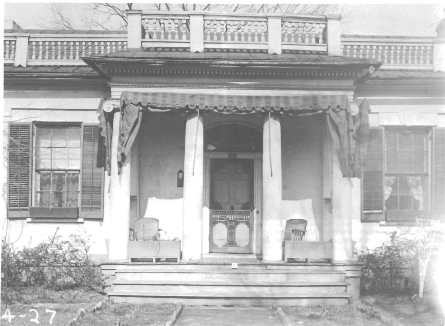
Jerry Cowles House, Georgia (ca. 1830). Awnings can be easily raised or lowered to control the sun. Shutters can be opened and closed to accomplish the same purpose. Although not automated like most of our modern climate controls, shutters and awnings require little effort and can make a substantial difference in interior comfort.
