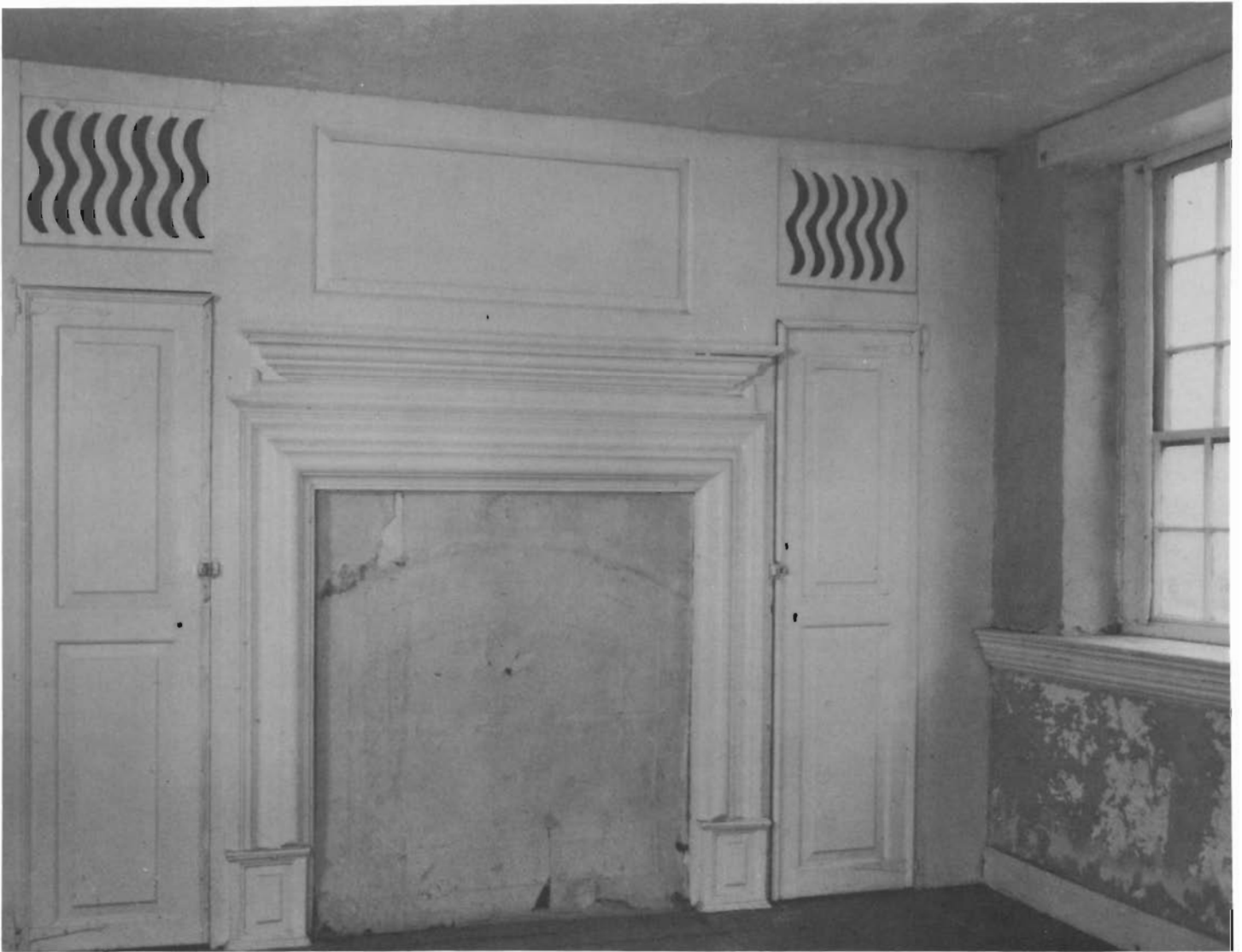
William Miller House (Avondale), Pennsylvania (1730). The closets flanking this fireplace are warmed by the heat from the chimney even though this particular fireplace has been sealed. The warmed air rises, exhausts from the grills over the doors, and is replaced with cool air drawn in the gap under the doors. The grills also provide light to the upper portion of each closet.
