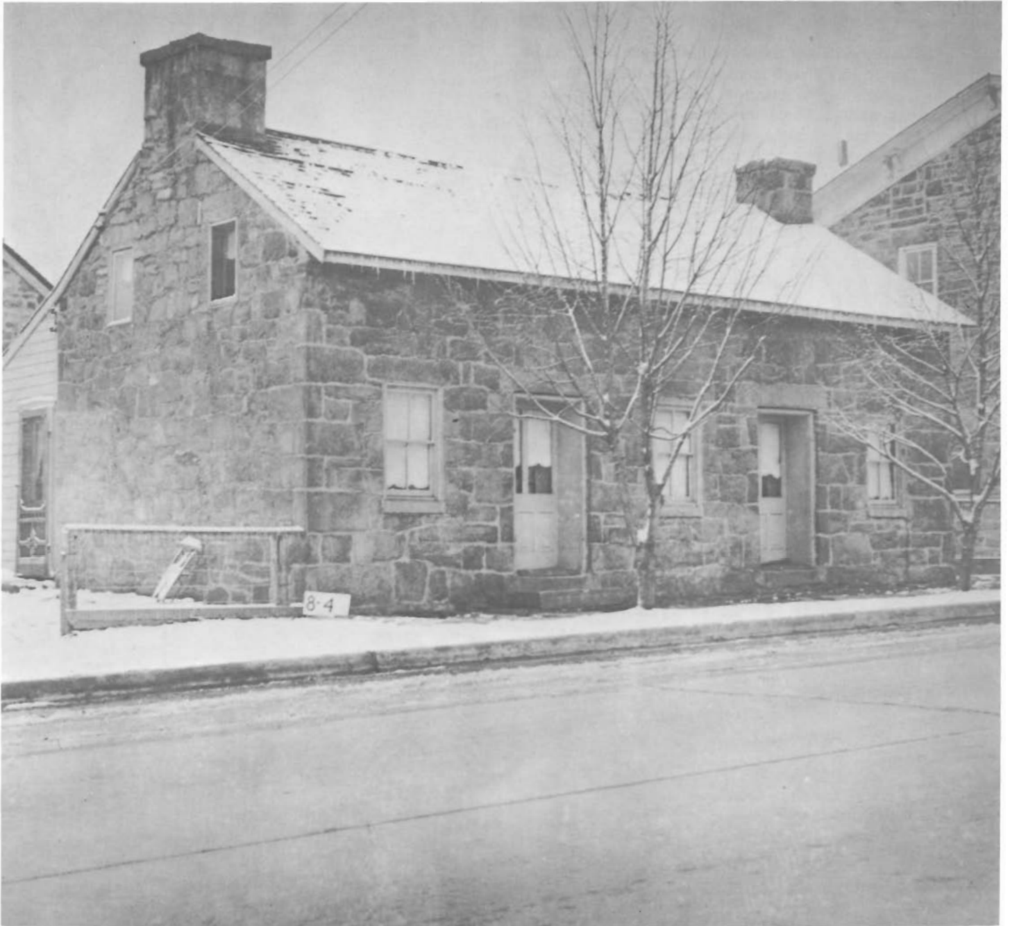
Ben Hayden House, Pennsylvania (ca. 1822). The heavy stone walls, compact shape, and small openings are all energy saving characteristics. Although the individual stones in this house are large, what is important to energy conservation in massive walls is the thickness of the wall, not the size of the masonry units in it.
