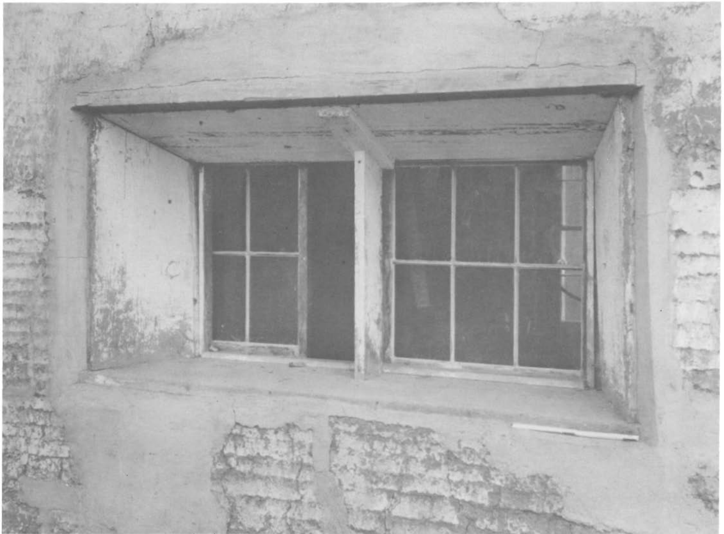
Store, California (ca. 1855). This window has the splayed reveal on the outside, shading the window from direct sun, but allowing in as much incident light as possible. Note that the window head is also splayed. The walls are adobe brick, ideal for moderating the effects of the hot California sun.
