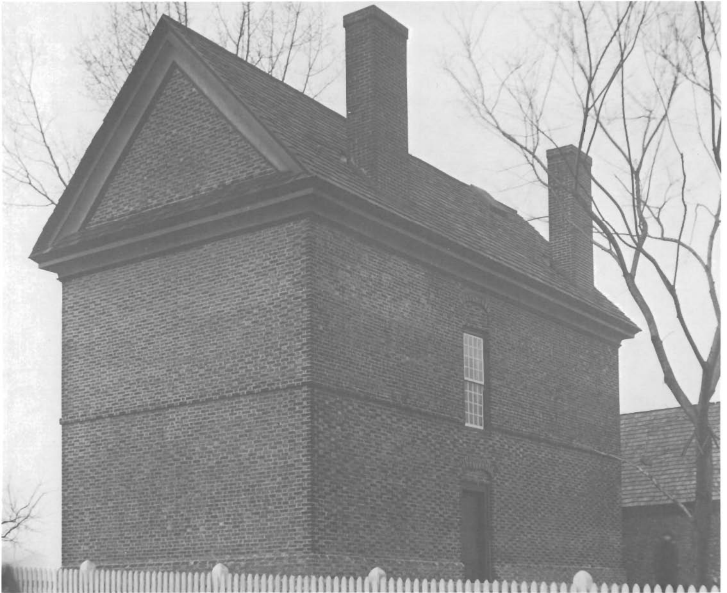
Bel Air (Singly House), Pennsylvania (ca. 1725). The north elevation of this house has no windows except for one which lights the stair landing. There are two interior chimneys in the north wall with fireplaces flanked by closets in each room. The coldest wall in the house is thus isolated from the inhabitants. The closets also serve as warm air convection flues to provide additional heat.
