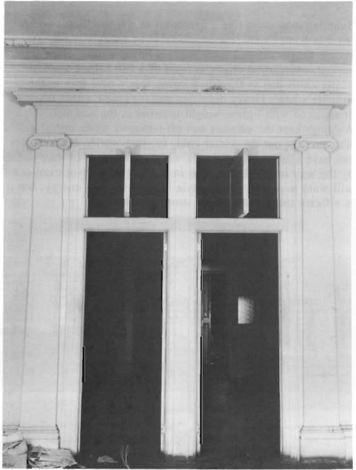
Robert Ralston House, Pennsylvania (early 19th century). These open transoms allow the passage of both light and air even with the doors closed.
