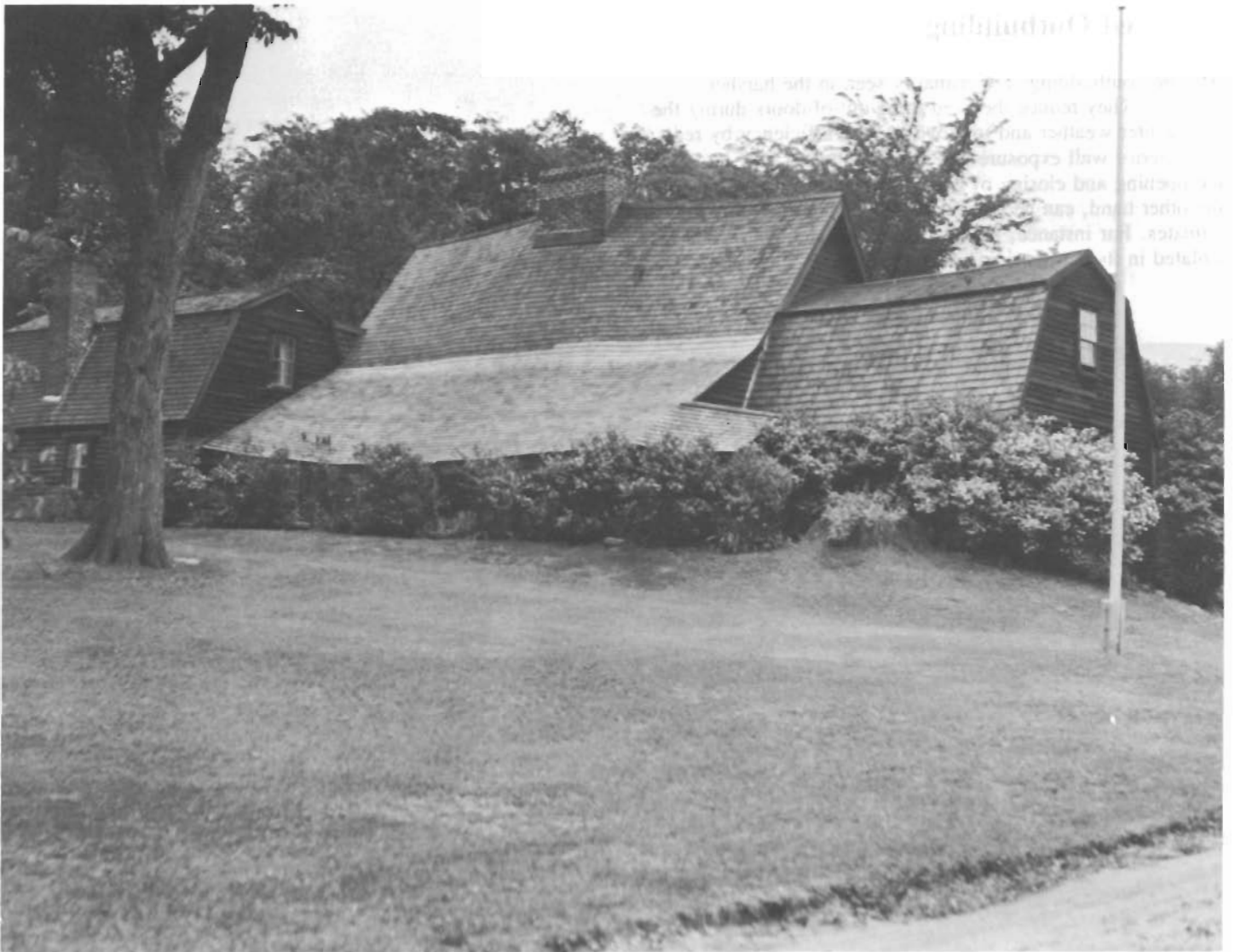
Fairbanks House, Massachusetts (1636). The house is nestled against the southeast slope of a hill with a berm and dense shrubbery protecting the north and west walls from the New England winters. Notice how little of the house other than the roof is visible in this view from the northwest.
