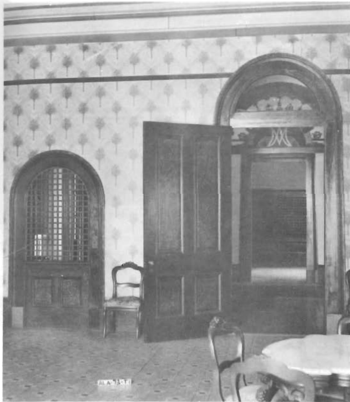
Convent of the Visitation, Alabama (ca. 1864). The door on the right has a glazed, fixed transom lighting the hallway beyond. The gridded but unglazed opening on the left provides both light and cross ventilation.
