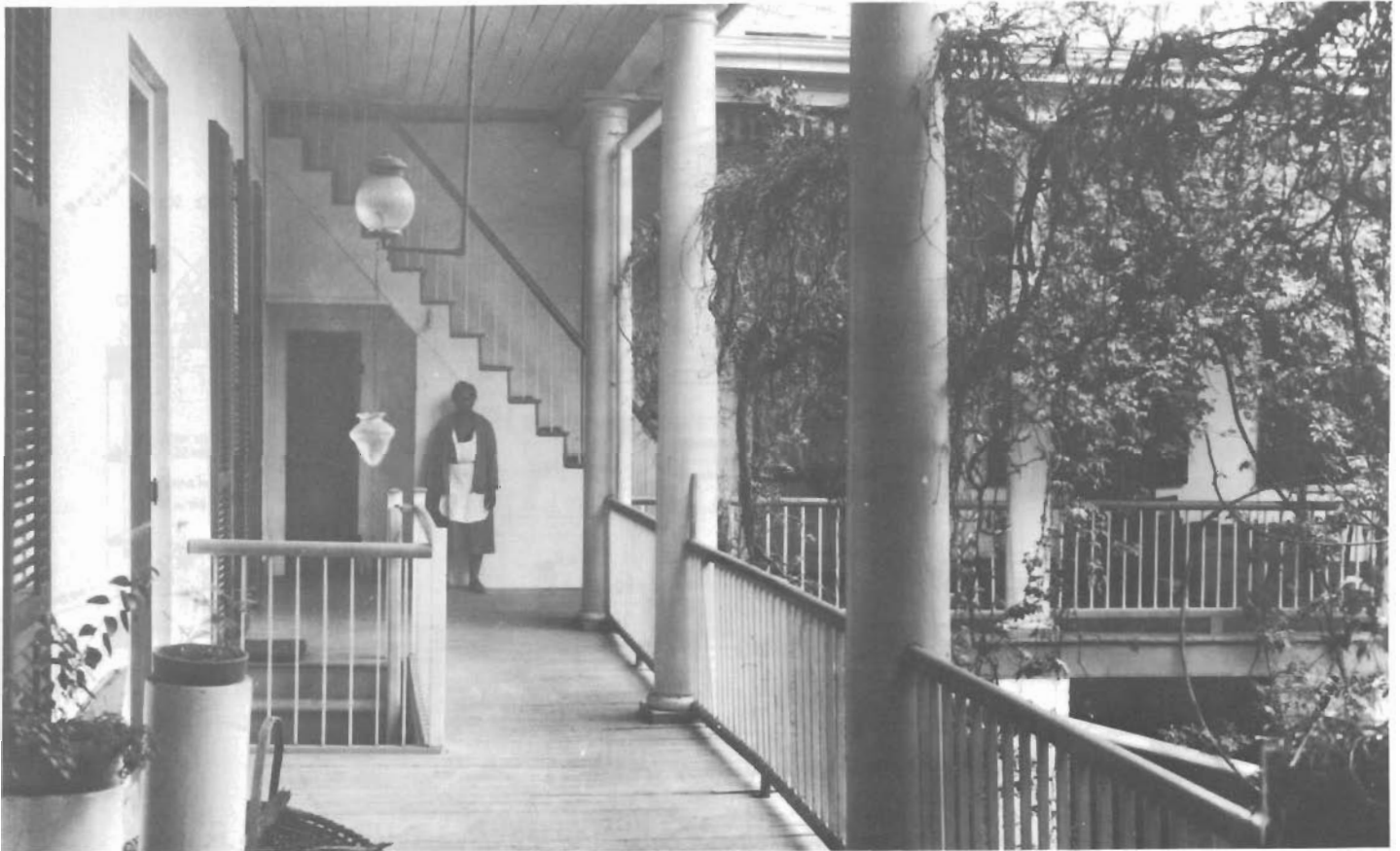
Umbria, Alabama (ca. 1829-30). The two story porch wraps around a courtyard. It not only shades the house but also provides sheltered exterior circulation, appropriate for a warm climate. Shutters with movable louvers and screen doors allow additional control of light and ventilation.
