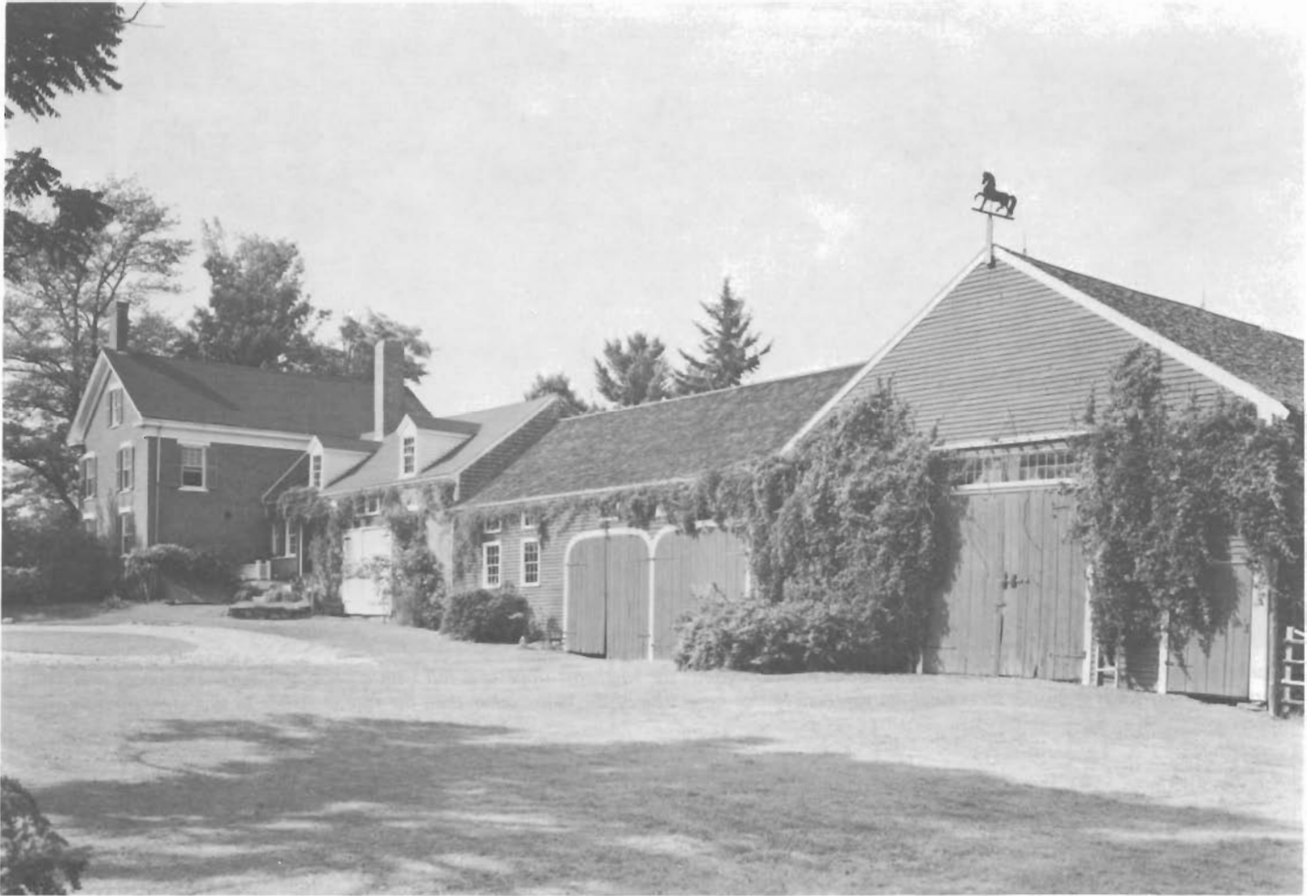
Perkins House, Maine (ca. 1850). Attached outbuildings such as these are common in the cold New England climate. The bulkhead to the cellar of the main house and a porch are nestled in a corner, protected from the wind. Clerestory windows, which bring additional light to the interior, are visible just below the eaves of the two middle sections.
