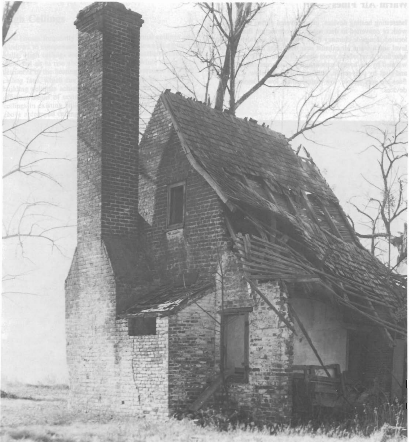
Towles House, Virginia (early 18th century). The chimney placement minimizes the transfer of heat to the interior of the house by reducing the contact area of the chimney mass with the house. The flue is freestanding, reducing not only the heat gain, but the fire hazard as well. The house is no longer standing.
