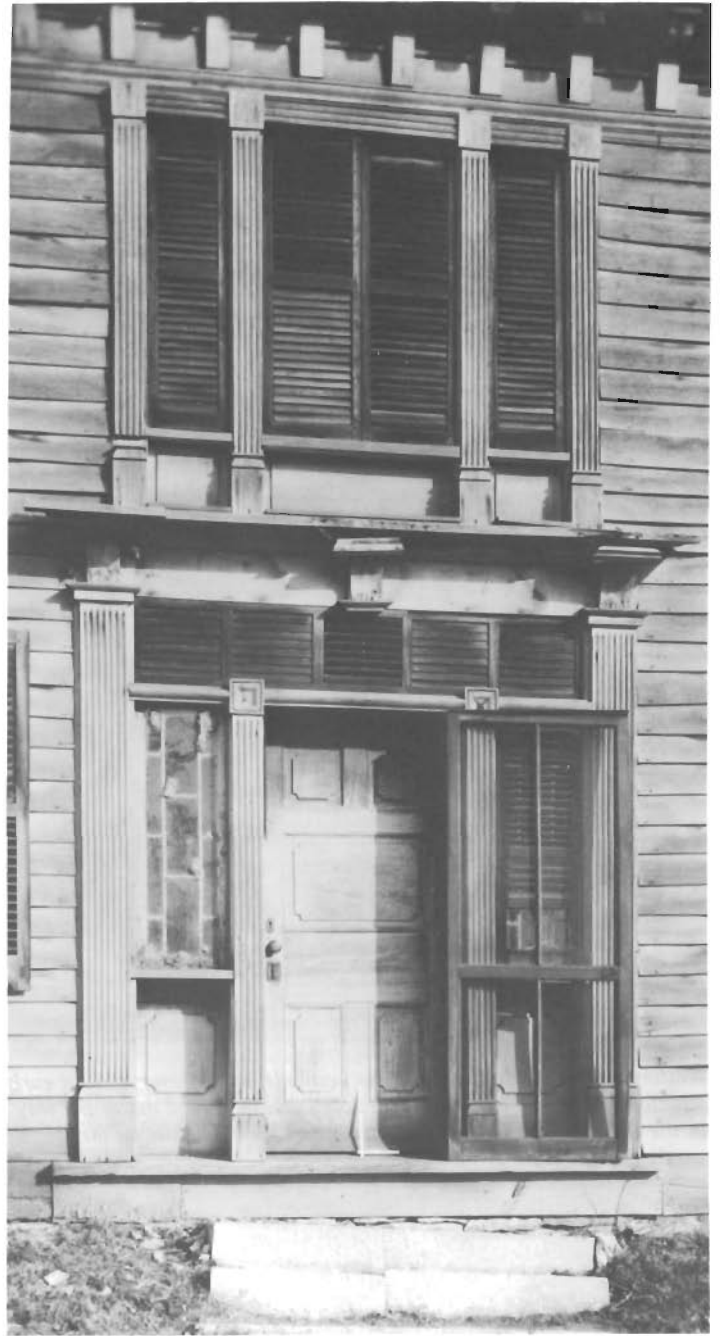
Hancock House, Iowa (ca. 1850). Demountable louvered shutters are used on this entrance and window, where hinged shutters would tend to obliterate the architectural detailing when open. Since they were less convenient to use, they were probably changed seasonally rather than daily.
