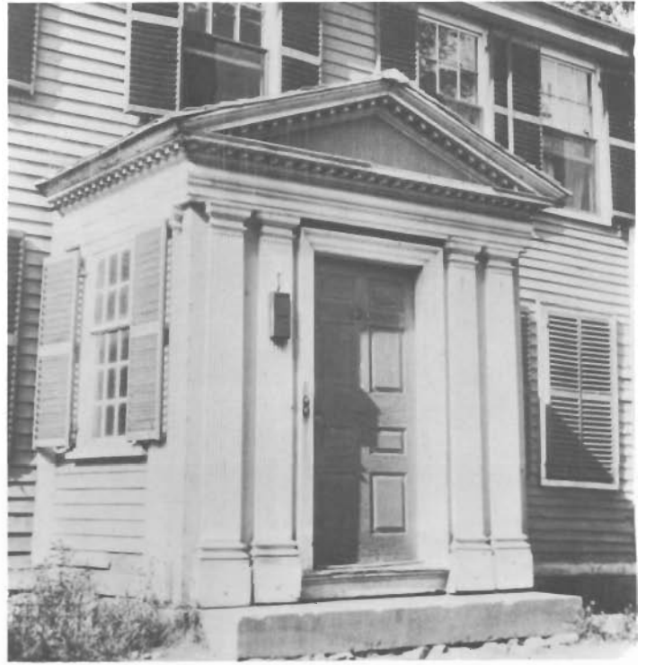
John Bemis House, Massachusetts (ca. 1740). This is an unusually large and elaborate vestibule complete with shuttered windows. Vestibules are generally unheated spaces not requiring this heavy construction.
