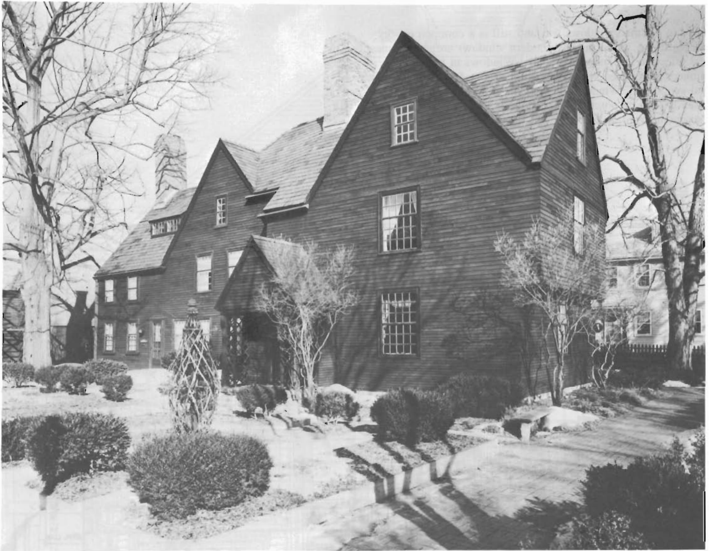
House of the Seven Gables, Massachusetts (ca. 1668). The slate roof and the dark stain on the clapboards are used to help absorb heat from the sun. The deciduous trees shade the house from the sun in the summer so the dark color is not a detriment.
